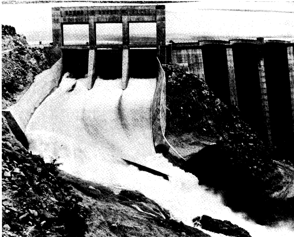
Figure 25.—Prototype spillway discharge; Gate No. 1, 159 \text{ m}^3/\text{s} ( 5600 \text{ ft}^3/\text{s} ); Gate Nos. 2 and 3, 54 \text{ m}^3/\text{s} ( 1900 \text{ ft}^3/\text{s} ). Photo P801-D-79510
