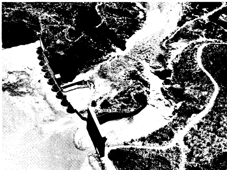
Figure 2.—Aerial view of Bartlett Dam after March 1978 flood (note large eroded hole downstream from spillway chute). Photo P801-D-79494
