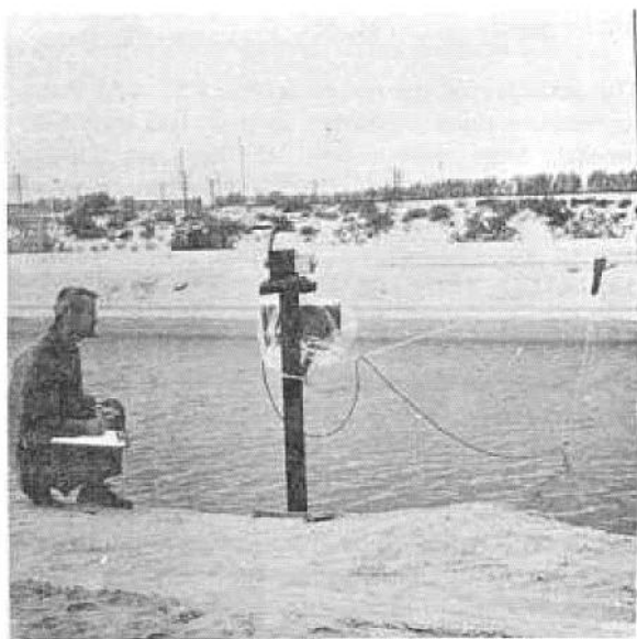
Figure 50. Radioisotope detector and counter installed for canal discharge measurement. Photo P50-D-31943
