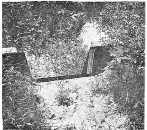
Figure 14. Sediment deposits have reduced the depth of the weir pool sufficiently to increase the velocity of approach to well above the desirable level. The head gage should not be located close to the weir blade. The weeds should be removed and the "edge" of the weir should be sharp. Discharges over this weir will be larger than indicated in "standard" tables. Photo P20-D-21558
