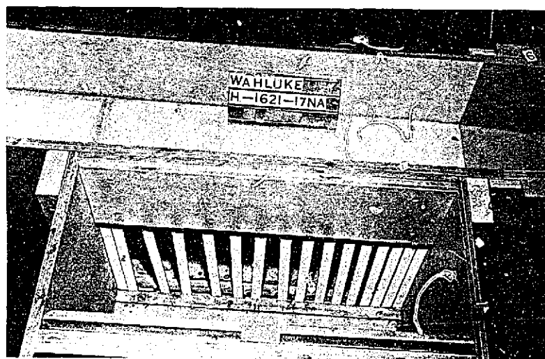
Baffled turnout looking upstream. Photo P222-D-67493
