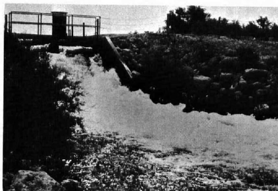
E. Baffled drop at MODE 2. Photo PX-D-66014
