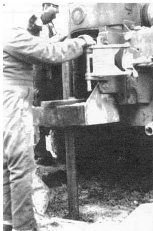
Figure 10. – Closeup of Failing 1500S drill rig during push-tube sampling. P-801-D-81152
