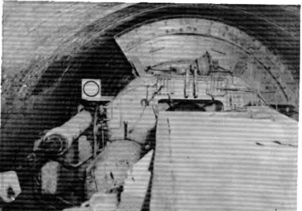
MACHINE AT HEADING. NOTE LASER BEAM TARGET
