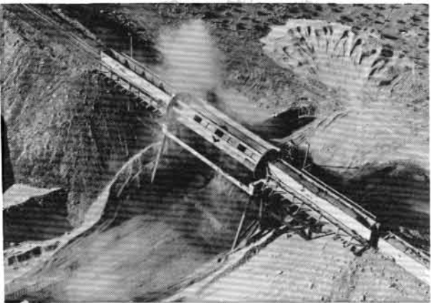
WASTE DISPOSAL-ROTARY CAR DUMP IN OPERATION
