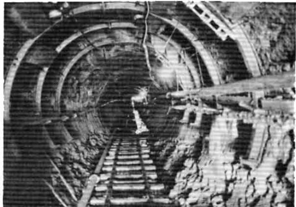
SANDSTONE & SHALE SECTION. THE SHALE DETERIORATES RAPIDLY
