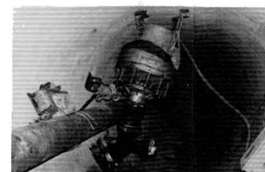
88 HP PUMP INSTALLED TO PUMP WATER FROM SPRING IN THE INVERT TO THE INLET OF HADES TUNNEL
