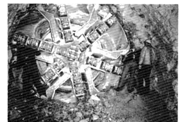
CUTTER HEAD AT HOLE THROUGH
