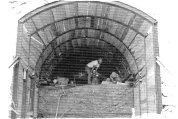
TURNING UNDER AT INLET PORTAL
