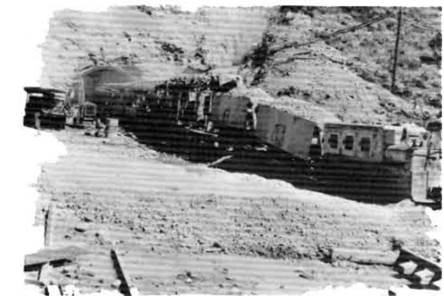
LOADING MUCK CARS AT START OF MACHINE OPERATIONS
