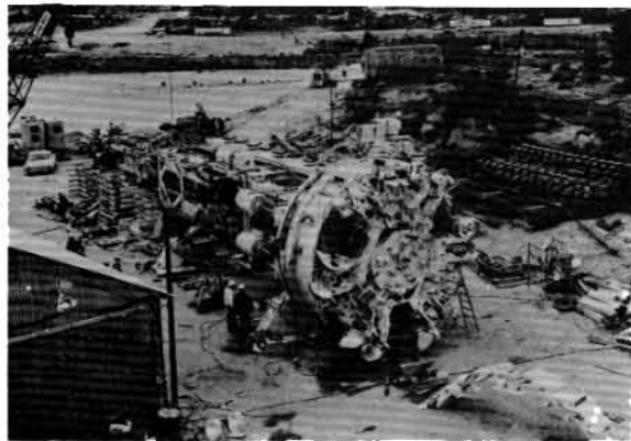
ASSEMBLING MACHINE NEAR TUNNEL PORTAL
