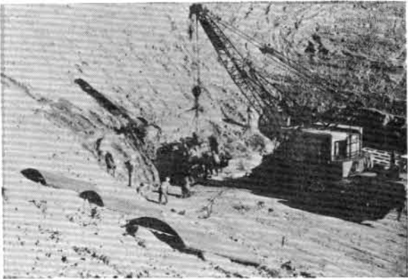
LOWERING CUTTER HEAD INTO GAP TO INSTALL ON MACHINE BODY WHICH WAS MOVED IN THROUGH THE CUT AND COVER
