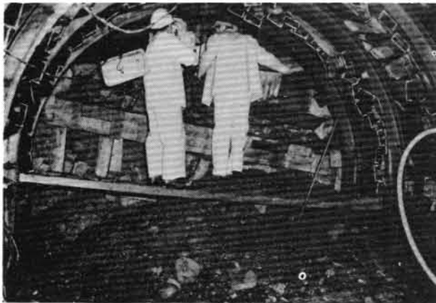
NOTE CHANNEL SPILING AND BREAST BOARDS REQUIRED IN UNSTABLE MATERIAL
