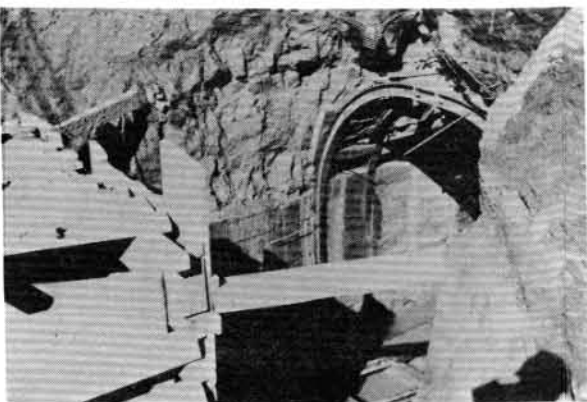
GAP IN CUT AND COVER SECTION AT PORTAL FOR INSTALLATION OF MACHINE CUTTER HEAD
