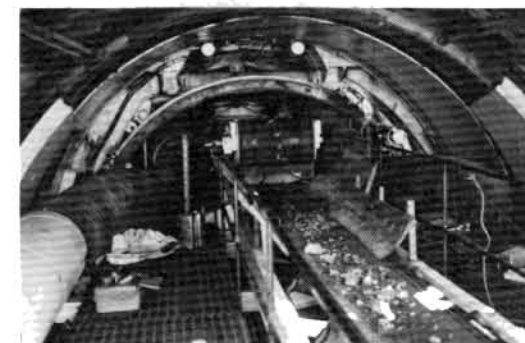
MUCK CONVEYOR AND SEGMENTS BEING INSTALLED
