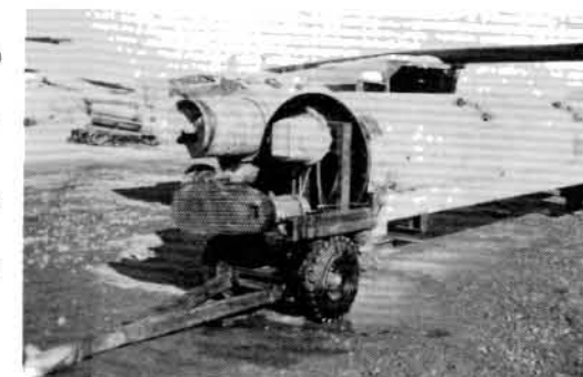
MORAN CAR READY TO HAUL CEMENT TO TUNNEL FOR BACKFILL GROUTING
