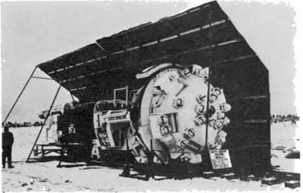
ASSEMBLING BORING MACHINE
