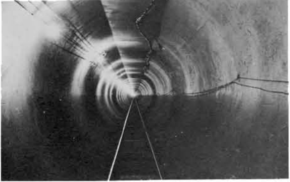
COMPLETED CONCRETE LINED SECTION
