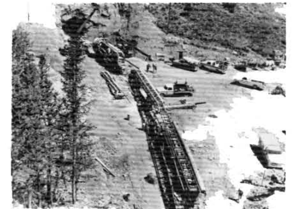
OVERHAULING TUNNELING MACHINE AND BACKUP EQUIPMENT AT OUTLET PORTAL
