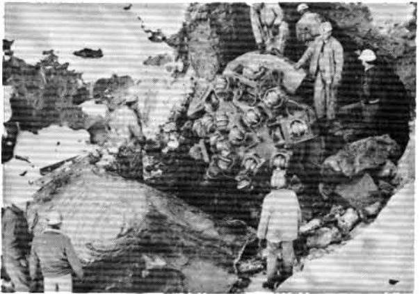
MACHINE HOLED THROUGH AT INLET PORTAL
