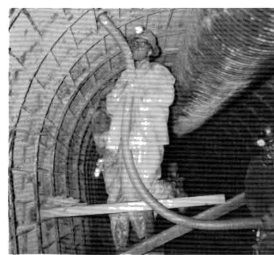
PLACING PEA GRAVEL BEHIND STEEL PLATE LINERS USING THE SHOTCRETE MACHINE
