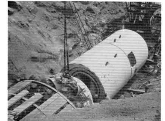
CUTTER HEAD BEING MOVED INTO POSITION FOR ASSEMBLY
