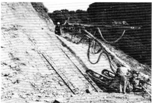
INSTALLING ROCK REINFORCEMENT BARS AT OUTLET PORTAL PRIOR TO HOLING THROUGH
