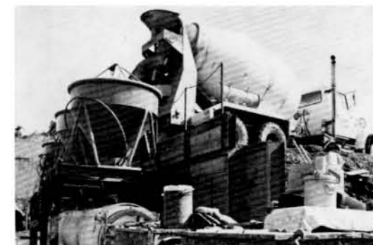
LOADING CONCRETE IN HOPPERS FOR TUNNEL
