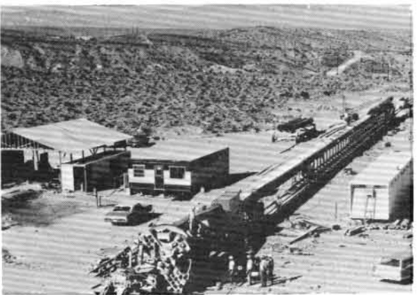
ASSEMBLING MACHINE-NOTE CONVEYOR WITH VENTILATION SYSTEM ON TOP
