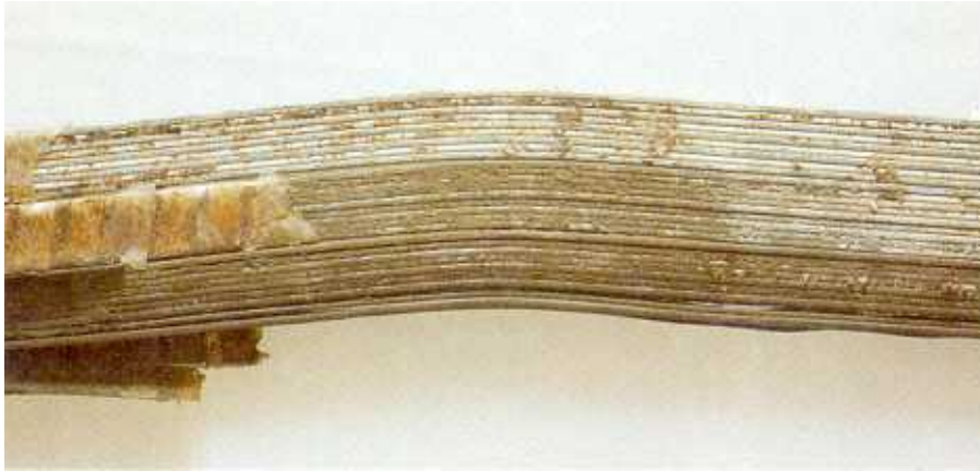
Figure 11.—Groundwall and turn insulation removed from coil. P801-D-79798.
