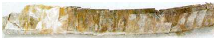
Figure 10.—View showing discoloration of binder material. P801-D-79797.
