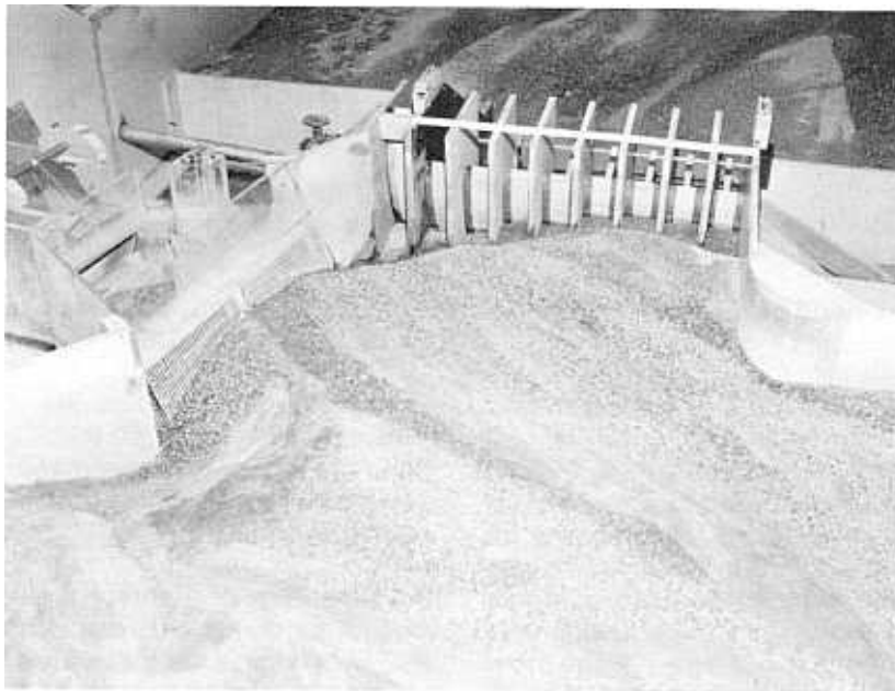
Figure 29.—Narrow spillway gates in conjunction with the existing headworks. P801-D-79637
