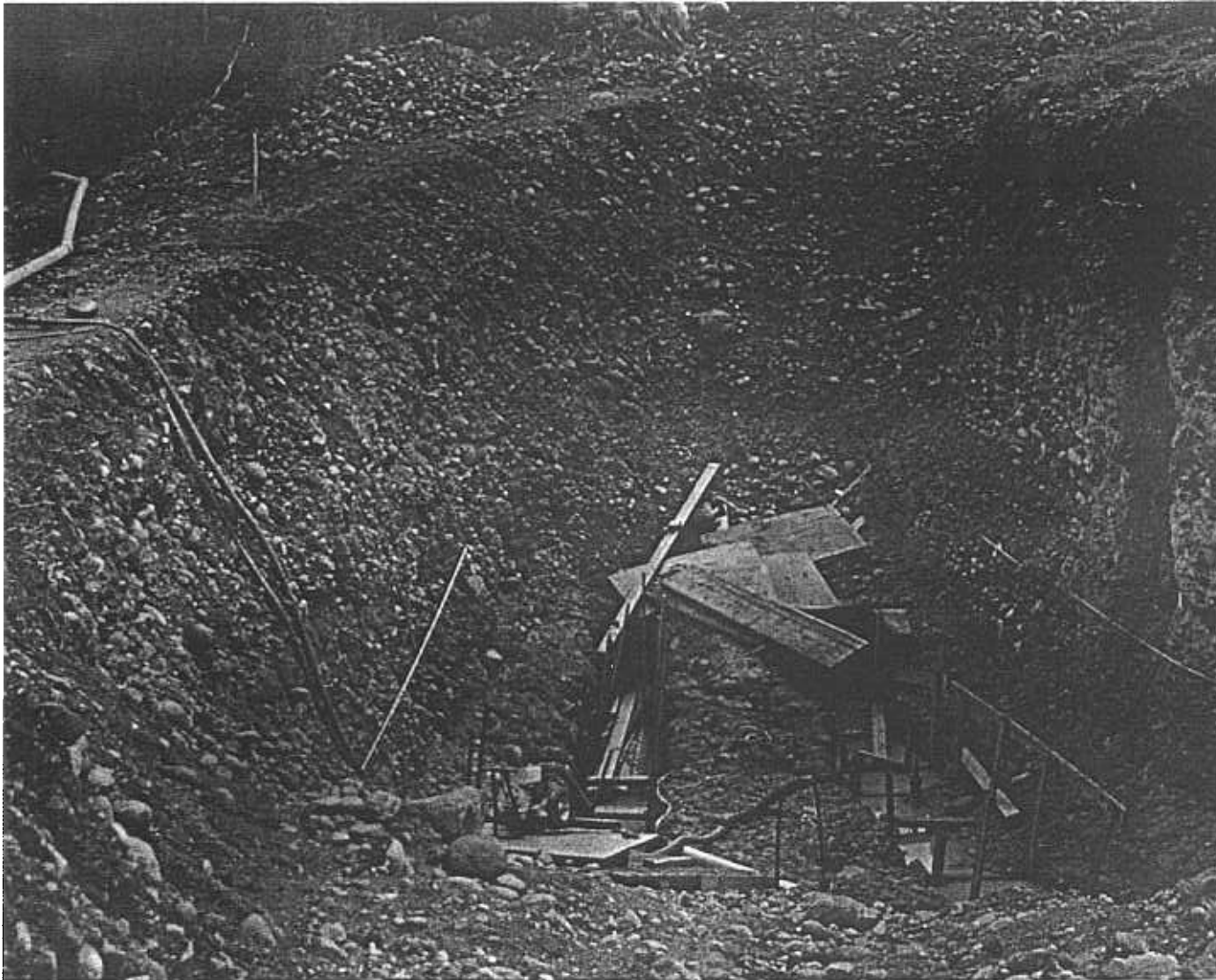
Figure 1.— General view of site ST-68. The eroded shear zone is apparent on the right, or south, wall. Photo P801-D-79248
