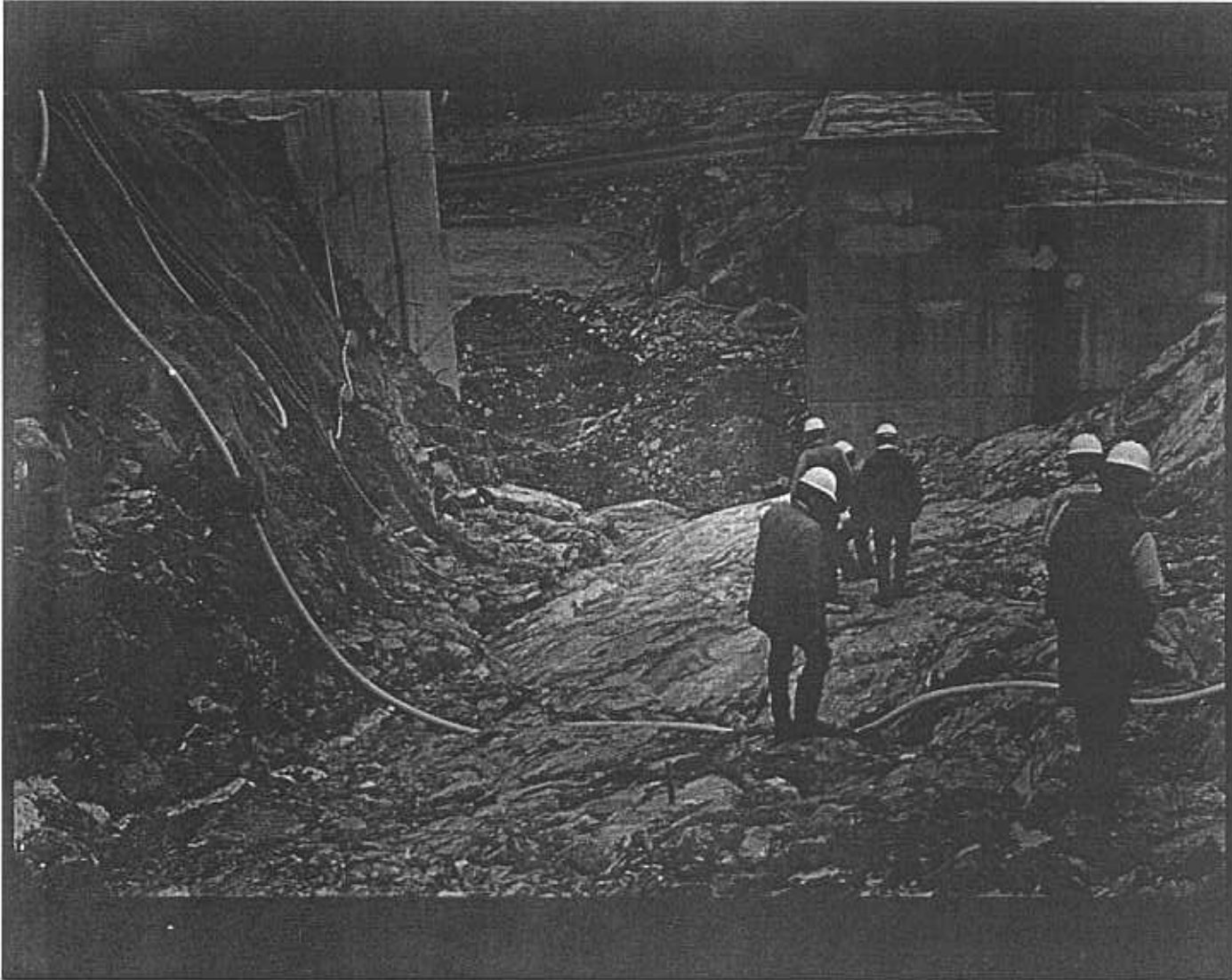
Figure 11.— Left abutment foundation excavation looking toward the river channel. The fault (F-1) occurs along the toe of the 30-m (100-ft) high cut slope. Photo P801-D-79258
