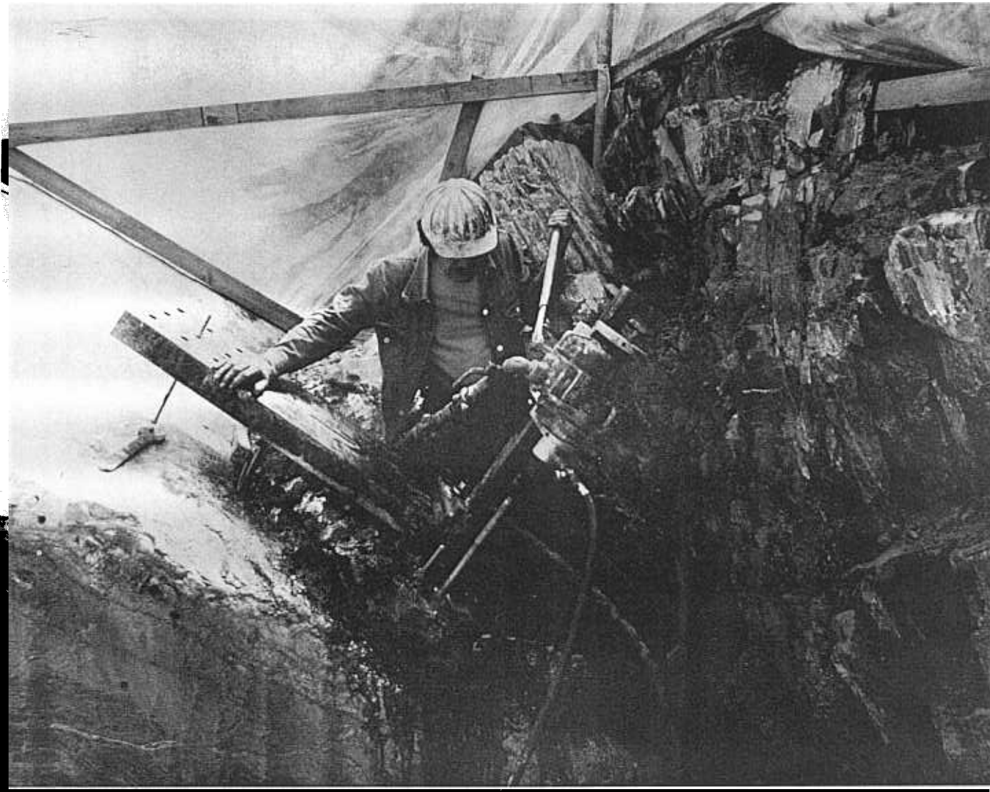
Figure 14. — Air-powered, 25-mm (1-in) diameter core drill used to drill holes into the gouge. There were 34 holes drilled through 100 mm (4 in) of amphibolite. Photo P801-D-79261
