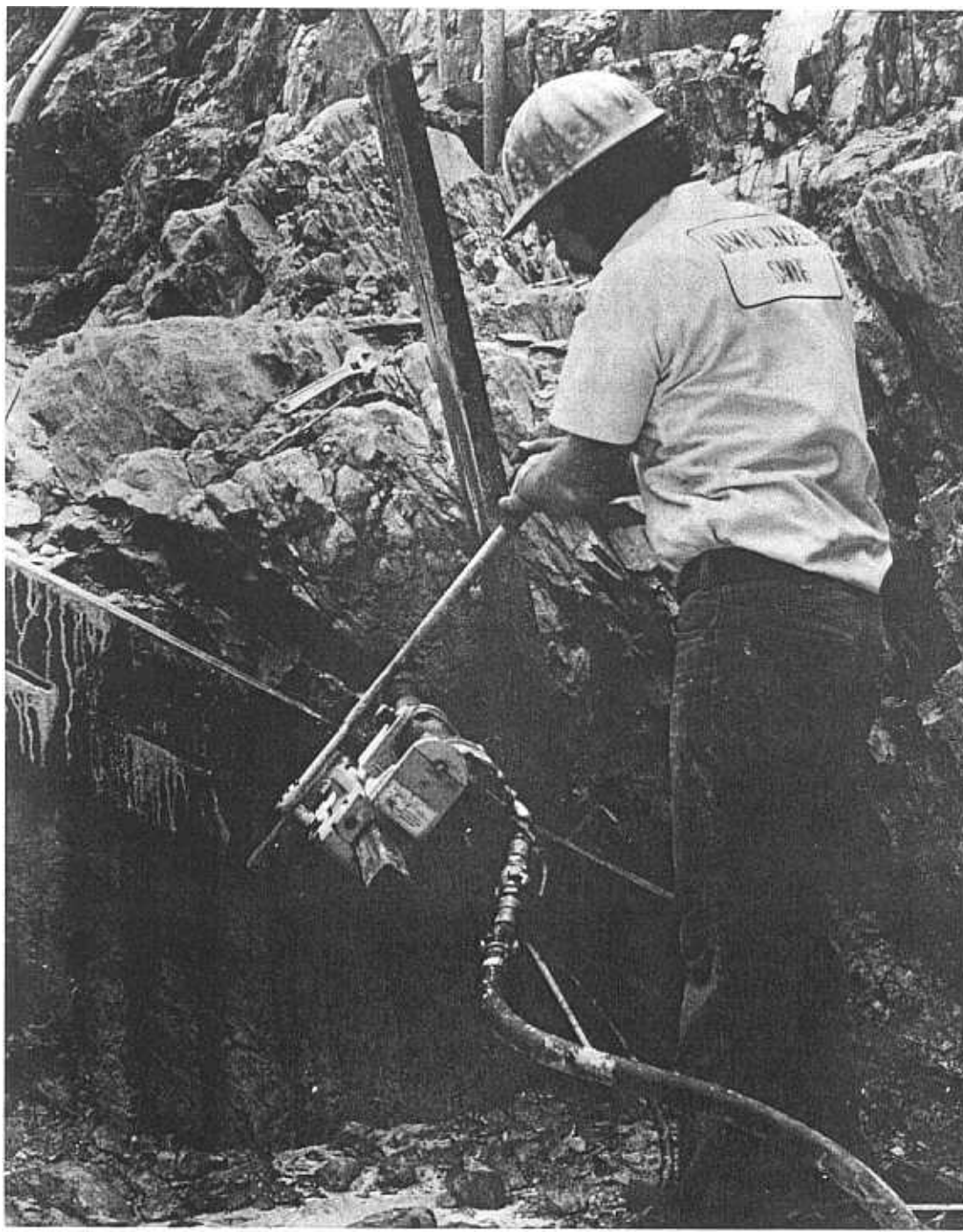
Figure 13.— Air-powered, 75-mm (3-in) diameter core drill mounted on the downslope vertical face. Operator is core drilling a continuous line of holes so that the overburden can be removed without disturbing the fault. Photo P801-D-79260
