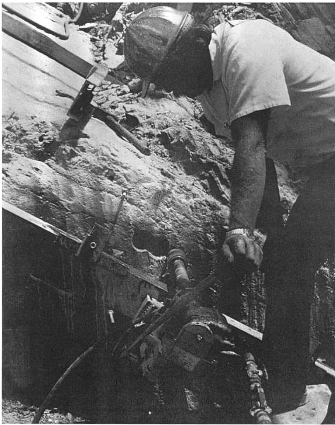
Figure 18.—The air-powered core drill line being used to drill eight 75-mm (3-in) diameter holes to relieve the bottom of the test site. Photo P801-D-79265
