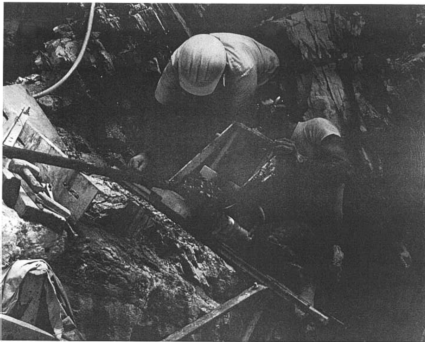
Figure 20. — Mounting the air-powered saw driver onto the track preparing to make the second cut. (This relieved the slabs for removal.) Photo P801-D-79267
