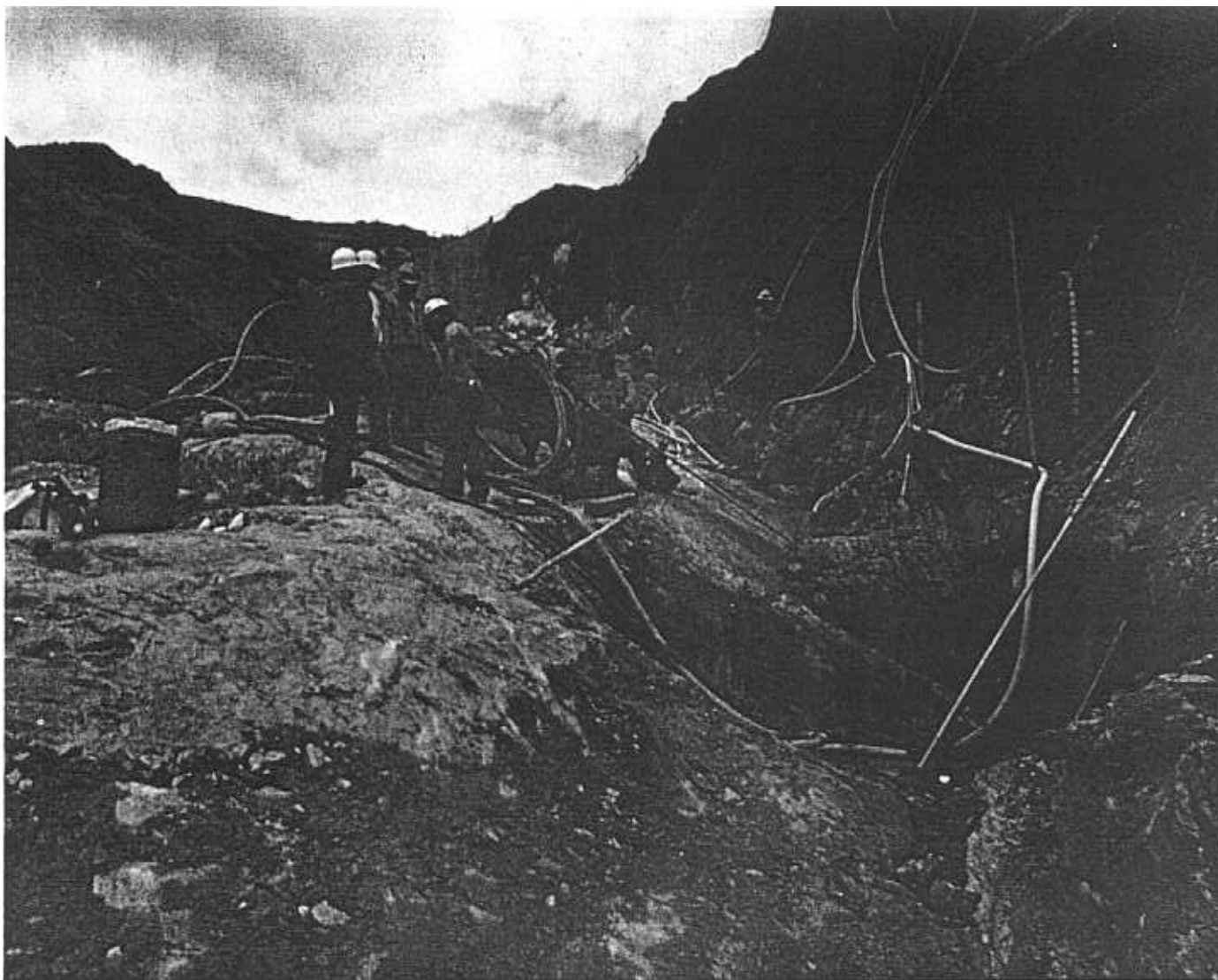
Figure 12.— Exposed vertical wall after controlled excavation in preparation for sampling. Photo P801-D-79259
