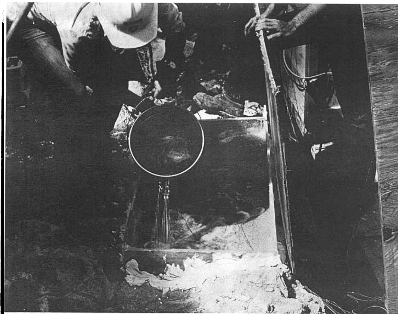
Figure 7. — The low viscosity monomer system is poured into the reservoir to begin impregnation. Photo P801-D-79254
