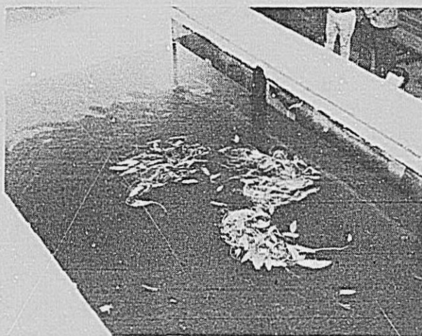
Figure 11. Skimmer weir in operation. Photo P769-D-76121
