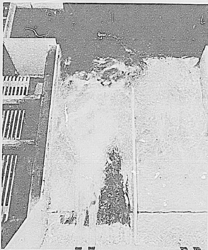
a. Outlets No. 3 and 4, total Q = 4,750 \text{ ft}^3/\text{s} . Photo P296-D-75725
