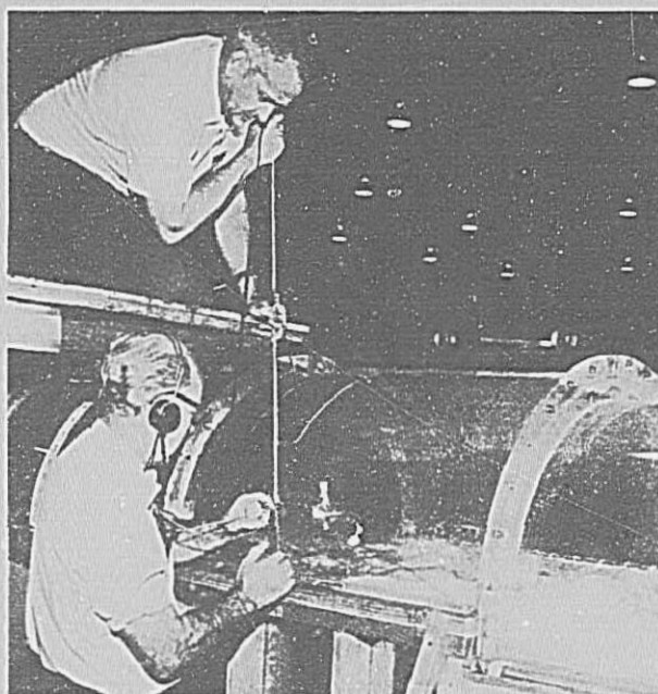
Figure 9. Velocity measuring station 185 feet (56.4 meters) downstream from the valves. Photo P801-D-74266
