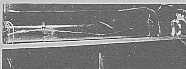
B. View of vortex extending length of conduit. Photo P622-D-74328
