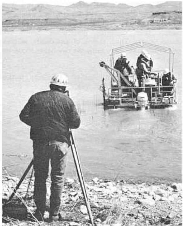
Figure 6. Launching the boat to sound a range line. Photo P24-500-1244 NA
