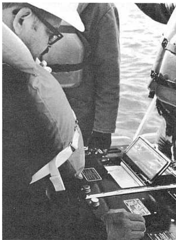
Figure 3. Recorder for sonic charting. Photo P24-500-1246 NA
