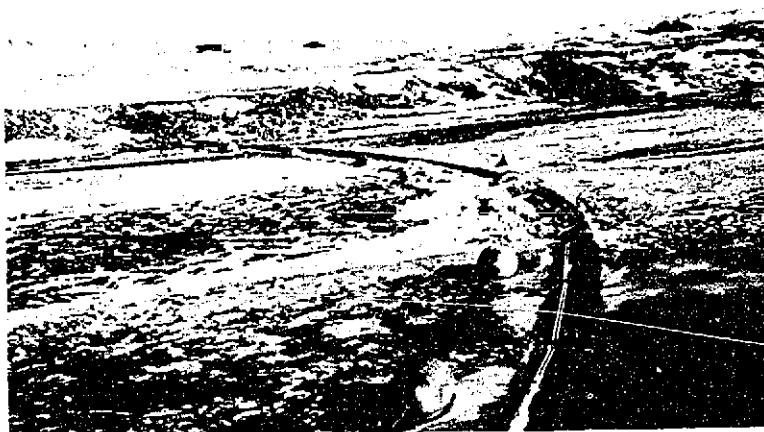
C. Ice control structure. Note float ice in center passing under upstream boom. Photo P20-703-1183
