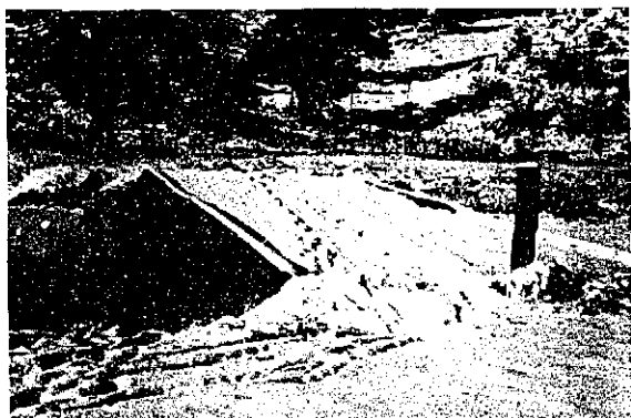
Photograph 5. Canal deer crossing (or bridge) on the Charles Hanson Feeder Canal. Tracks show deer usage. Photo P-245-713-4111 NA
