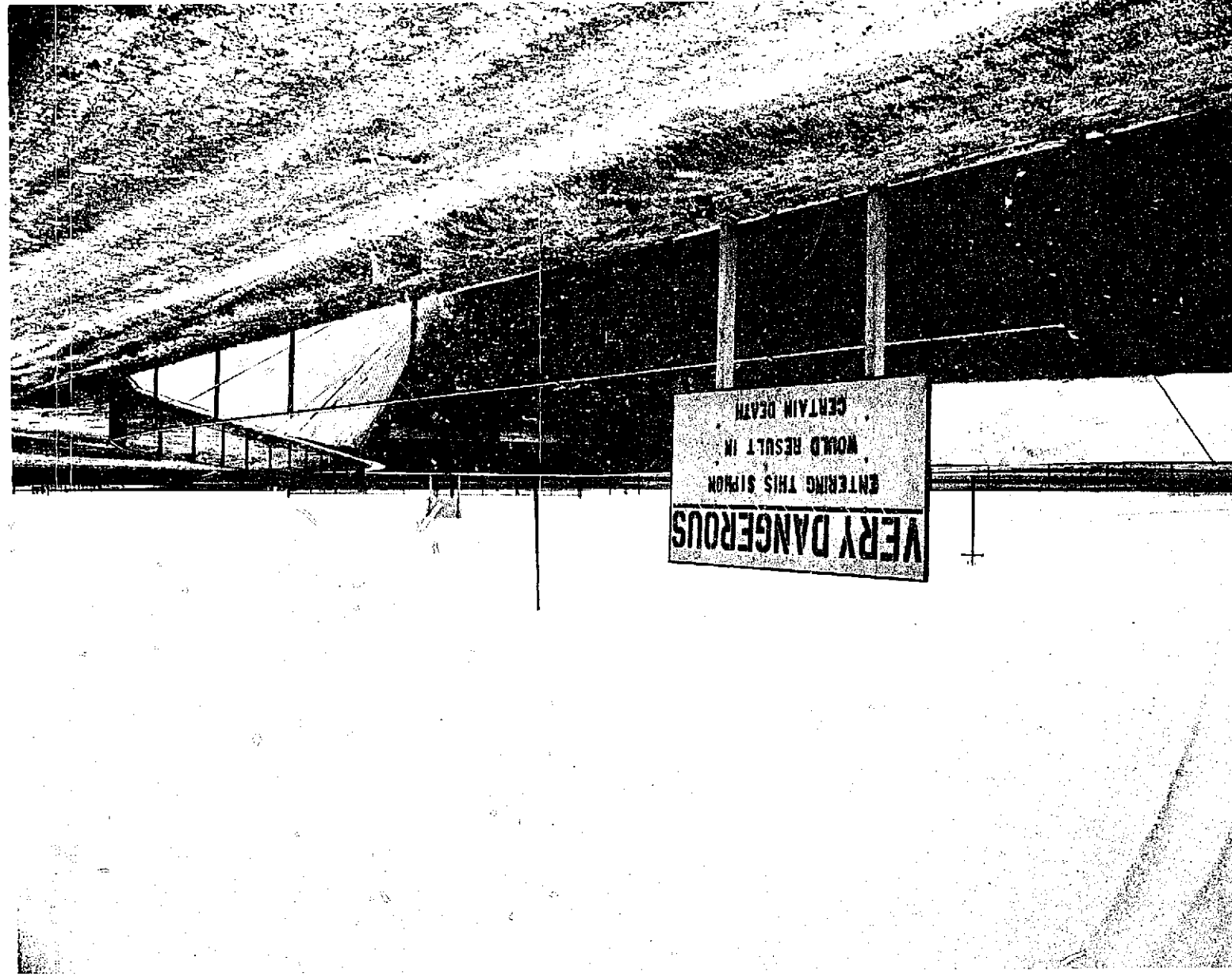
Frontispiece — Safety fence and float at inlet to siphon on the San Luis Canal. Photo P-805-236-14106
