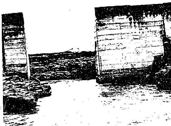
Figure 5. Main channel breach in Rock Canyon Barrier Dam, upstream side. Photo P382-D-69415
