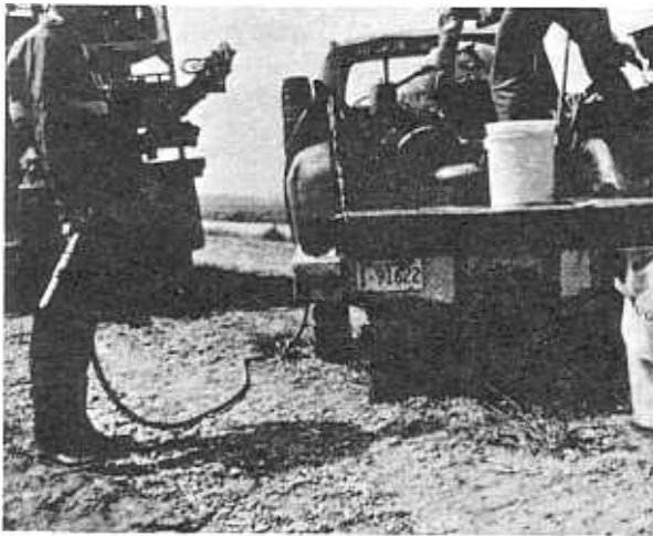
Photograph 24. Treatment of spoil bank for erosion control. A water-base acrylic copolymer was used for the stabilization application. View at left shows spray rig used in application. Left Photo P602-D-69239, right Photo P602-D-69240
