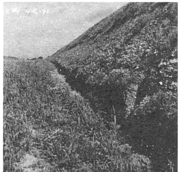
Photograph 27. View at left looking downstream at area to be treated on right bank of the O&M road opposite Mile 0.09, Putah South Canal. Condition after 1 year is shown at right. Slope was stable with a well-defined crust, and the material appeared to penetrate very well in the sandy-gravel deposit. Left Photo P413-D-69245, right Photo P413-D-69246
