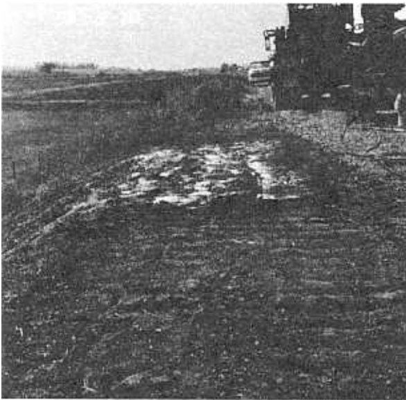
Photograph 26. View at left shows top of left slope immediately after treatment. Condition after 1 year is shown at right. Only a portion of the top slope was treated which resulted in the erosion shown in Photograph 25. This would indicate the need for treating the top of the slope. Left Photo P602-D-69243, right Photo P602-D-69244
