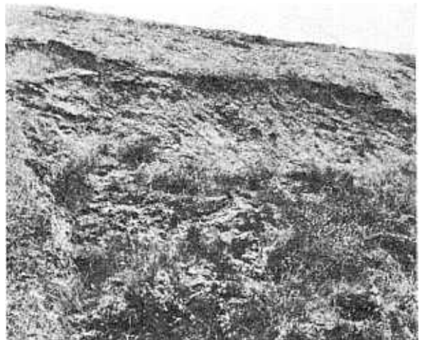
Photograph 23. View of spoil bank opposite Mile 25.0 on the Tehama-Colusa Canal, Central Valley Project, California. This area has a history of sloughing which required rebuilding the fence, shown in Photograph 24, numerous times. Photo P602-D-69238
