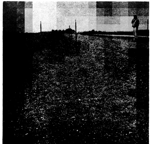
Photograph 26. View at left shows top of left slope immediately after treatment. Condition after 1 year is shown at right. Only a portion of the top slope was treated which resulted in the erosion shown in Photograph 25. This would indicate the need for treating the top of the slope. Left Photo P602-D-69243, right Photo P602-D-69244
