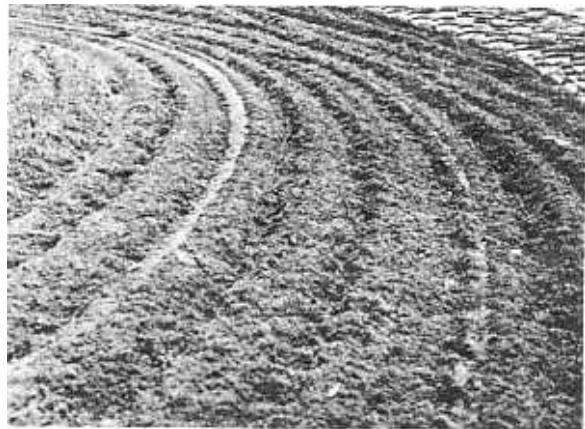
Photograph 19. Fort Thompson-Grand Island 345-kv Transmission Line—A close-up view showing the condition after the first coat of liquid asphalt had been harrowed at USBR Tower No. 174/2. Photo P-466-602-6627
