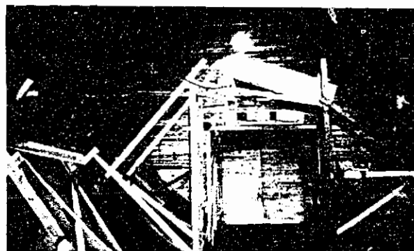
Figure 3-3. View of full tunnel bulkhead just inside of the downstream portal of the spillway tunnel. Photo P459-D-68578
