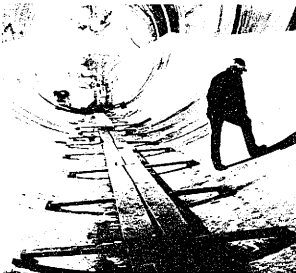
Figure 3-11. Appearance of the spillway tunnel near the end of construction is shown. Note the excellent inspection potential with the white epoxy-phenolic paint coat. Smoothness of the total lining is also apparent. Photo P459-640-998
