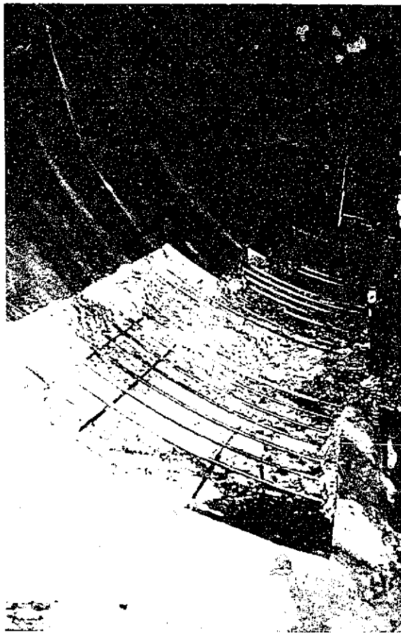
Figure 3-4. View of chipped out damaged Areas A and B showing the saw cut periphery of the damaged area and the partially replaced reinforcement steel mat. Photo P459-D-68576
