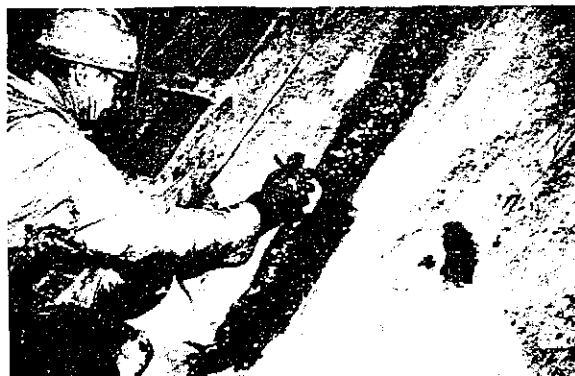
Figure 3-8. Epoxy-mortar repair being made. Finisher is compacting epoxy mortar with wooden tamper. Photo P459-D-68812
