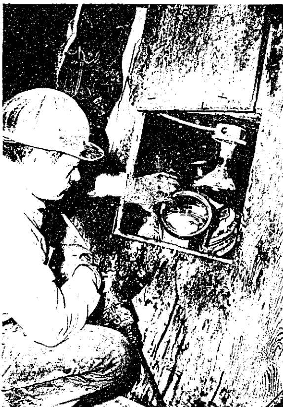
Figure 3-9. Wooden storage compartment for warm storage of epoxy components. Material temperatures of 75° to 80° F were maintained in this simple setup. Photo P459-640-1004 NA
