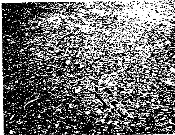
Figure 1-1. Typical erosion pattern in the invert lining. Photo P459-640-3667 NA
