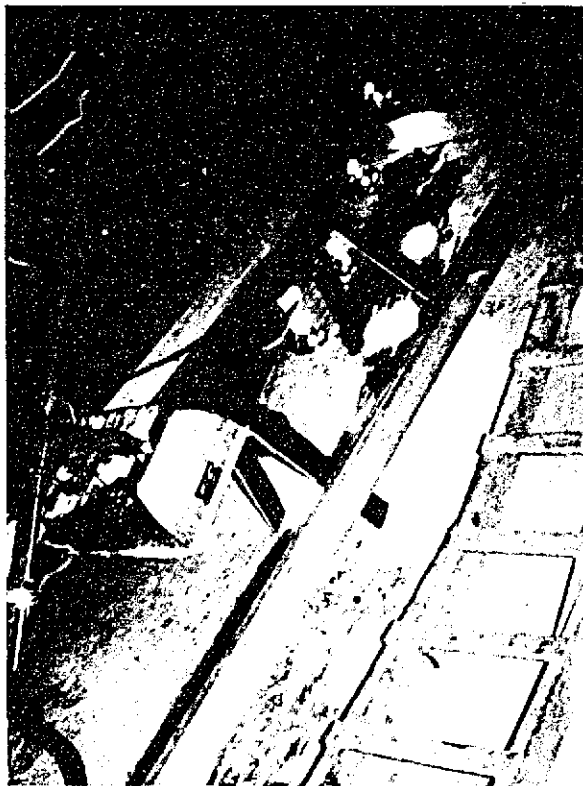
Figure 3-10. Bank of infrared lamps and a propane-fired radiant heater being used to post cure epoxy-mortar patches. Photo P459-D-68813
