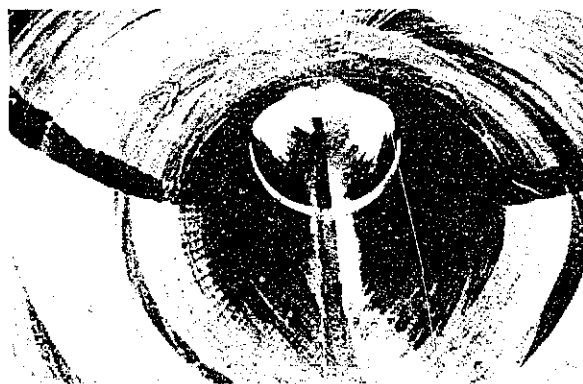
Figure 3-19. Completed repair work. View looking upstream into bend of tunnel. White slash in center of photograph is the completed aeration slot. Photo P459-D-68573
