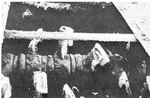
Figure 25. Inside of pugmill, shafts turn in opposite directions while spray bars supply water—Cheney Dam. Photo P835-D-58951
