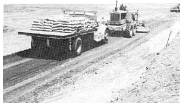
Figure 20. Final compaction by pneumatic-type rolling provided by a loaded truck. Bonny Test Section. Photo P331-700-26
