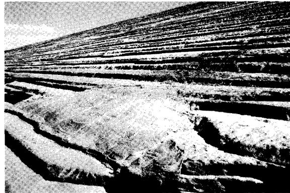
Figure 45. View of patch on Cheney Dam at Station 85+80—October 1971, 1-1/2 years after patch was placed. Photo P835-D-70306.
