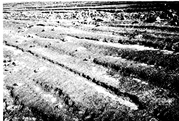
Figure 49. General view of Lubbock Regulating Reservoir showing weathered material, Sta. 51—March 1968, 1 year after construction. Photo P719-D-66536
