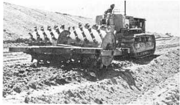
Figure 19. Initial compaction of the soil-cement with a sheepfoot roller. Bonny Test Section. Photo P794-701-561
