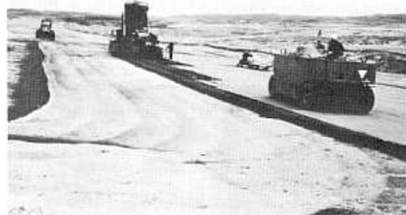
Figure 33. Placing and rolling second lift—Merritt Dam upstream slope modification. Photo P719-701-7
