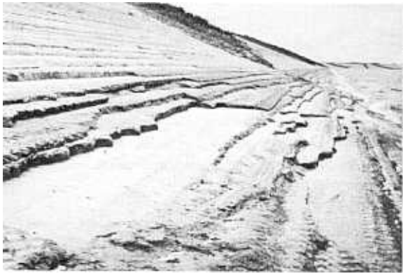
Figure 41. View of Cheney Dam at Sta. 85+75 showing moderate breakage of facing—October 1966, 3 years after construction. Photo P835-D-56106
