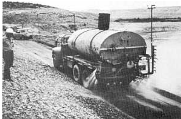
Figure 35. Watering inplace soil-cement—Starvation Dam. Photo P66-D-66533
