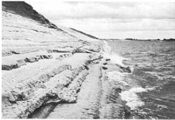
Figure 40. View of Cheney Dam at Sta. 110+00 showing moderate breakage of facing—October 1966, 3 years after construction. Photo P835-D-56108
