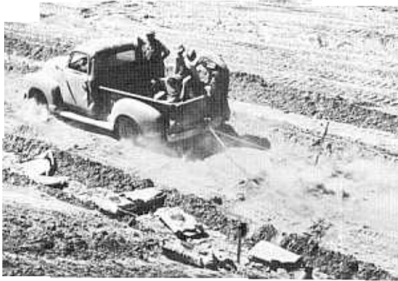
Figure 16. Distribution of the dumped cement on soil layer with a spiked-tooth harrow prior to the start of the mixing in-place operation. Bonny Test Section. Photo P704-701-550
