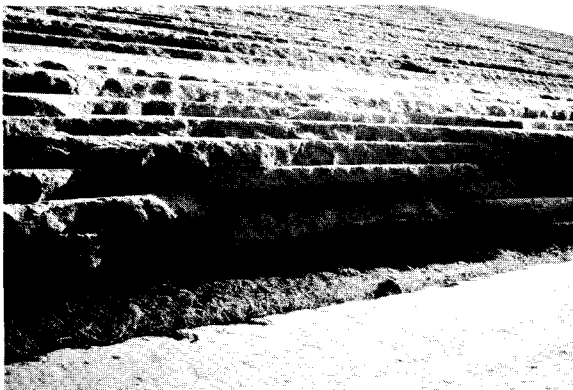
Figure 44. Closeup view of Cheney Dam at Station 95+90 showing Zone 1 material exposed—October 1971, 8 years after construction. Photo P835-D-70510
