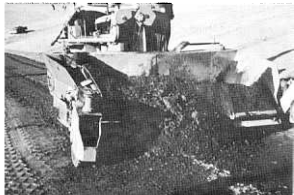
Figure 28. Closeup view of spreader box used to place even, uniform lift—Merritt Dam. Photo P719-D-58949
