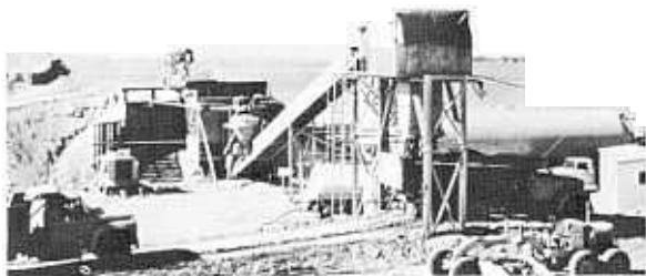
Figure 22. General view of soil stockpile and pugmill for mixing soil-cement—Lubbock Regulating Reservoir. Photo P719-D-58953
