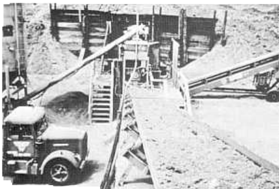
Figure 24. Cement vane feeder and soil feed belt to pugmill—Cheney Dam, Photo P719-D-58954
