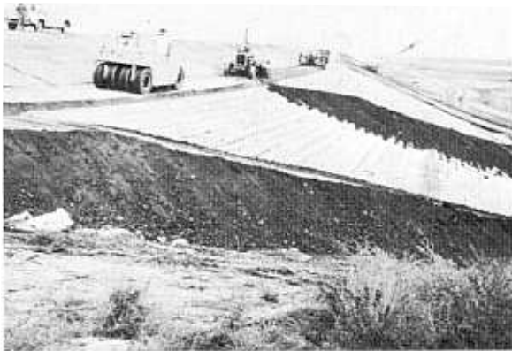
Figure 32. General view of placing and rolling operations—Cawker City Dike. Photo P495-731-460
