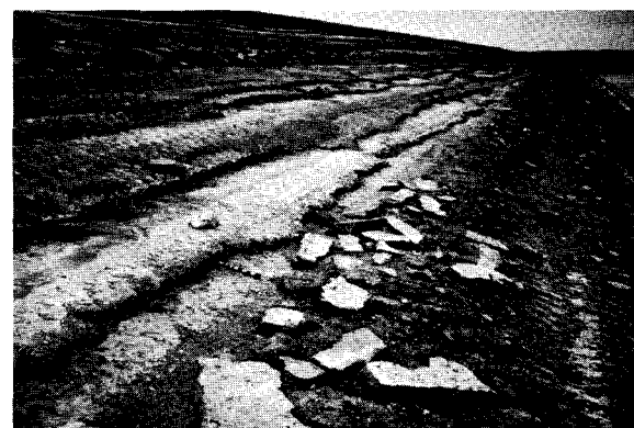
Figure 51. View of Lubbock Regulating Reservoir showing erosion of feathered edge—March 1968, 1 year after construction. Photo P719-D-66535
