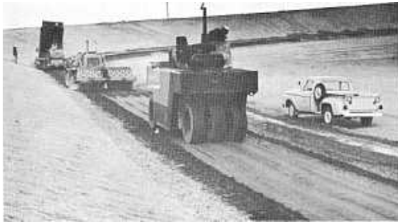
Figure 31. General view of placing and rolling operations—Lubbock Regulating Reservoir. Photo P662-525-5763
