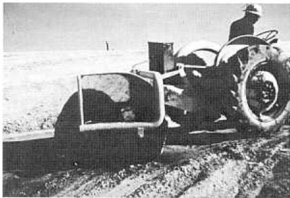
Figure 34. Power brooming to clean surface prior to placement of next lift—Lubbock Regulating Reservoir. Photo P719-D-58948
