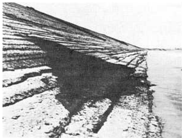
Cheney Dam, Wichita Project, Kansas. Protective surface repair on Cheney Dam. Material was 2,500-pound transit-mix concrete shaped to configuration of soil-cement. Photo P835-D-68954
