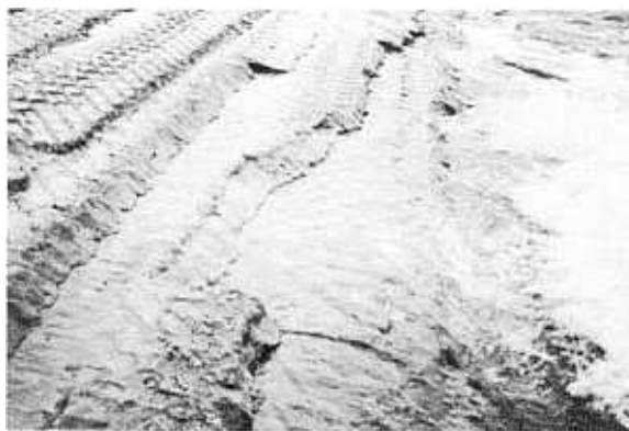
Figure 38. View of Cheney Dam at Sta. 67+50 showing normally anticipated wear pattern—October 1966, 3 years after construction. Photo P835-D-56104
