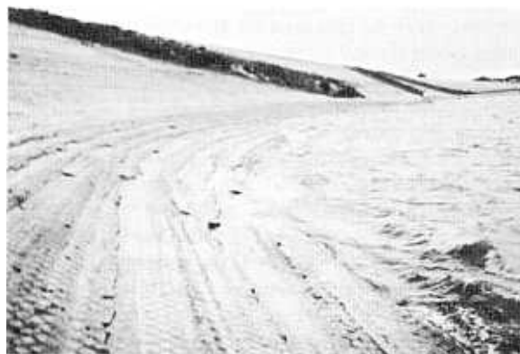
Figure 39. View of Cheney Dam at Sta. 40+00 showing normally anticipated wear pattern—October 1966, 3 years after construction. Photo P835-D-56102
