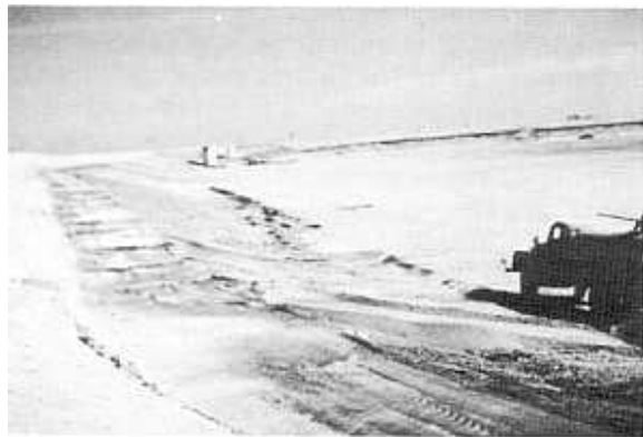
Figure 36. Watering inplace soil-cement with side boom spray—Lubbock Regulating Reservoir. Photo P719-D-66534
