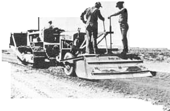
Figure 17. Mixing cement with soil by a tractor-drawn, self-powered, rotary-type mixer. Bonny Test Section. Photo P794-701-557
