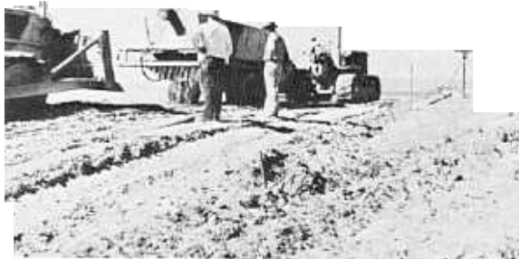
Figure 18. Applying water to soil-cement prior to wet mixing. Bonny Test Section. Photo P794-701-559
