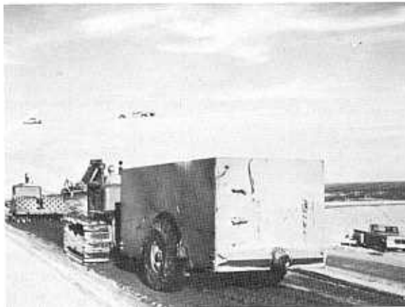
Figure 30. Pneumatic roller used to compact upper portion of lift—Merritt Dam. Photo P719-D-58947
