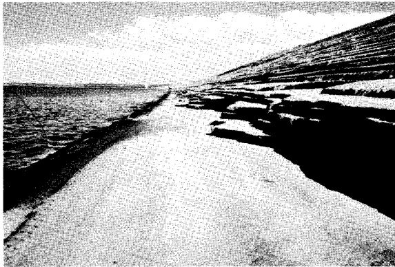
Figure 43. General view of Cheney Dam from Station 88+00 looking east. View shows some of the area of most severe breakage—October 1971, 8 years after construction. Photo P835-D-70305
