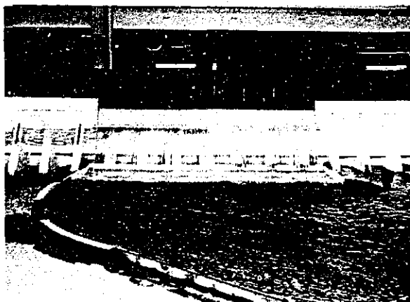
B. Plunge basin design discharge (30,000 cfs or 850 cu m/sec) totally stilled within the basin. Photo P382-D-69041
