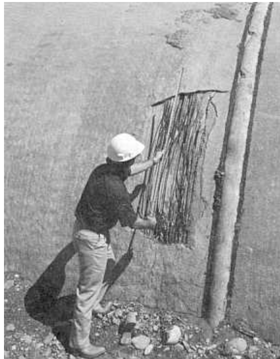
Figure 2. Deteriorated mortar coating with corroded and broken prestressing wire underneath.
