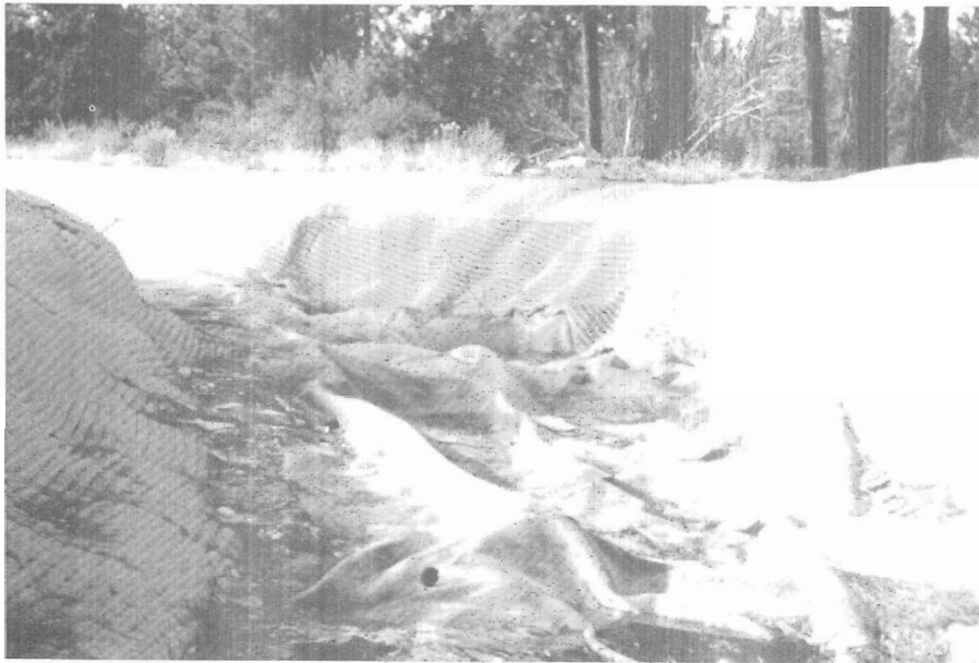
Photograph 34. - Extensive longitudinal wrinkles have developed in the canal invert.
