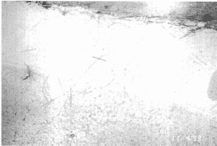
Photograph 8. - Transverse contraction crack.
