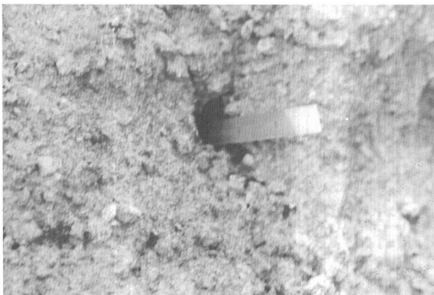
Photograph 68. - Occasional holes in shotcrete up to 4 inches deep.
