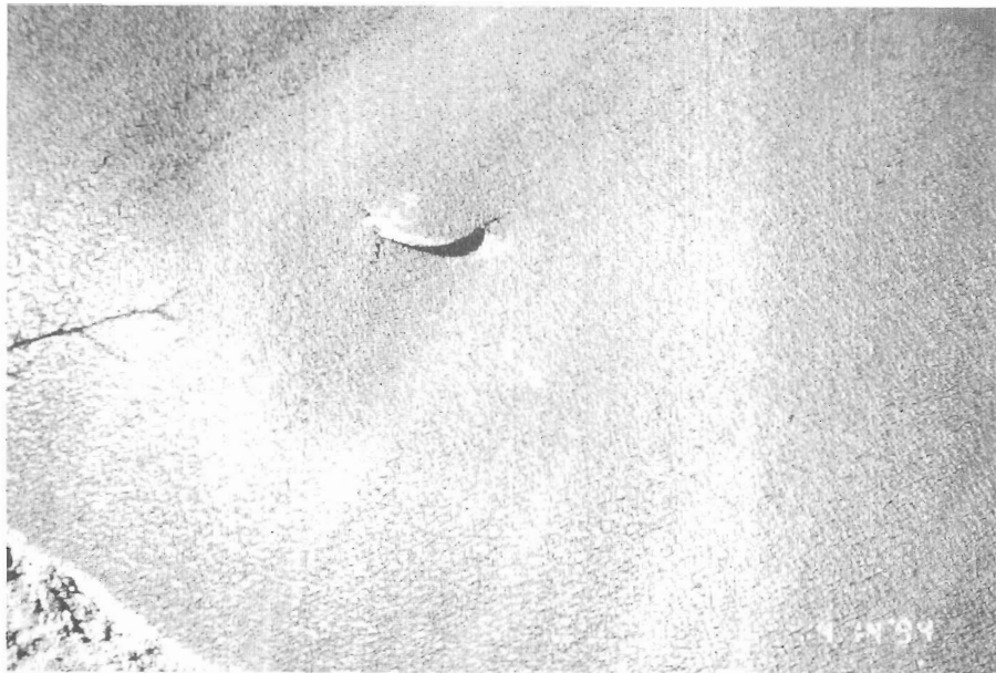
Photograph 12. - Suspected animal hoof damage.
