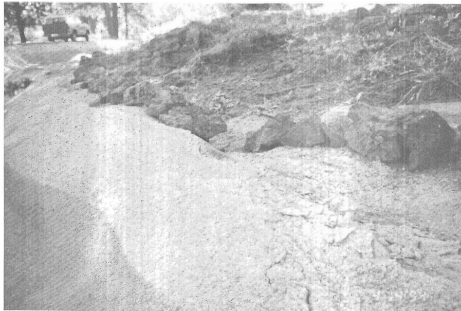
Photograph 6. - Tapered shotcrete over anchor trench has been damaged (cracked) by foot traffic.
