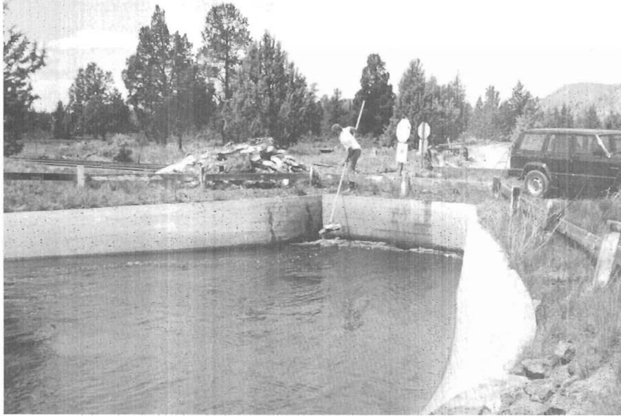
Photograph 53. - Irrigation district removes washed-out foam where it collected at siphon inlet.
