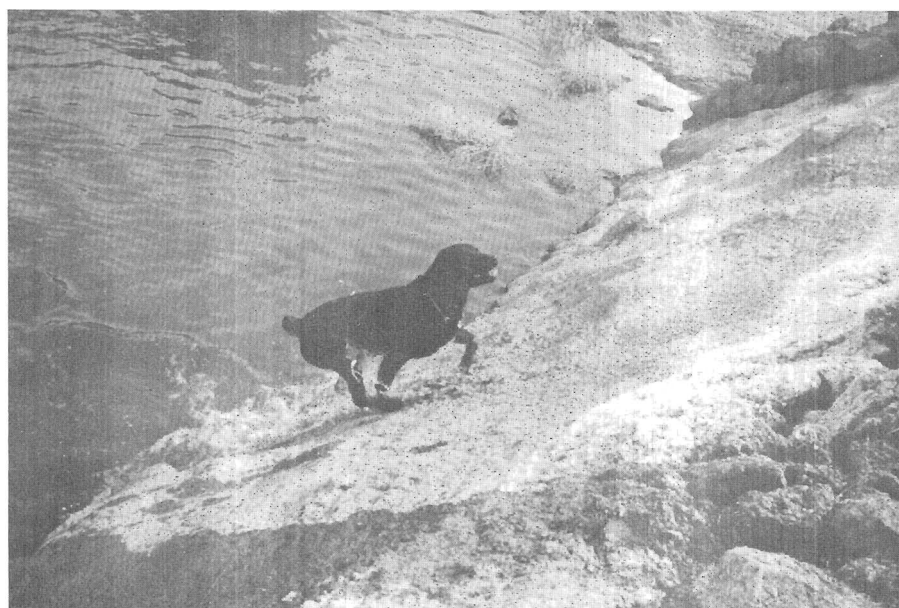
Photograph 75. - Rough shotcrete surface allows for animal escape.
