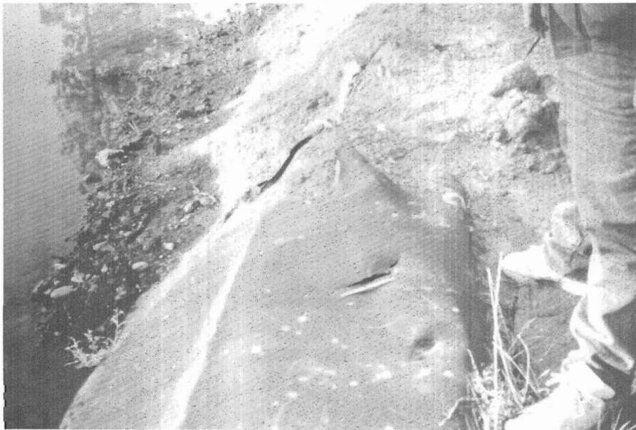
Photograph 14. - Backhoe damage at upstream dike.
