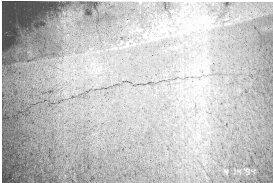
Photograph 4. - Longitudinal contraction crack in shotcrete lining.
