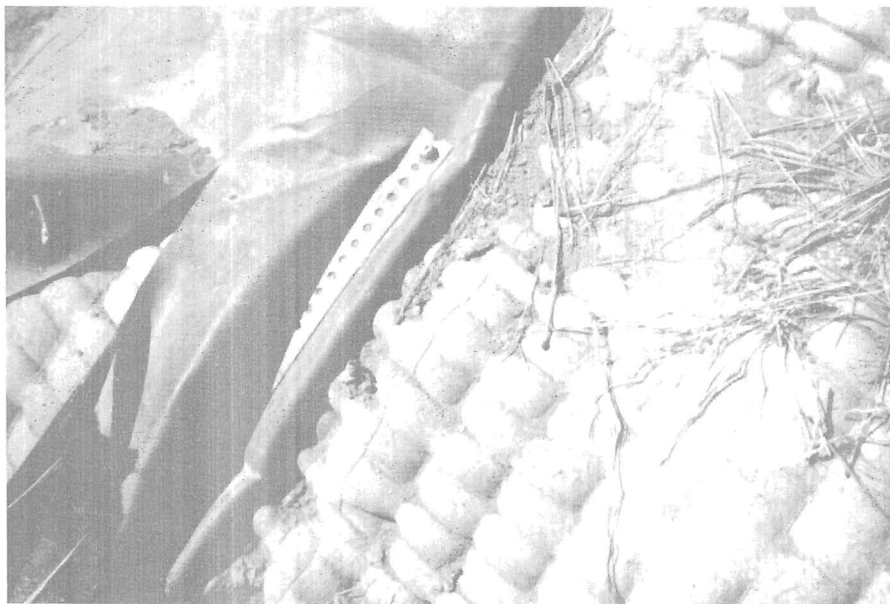
Photograph 28. - Batten strip ties exposed Hypalon into grout mattress in adjoining test section.
