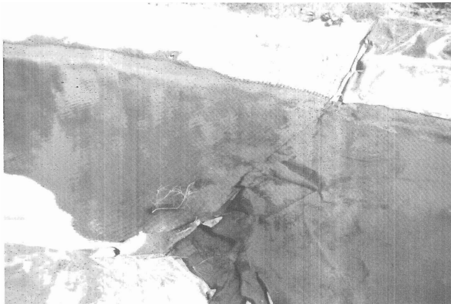
Photograph 26. - Cuts in geomembrane in invert at downstream dike need to be repaired.
