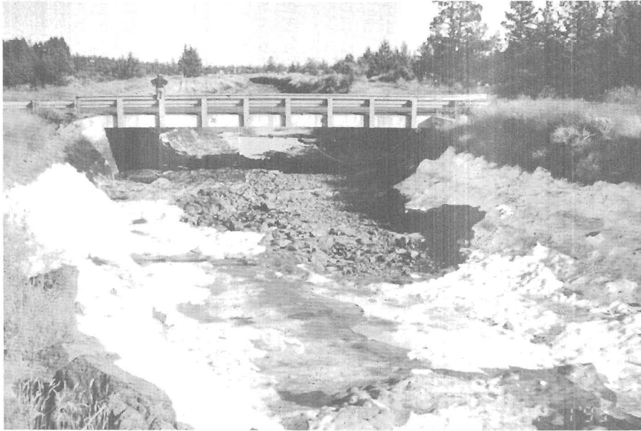
Photograph 45. - Canal overview—foam in the invert has washed out near the bridge.
