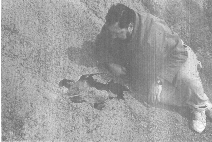
Photograph 69. - Two-foot-diameter hole in shotcrete on left bank. Shotcrete is only about 1 inch thick at this location.
