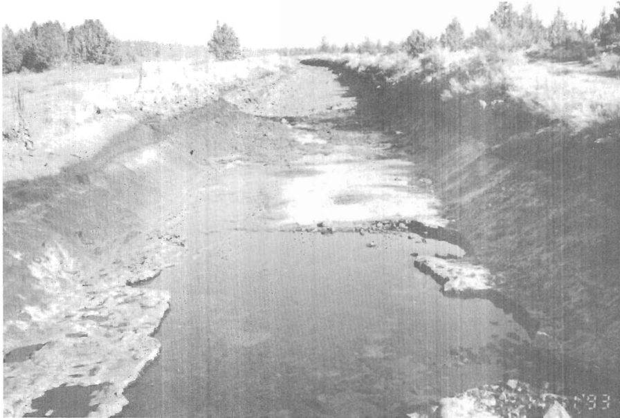
Photograph 51. - Canal overview—partially failed. Foam has washed out under bridge in upstream half of this test section.
