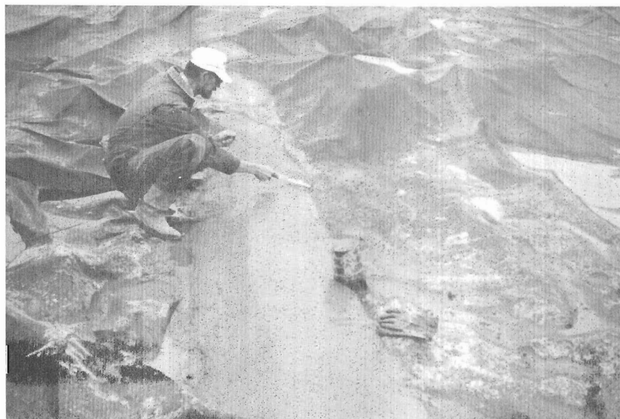
Photograph 56. - Irrigation district repairs seam with a concrete cap.
