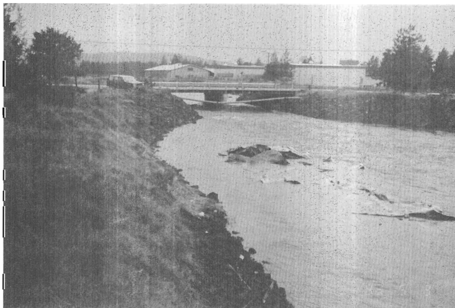
Photograph 62. - Runaway floating geotextile liner damaged the pipe crossing shown near bridge.
