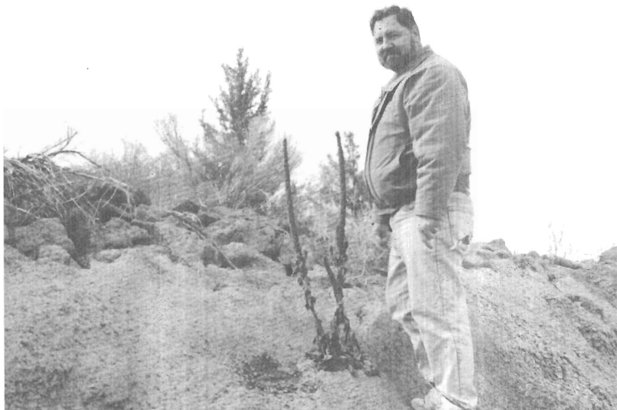
Photograph 67. - Vegetation occasionally growing out of shotcrete on side slopes.
