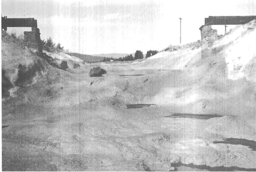
Photograph 72. - Drop section with smaller cross-section and higher velocities.
