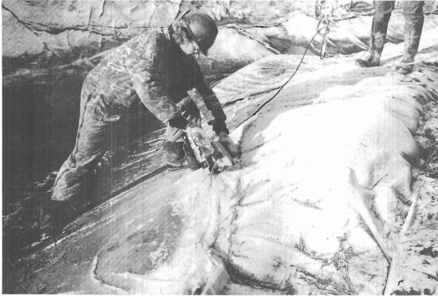
Photograph 19. - Contractor sewing geotextile seams.
