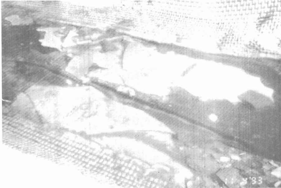
Photograph 41. - White "chalky" portland cement deposits in invert.
