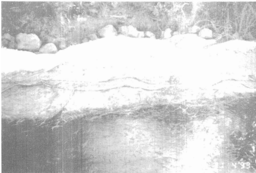
Photograph 18. - Dirt and sediment collecting on geotextile provides additional UV protection.
