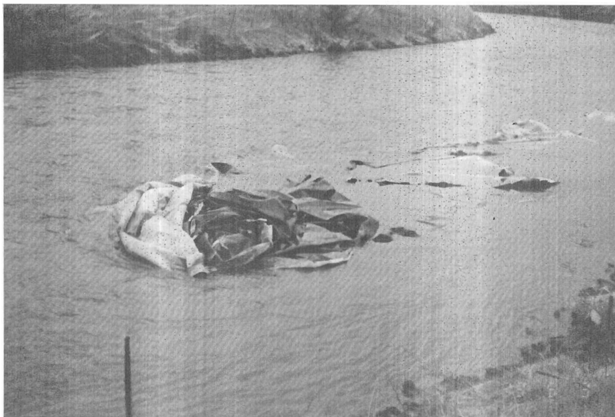
Photograph 61. - Sections of geotextile liner tore loose when the canal was filled with water.
