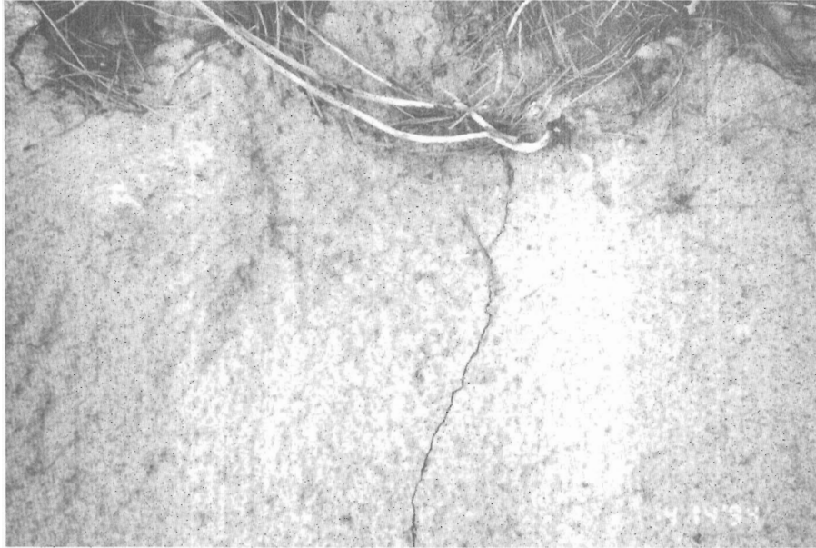
Photograph 3. - Transverse contraction crack in shotcrete lining.
