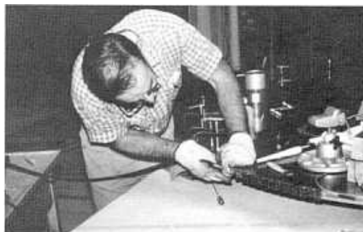
Figure 46. - The wire was cut and the strain relaxation was recorded.
