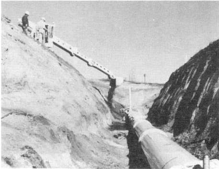
Figure 15. - Soil being dumped into trench.
