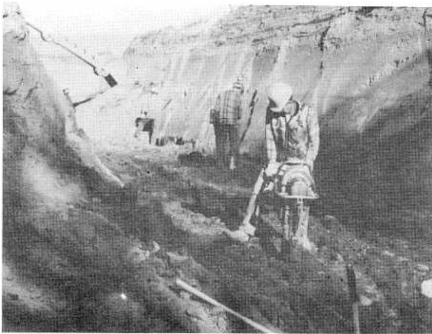
Figure 16. - Compaction using a wacker.
