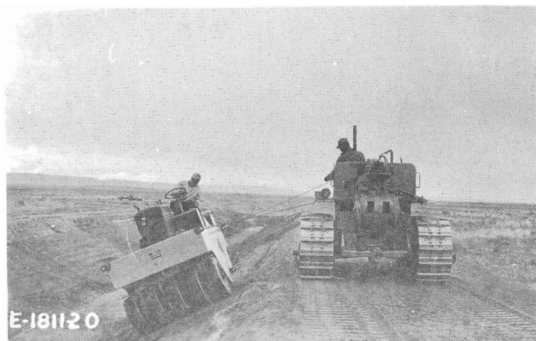
Figure B-9. - Compaction of soil-cement on lateral side slopes with a self-propelled, pneumatic-tired roller attached by cables to a tractor.
