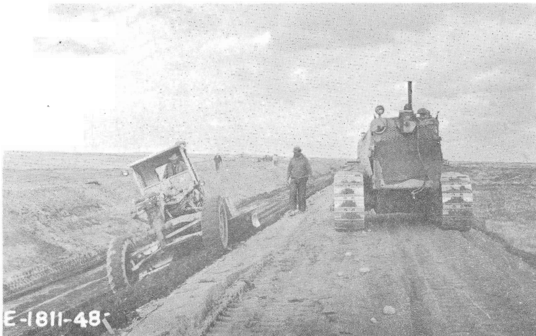
Figure B-8. - Use of a grader to spread soil-cement on the lateral side slope.
