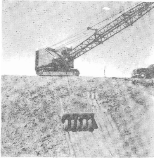
Figure B-6. - A rubber-tired roller compacting loose soil left after compaction by a sheepsfoot roller.
