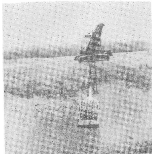
Figure B-5. - Canal side slope compacted by a sheepsfoot roller winched by a dragline.
