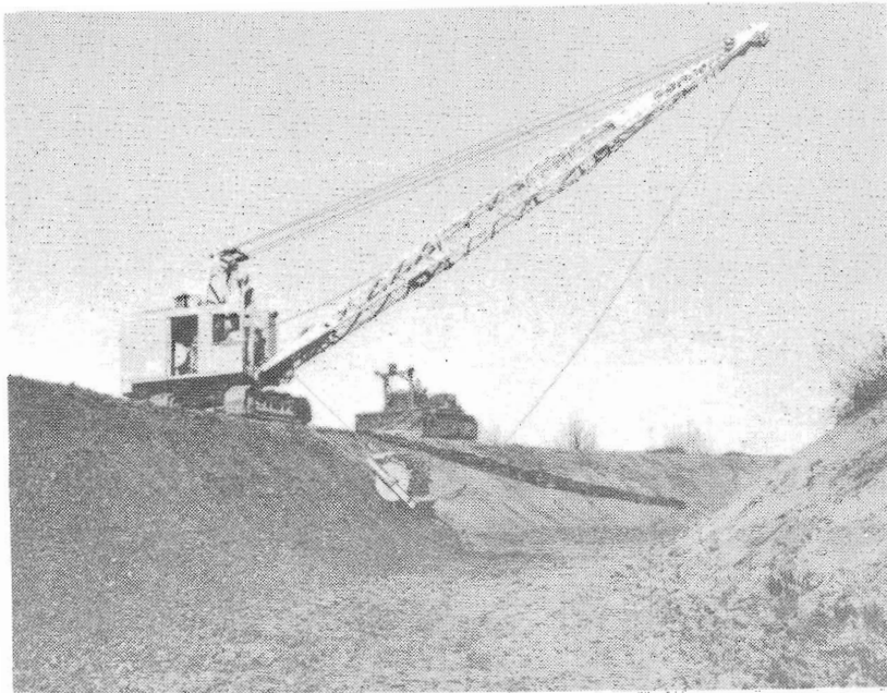
Figure B-1. - Transverse compaction of thin earth lining.
