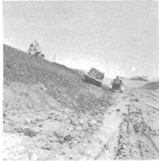
Figure B-7. - A sheepsfoot roller operating longitudinally with canal to compact soil on side slope.
