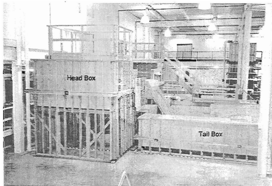
Figure 7.—Folsom Dam model head and tail boxes.
