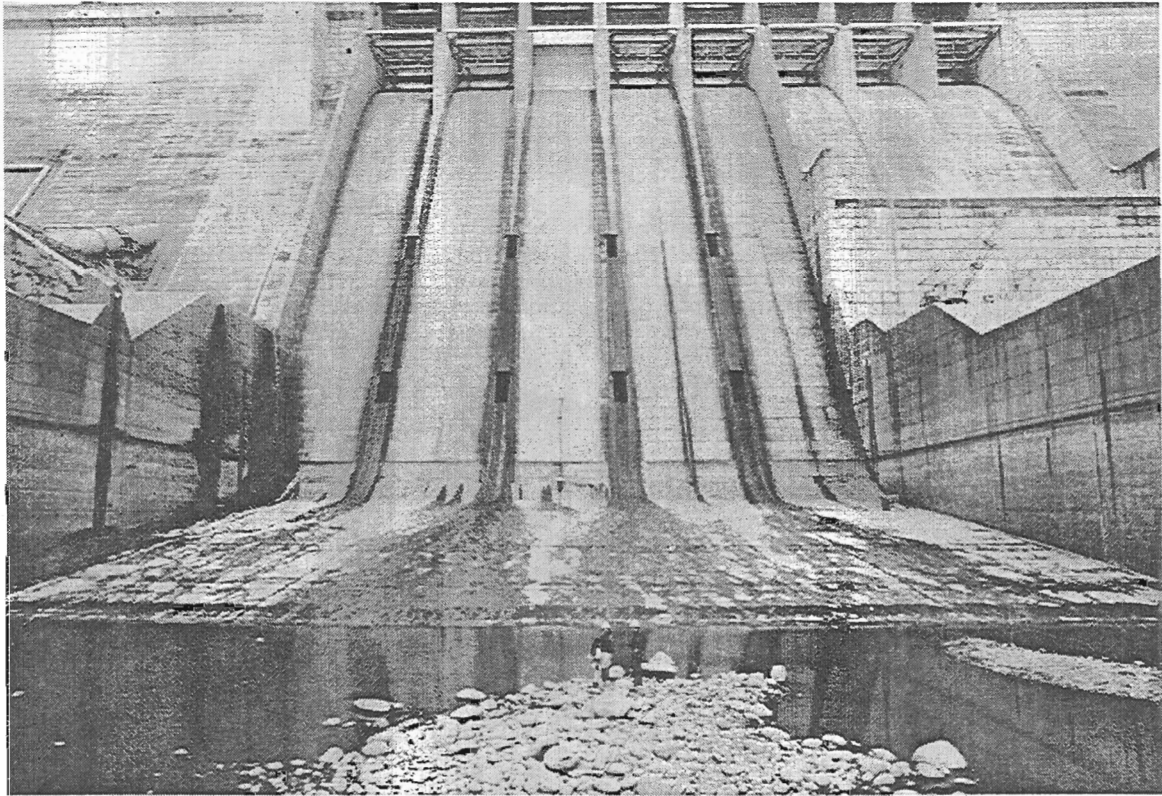
Figure 3.—Folsom Dam's 242-ft-wide service spillway and dewatered stilling basin with accumulated rock debris that caused abrasion damage (1996).
