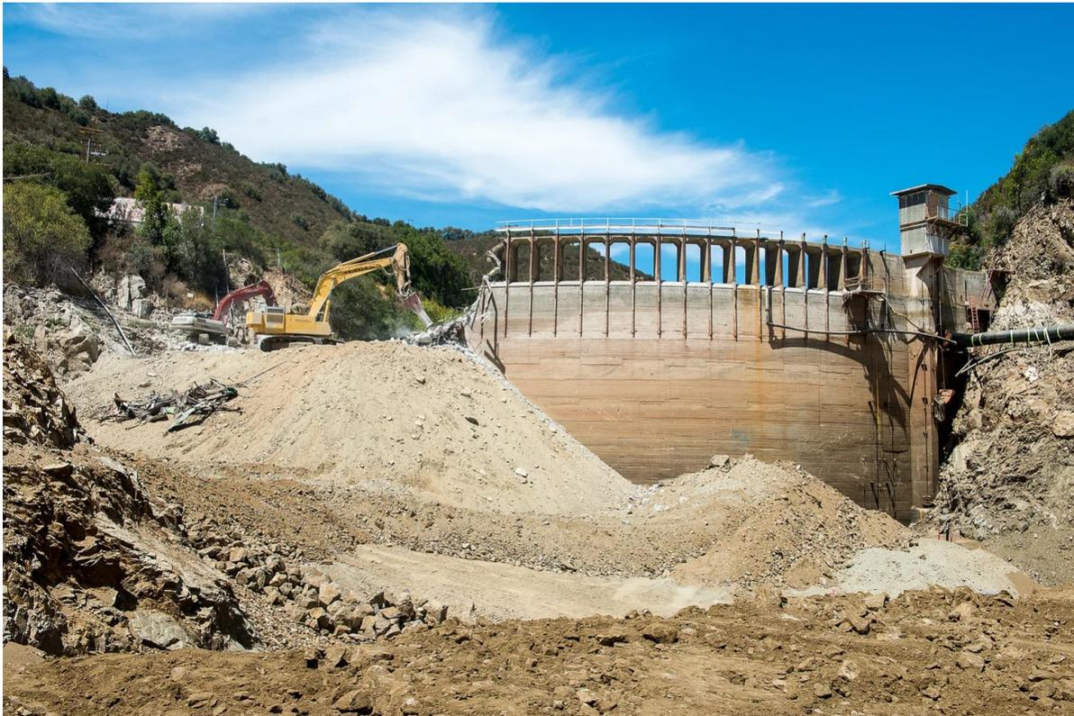
Figure 35. Two large hoe rams were used in the demolition of the dam (photo courtesy of San Clemente Dam Removal and Carmel River Restoration, all rights reserved).
