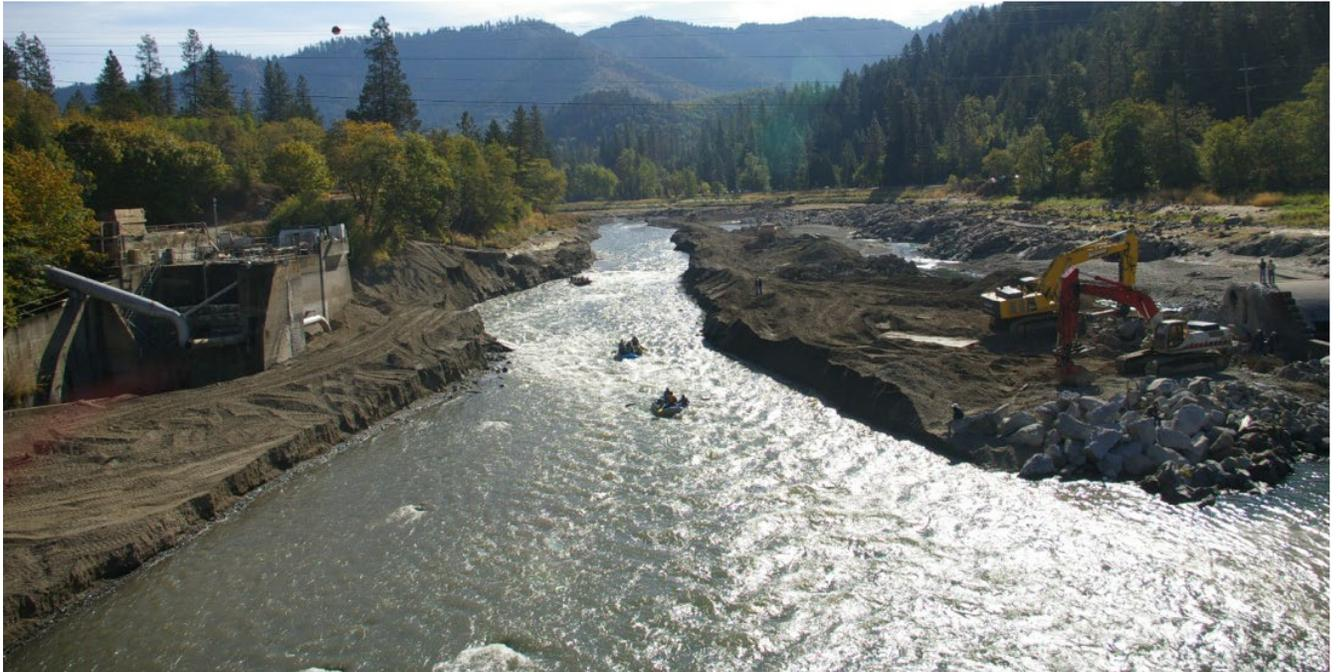
Figure 21. River erosion of reservoir sediments past Savage Rapids Dam near Grants Pass, Oregon, following dam removal (USSD 2015) (Reclamation/Bountry October 2009).
