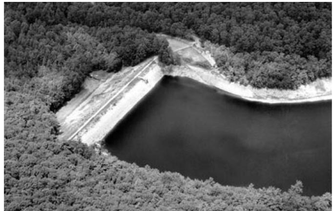
Figure 24. Birch Run Dam before breaching. The spillway can be seen on the right dam abutment (USSD 2015) (Photo courtesy of Johnson et al. 2007, all rights reserved).
