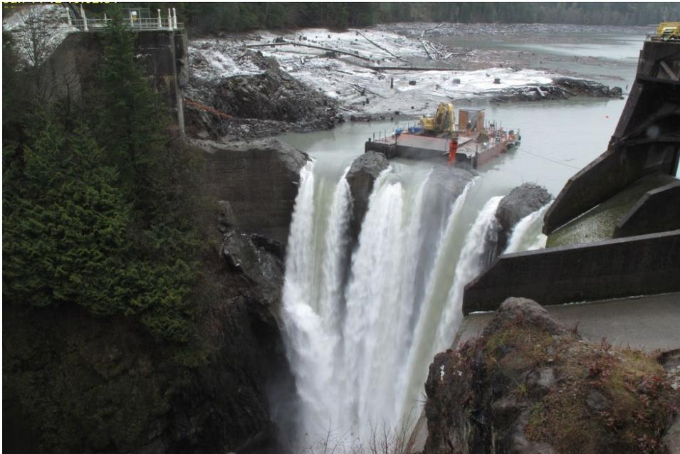
Figure 10. Mechanical excavation of the upper portion of Glines Canyon Dam in Washington, using a hydraulic excavator on a barge (USSD 2015). (Photograph courtesy of National Park Service, January 14, 2012).
