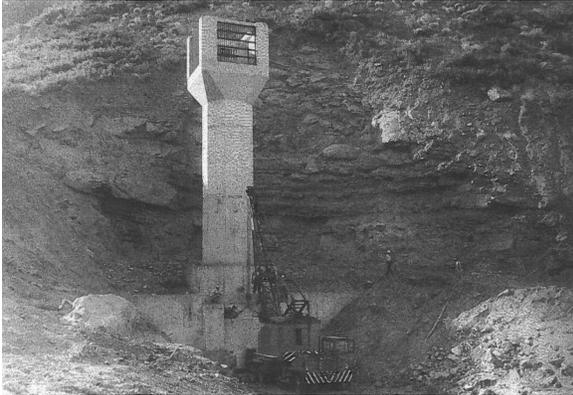
Figure 4. The outlet for Paonia Dam, near Paonia, Colorado, was constructed 21 m above the valley bottom in July 1961.
