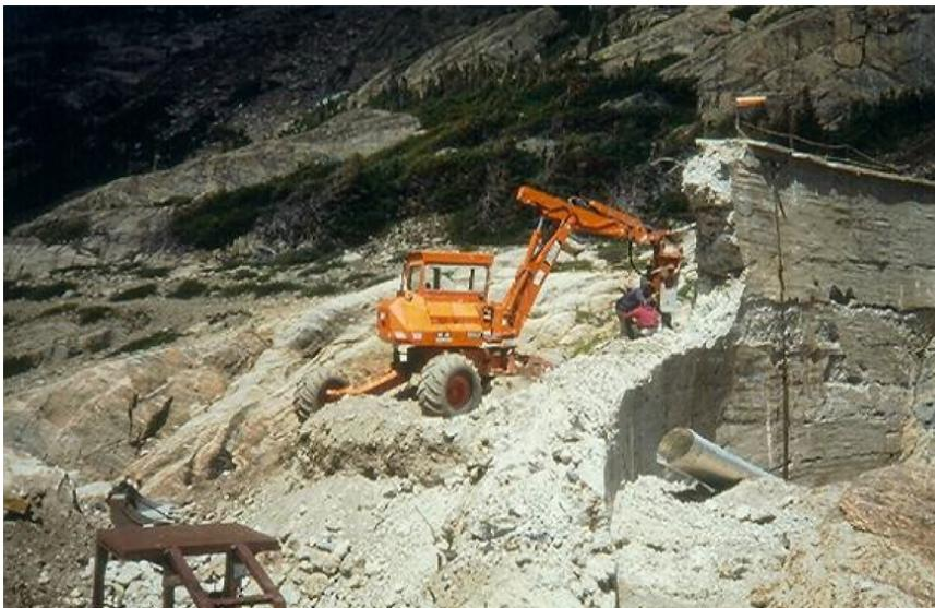
Figure 27. Schaeff Walking Excavator with hydraulic hammer was used in the deconstruction of Bluebird Dam to reduce concrete impacts on downstream greenback cutthroat trout populations (USSD 2015). (Photo credit Karpowicz et al. 2010).
