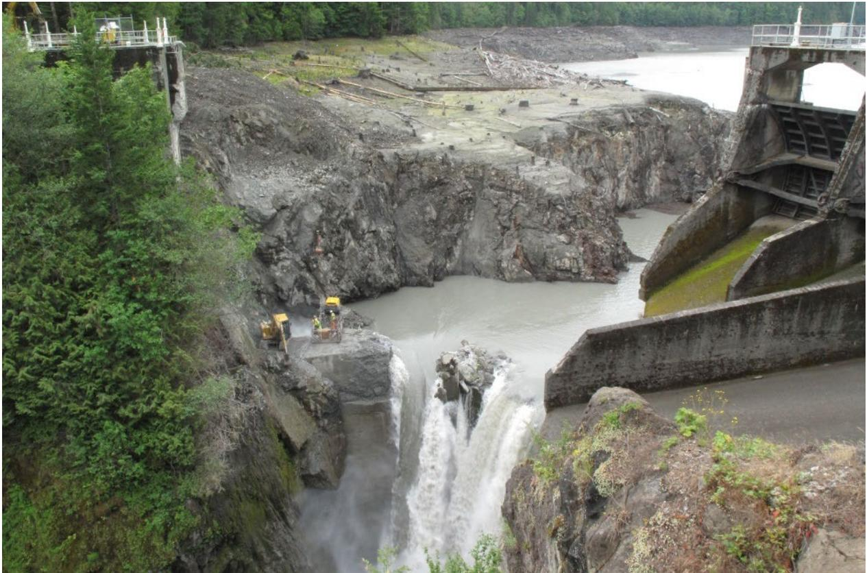
Figure 12. Drilling and blasting notches to excavate the lower portion of Glines Canyon Dam in Washington (USSD 2015) (Photograph courtesy of National Park Service, July 1, 2012).
