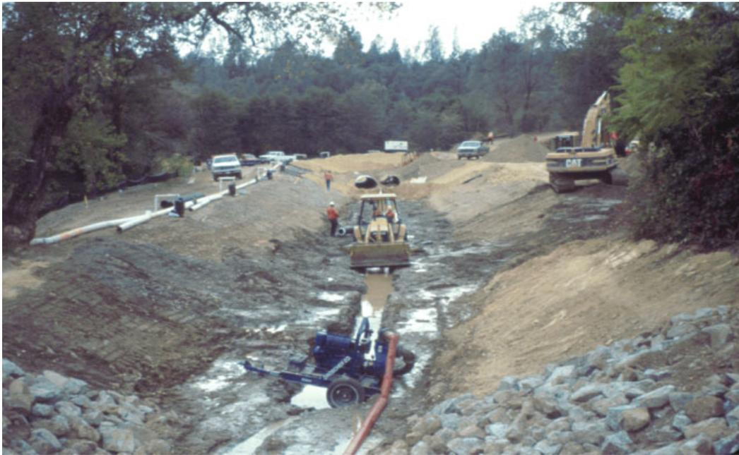
Figure 14. Lined bypass channel designed and constructed for removing Saeltzer Dam and contaminated sediments from Clear Creek in California (USSD 2015) (Reclamation/Hepler).
