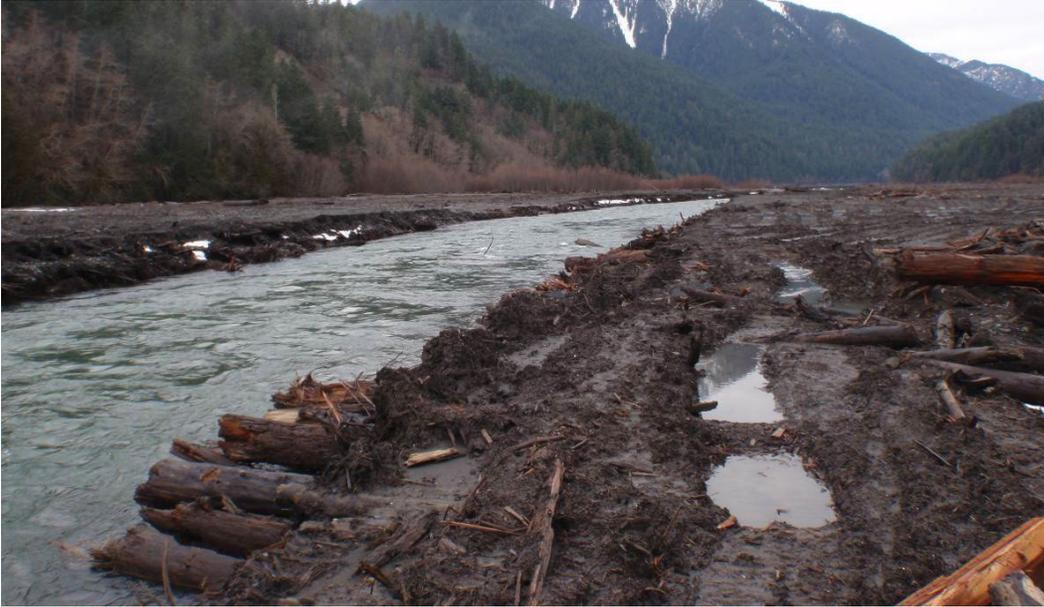
Figure 22. A pilot channel excavated through the Lake Mills delta and alder forest growing on the delta was cleared in preparation to remove Glines Canyon Dam near Port Angeles, Washington (USSD 2015) (Reclamation, December 2010).
