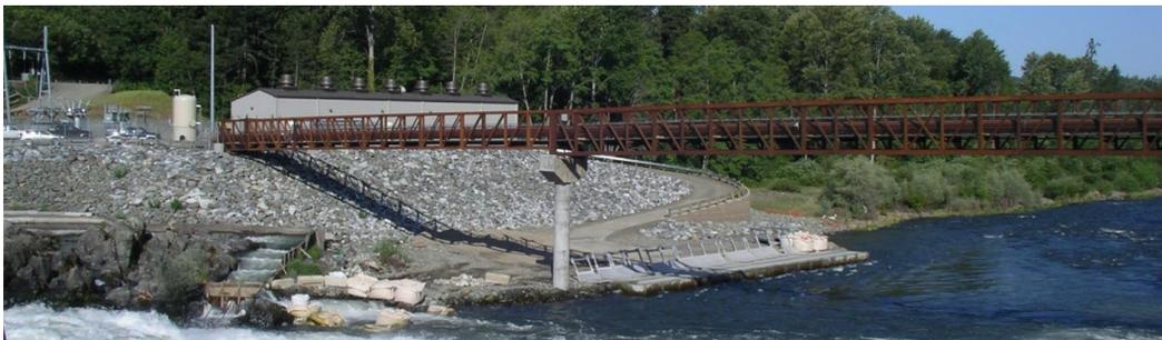
Figure 7. Pump station designed and constructed on the Rogue River in Oregon to replace gravity diversions from Savage Rapids Dam. A pipe bridge was constructed so water could be delivered to both sides of the river (USSD 2015) (Reclamation/Hepler).
