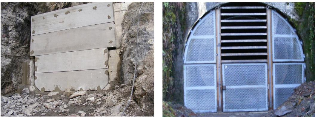
Figure 15. At Glines Canyon Dam, Washington, the upstream tunnel barrier (left) was blocked using precast concrete panels while the downstream tunnel barrier (right) was blocked using metal panels (USSD 2015) (Reclamation/Hepler).
