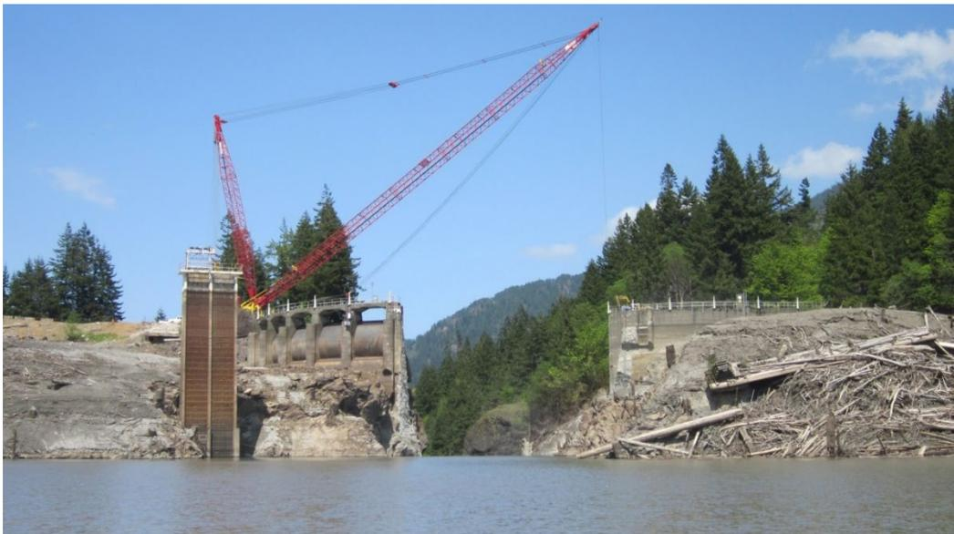
Figure 11. A large ringer crane was employed at Glines Canyon Dam, Washington in 2015 (Reclamation/Randle).
