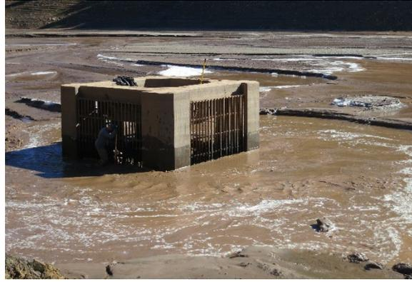
Figure 5. By November 2014, sedimentation and woody debris began to plug the dam outlet.
