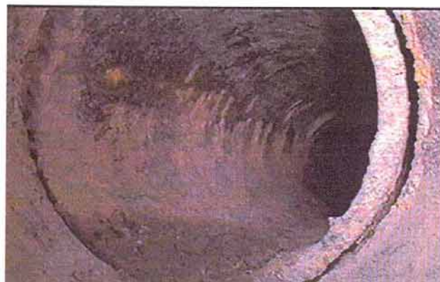
Figure D-10. —Concrete pipe experiencing extensive joint offset and separation at a bend in the pipe.
