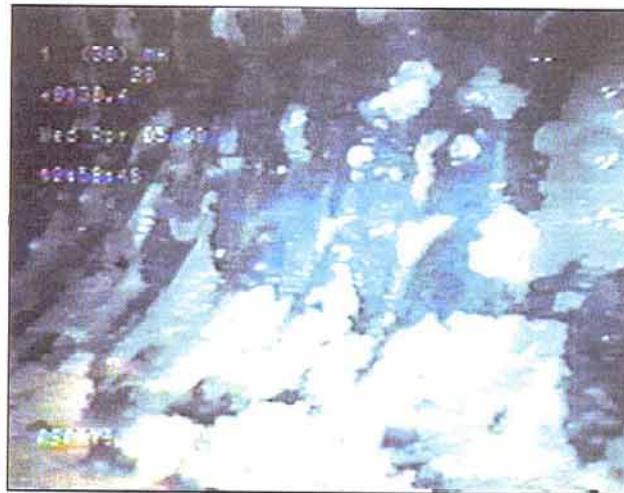
Figure D-9. —CMP pipe experiencing extensive loss of surface coating due to delamination.
