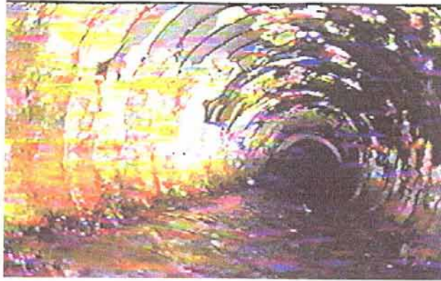
Figure D-8. —Extensive deterioration existing within a CMP pipe.
