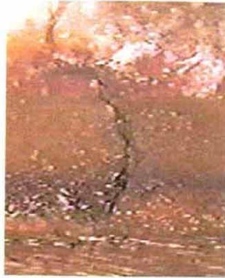
Figure D-11. —Extensive transverse cracking within a concrete pipe.
