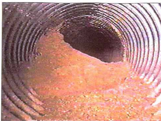
Figure D-7. —An HDPE pipe joint has experienced extensive separation. Materials surrounding the pipe have entered through the separated joint.
