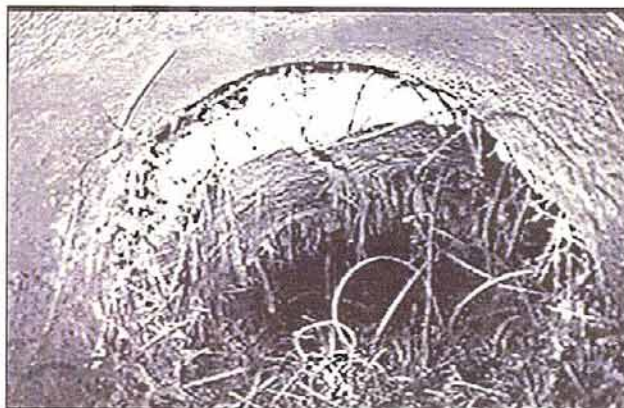
Figure D-4. —Clay tile pipe experiencing inward collapse of the crown.
