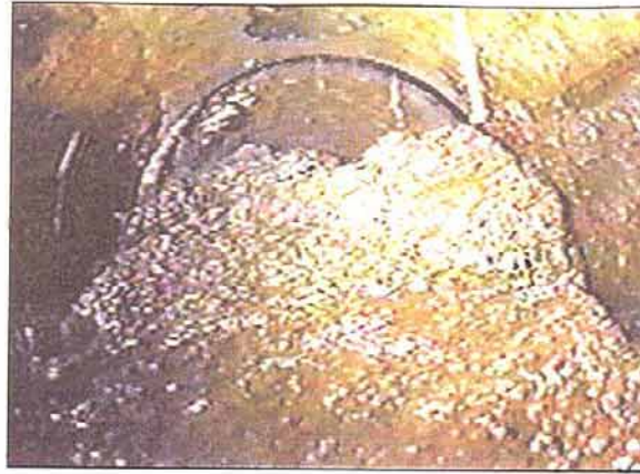
Figure D-13. —Accumulation of sediments has resulted in plugging of the pipe.
