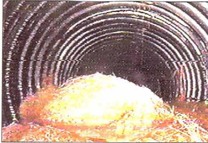
Figure D-16. —Root growth has resulted in partially plugging the pipe.
