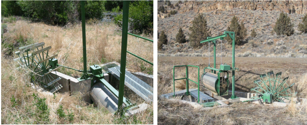
a. Operation – in the dry.
