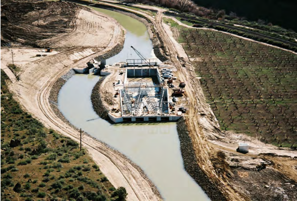
Figure 35.—Site isolation and dewatering for construction, Highline Canal Fish Screen Facilities at Grand Junction, Colorado.
