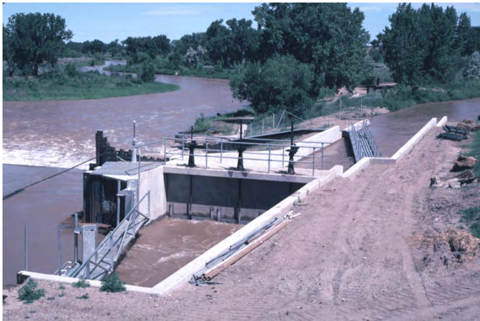
Figure 116.—Overview of T&Y Diversion with fish louver structure – Example 4 (T&Y Irrigation District).
