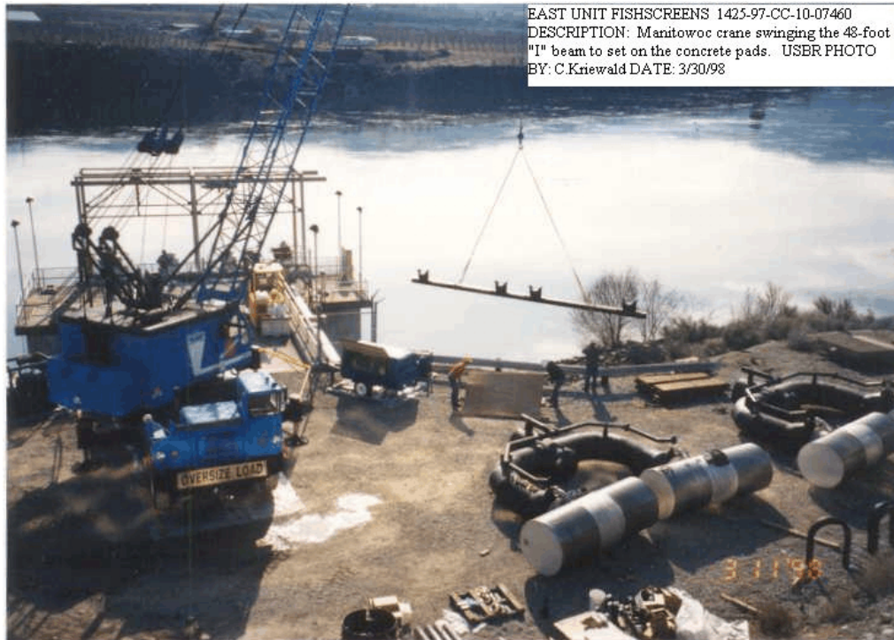
Figure 15.—Installation of cylindrical tee-screens at East Unit Pumping Plant, Washington.
