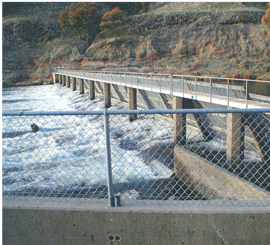
Figure 130.—Nimbus Dam bar rack barrier, American River, near Sacramento, California. (Nimbus Fish Hatchery).
