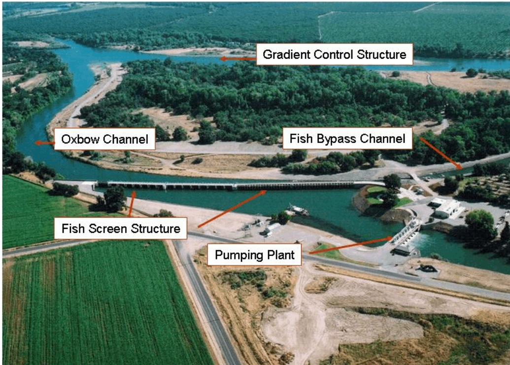
Figure 6.—Aerial view of GCID fish screen structure.
