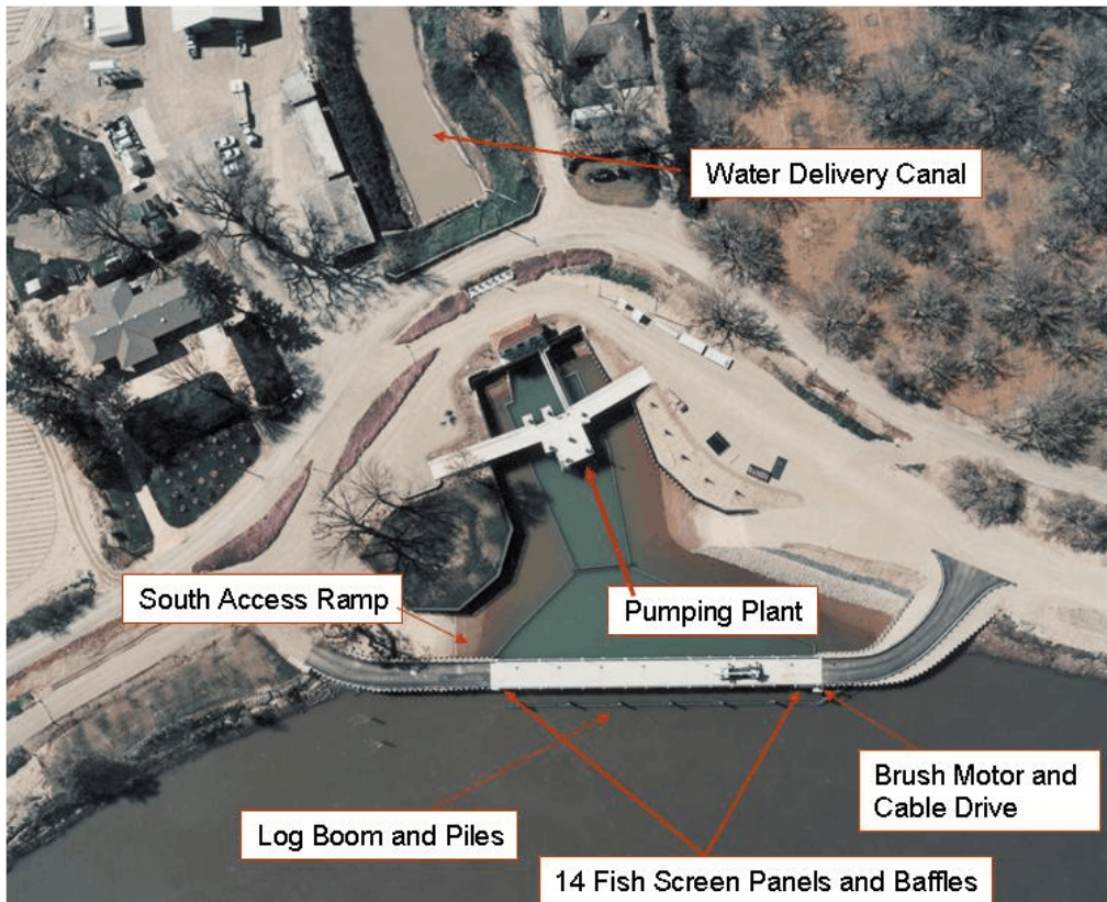
Figure 29.—Aerial photo of Wilkins Slough Fish Screens (RD-108).
