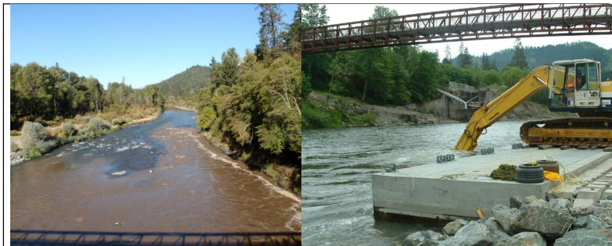
Figure 14. Downstream view of turbidity plume released from breaching of Savage Rapids Dam in Oregon (left photo), and temporary removal of sediment aggradation just downstream of dam at water intake.
