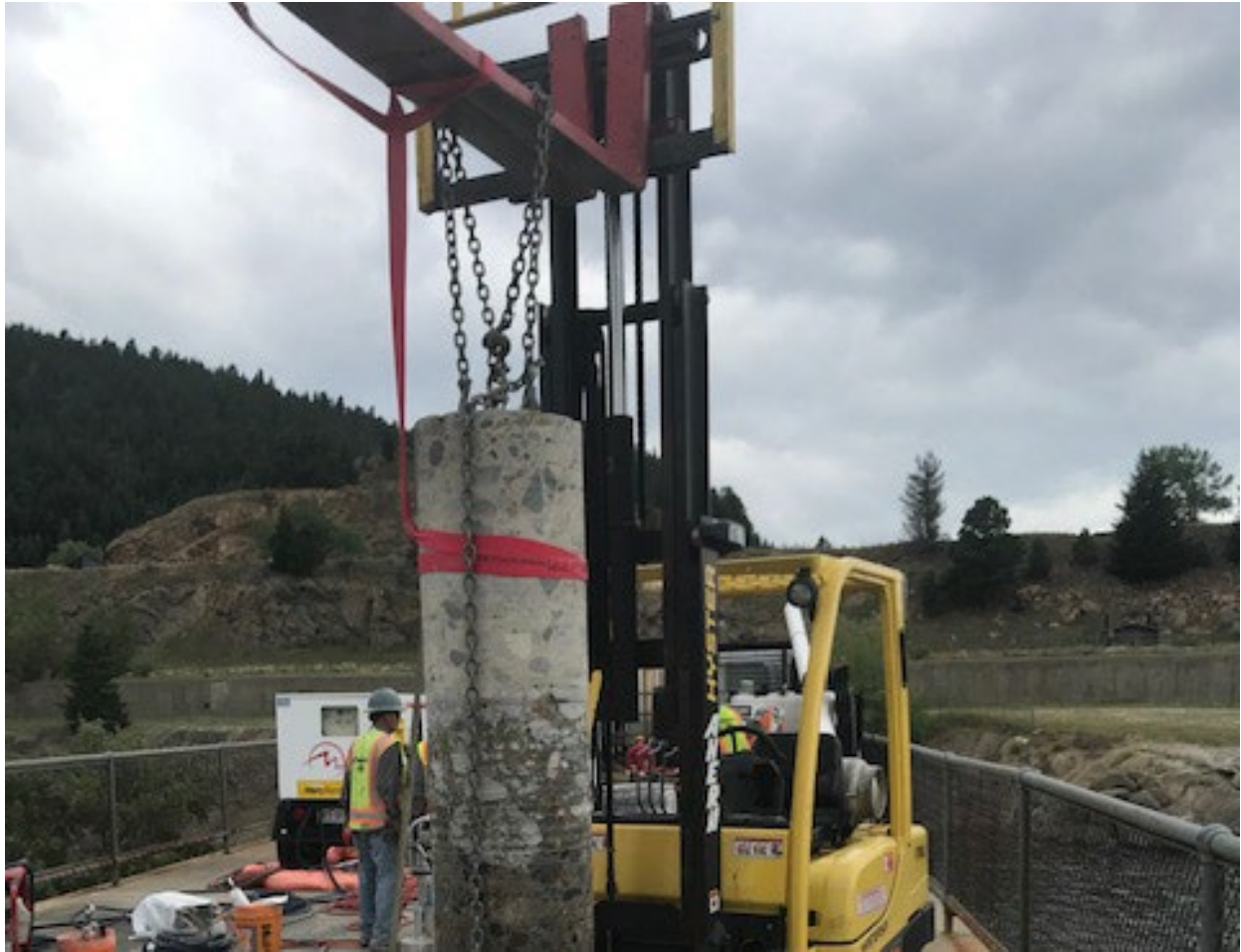
Figure 3. 18-inch concrete core lifted using anchors
