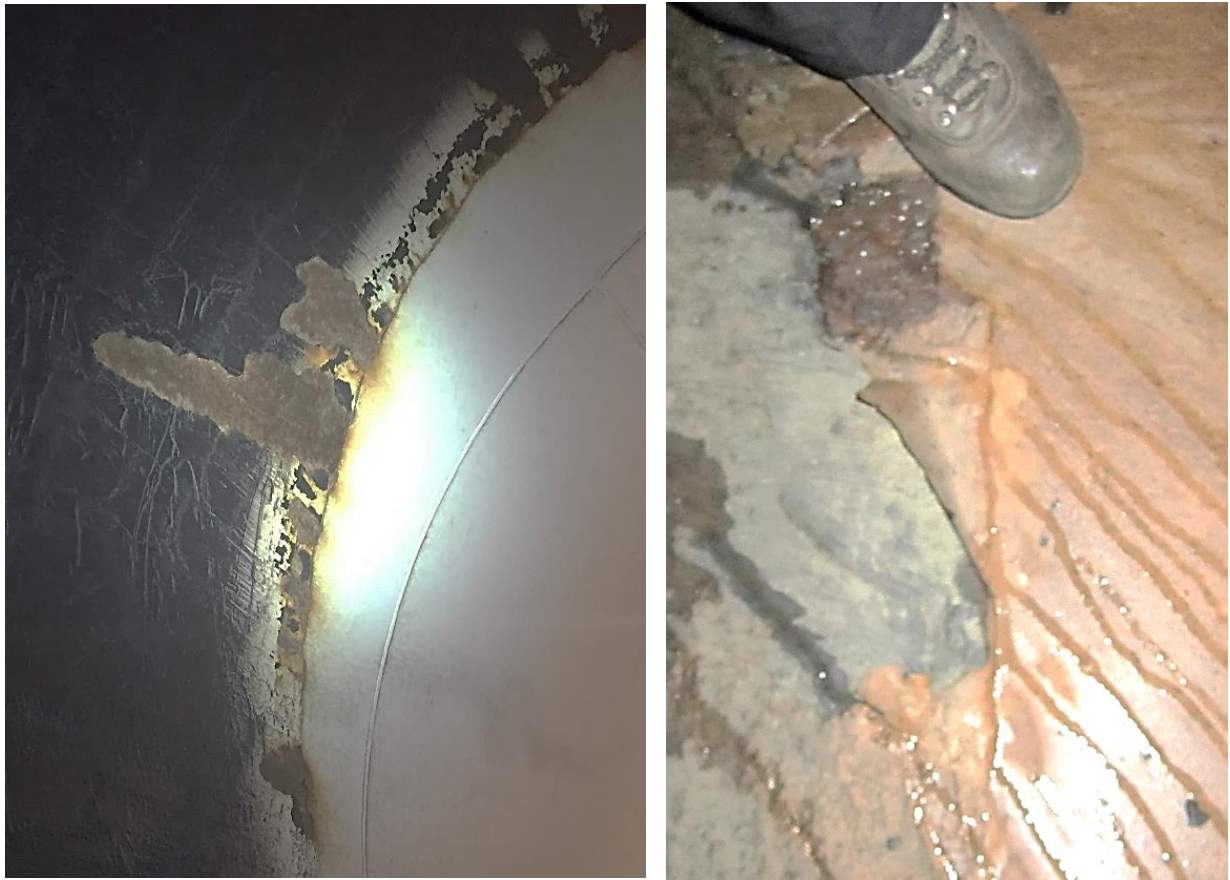
Figure 1-2. Photograph of Unit 12 discharge tube at Grand Coulee Keys Pump/Generator Plant. Left: Solvent-borne epoxy/coal tar enamel interface; some coal tar enamel has disbonded. Right: Solvent-borne epoxy disbondment at the interface, but no corrosion.
