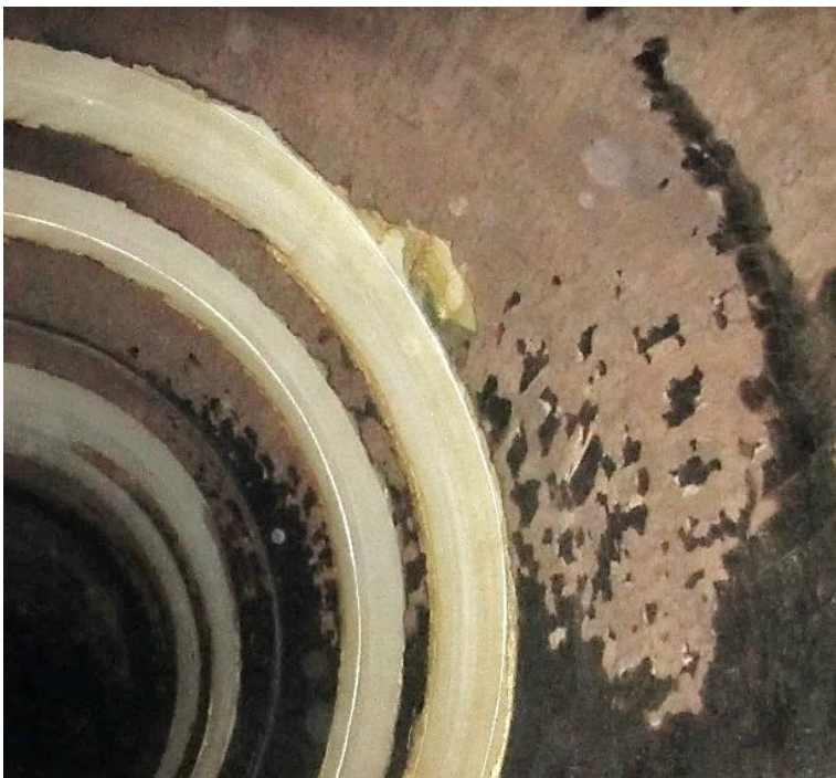
Figure 2. Coal tar enamel lined discharge tube showing badly degraded enamel in the pipe crown and several bands of spot repairs at Unit 6, Grand Coulee Keys Pump/Generator Plant. Photo taken in the above ground section, which is subjected to fluctuating temperatures.
