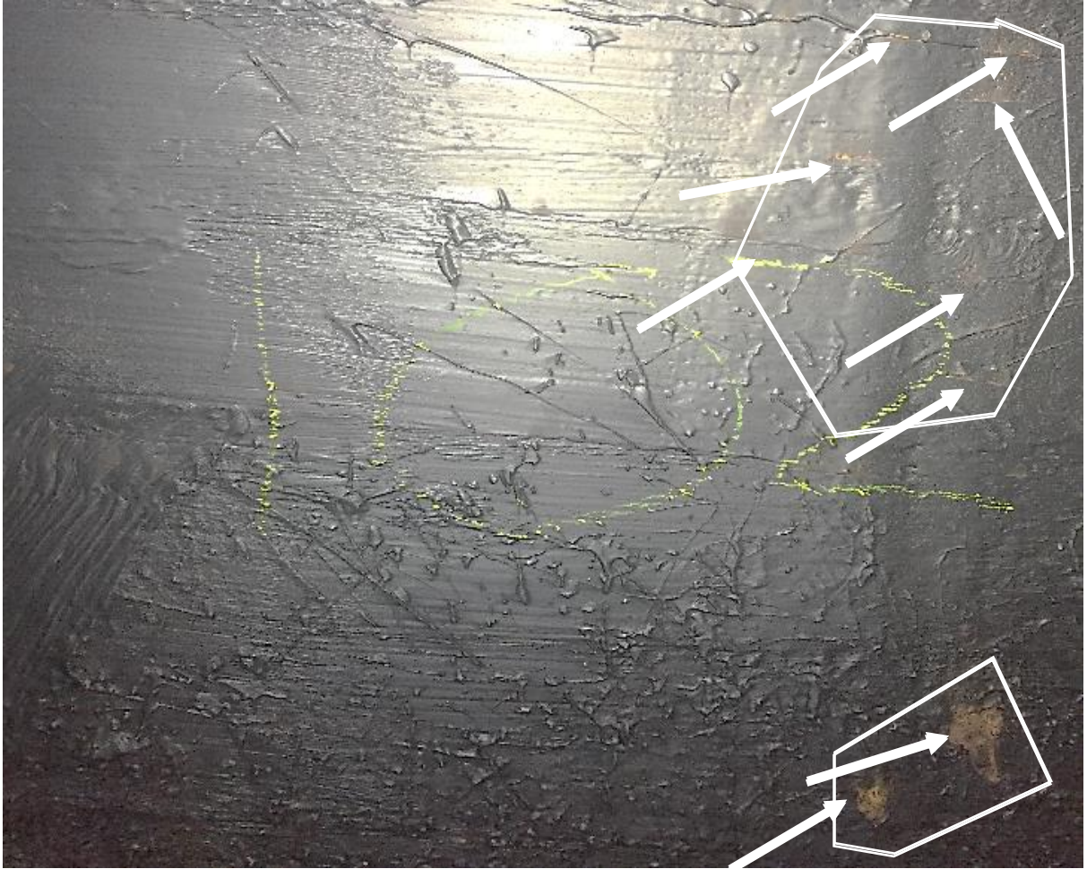
Figure 5. Areas selected for spot repair should be outlined to correct all defects, while preserving as much coal tar enamel as possible.
