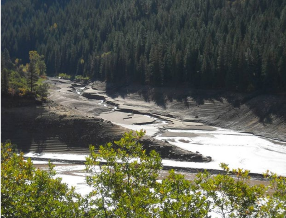
Figure 6. A photo of Paonia Reservoir in Colorado after the reservoir was drawn down: a channel incised through a portion of the reservoir sediments.
