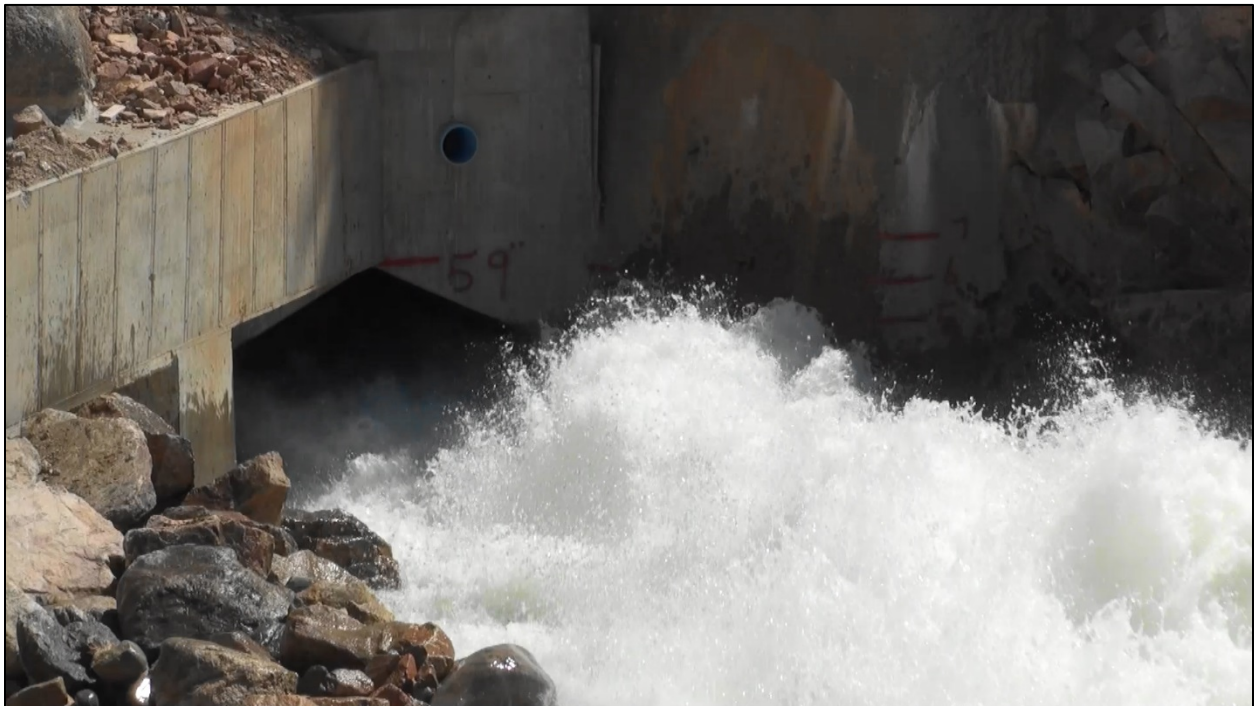
Figure 7 Discharge into stilling basin with hollow jet valve at 100 percent open. Flow is about 380 \text{ft}^3/\text{s} (flowing left to right).
