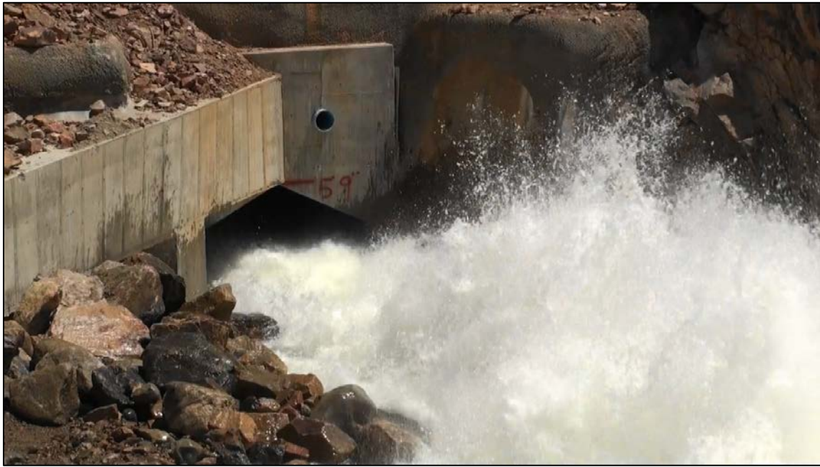
Figure 8 Discharge into stilling basin with both hollow jet valve and jet flow gate 100 percent open. Flow is greater than 430 ft 3 /s (flowing left to right).
