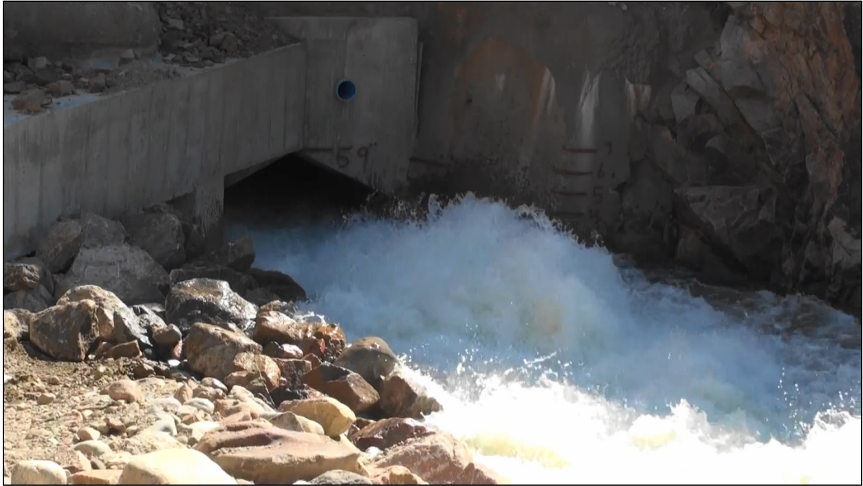
Figure 6 Discharge into stilling basin with the hollow jet valve at 50 percent open. Flow is about 220 \text{ft}^3/\text{s} (flowing left to right).
