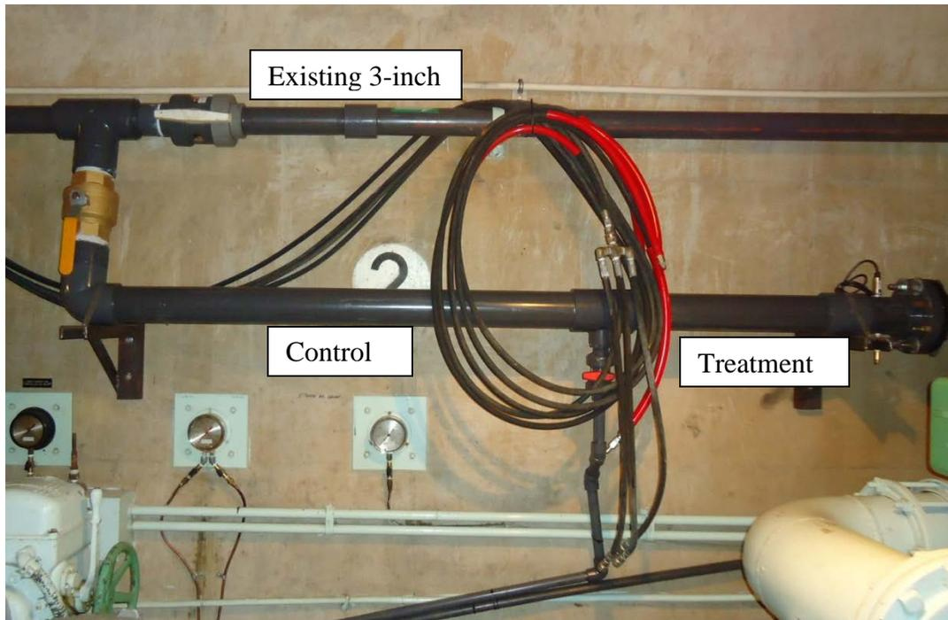
Figure 1 Test piping bypass on existing 3-inch cooling pipe.
