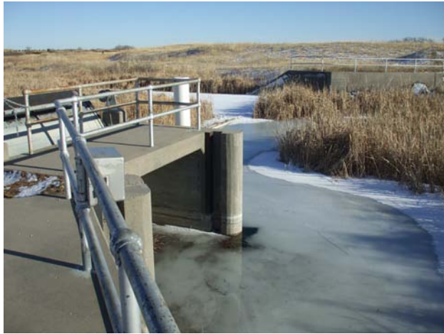
Figure 4. Dunlap Dam & bypass gate bay.
