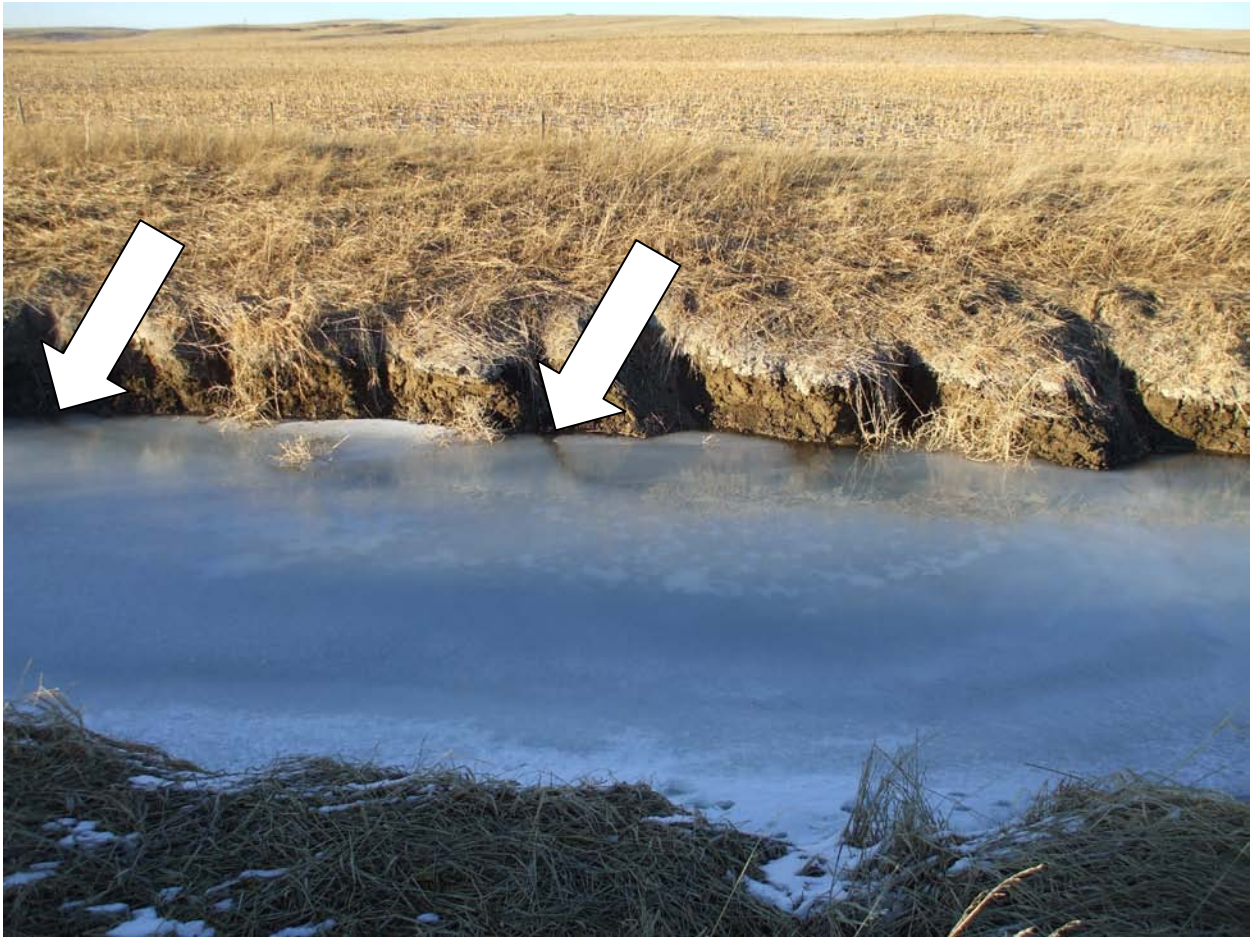
Figure 2. This photo of the MFID canal taken on 01/23/2012 shows patterns in the ice (arrows) that indicate the canal is functioning as a ground water interceptor at the time of the visit.
