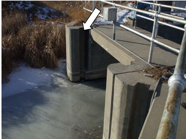
Figure 6. MFID canal heading gate bay
