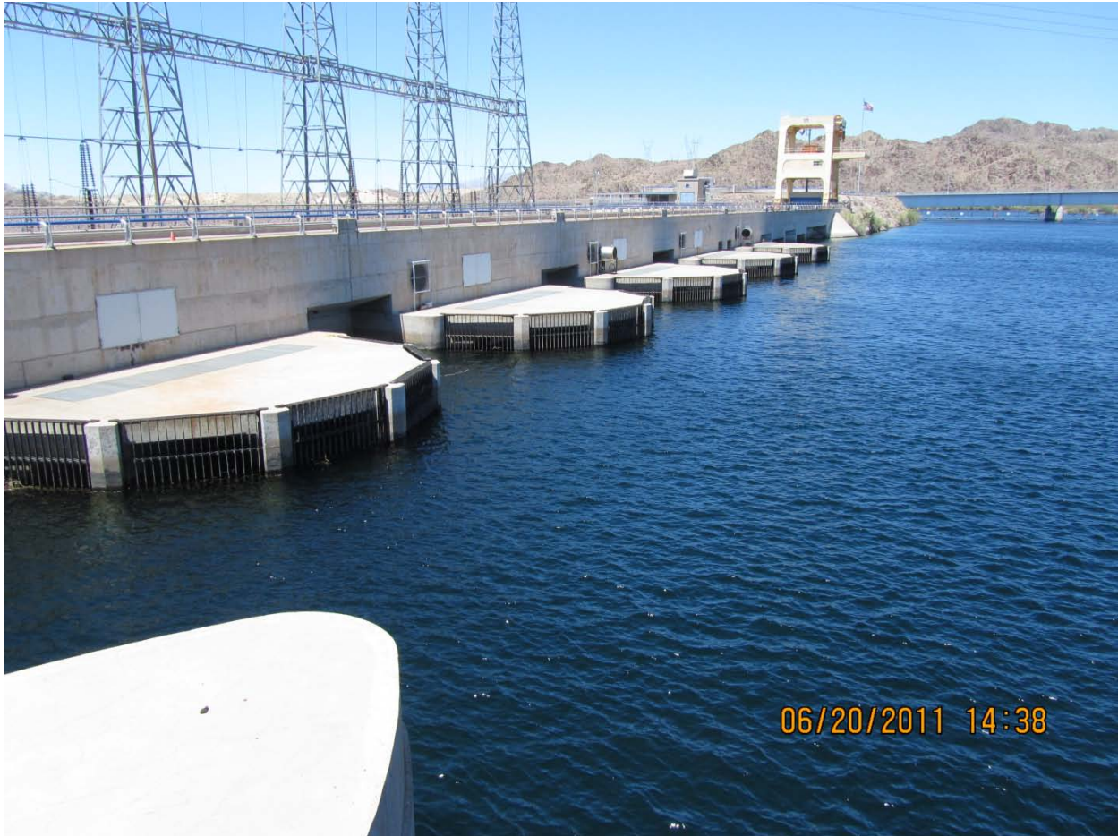
Figure 1 - All five penstock inlet trash rack structures at Davis Dam
