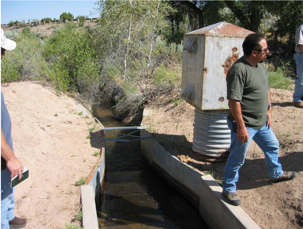
Figure 1—Parshall flume with stilling well and equipment shelter.
