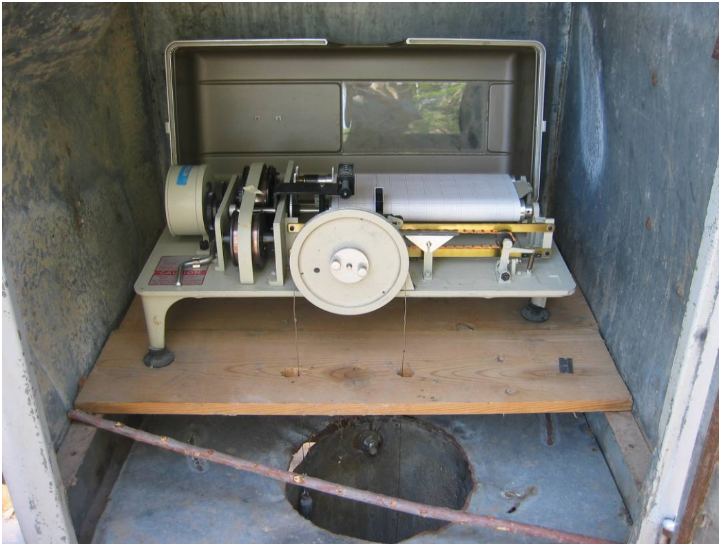
Figure 3—Stevens Recorder in equipment shelter atop a stilling well.
