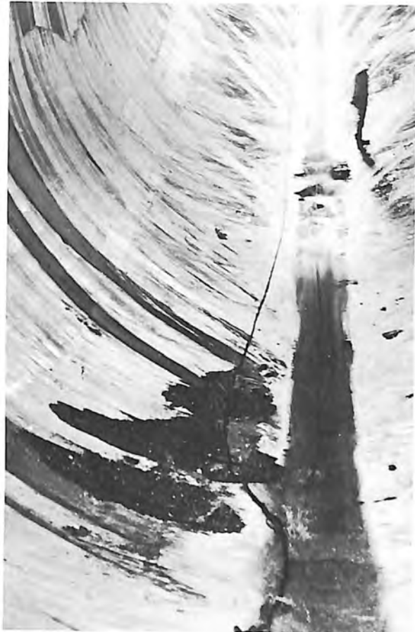
Figure 5. View looking upstream showing the two major damaged areas in the vertical bend. One area is in the left foreground, the other in the invert at the center of the photograph. Note man near the upper damage area. Photo P459-640-4088
