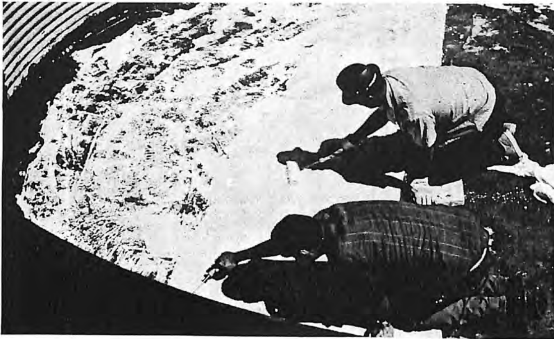
(a) Application of B-5800 to form a residual vinyl plastic film. The material was applied as a concentrated mixture, 3 parts B-5800 to 1 part water, in two equal applications at a total rate of 0.4 gsy ( 1.8 \text{ l/m}^2 ). Photo P800-D-68963
