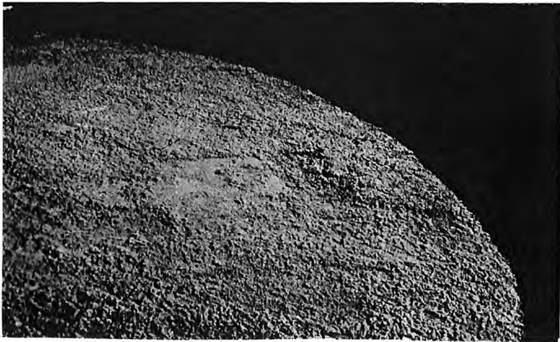
Photograph 6. Installation of soil sealants by mixed in-place treatment method.
