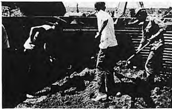
(a) Spreading soil in tank. Photo P800-D-68959
