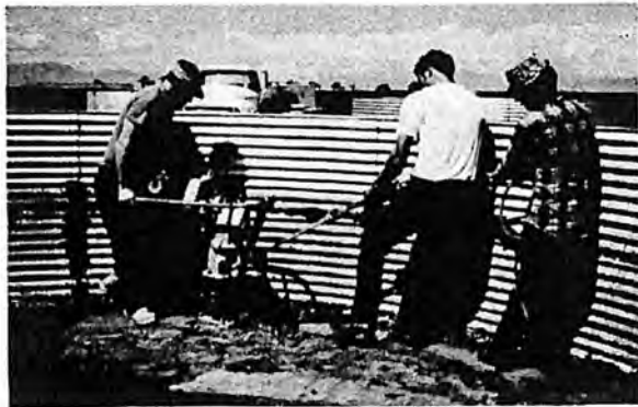
(b) Compacting soil in tank with a Wacker compactor. Photo P800-D-68960
