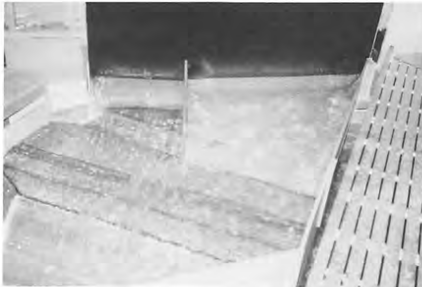
Figure 12. - The hydraulic jump in the existing spillway chute under PMF flow conditions.
