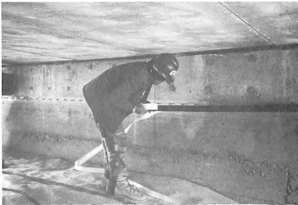
Photograph 22. — Stainless steel batten strips are used to attach geomembrane to bridge abutment.
