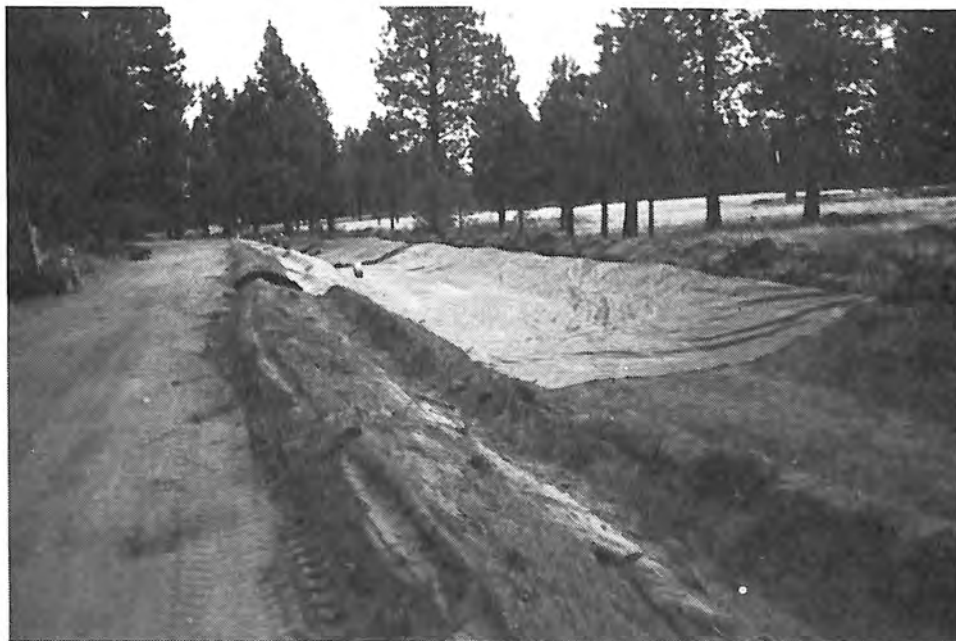
Photograph 36. — Second Terra-Tuff panel in place, ready for seaming.
