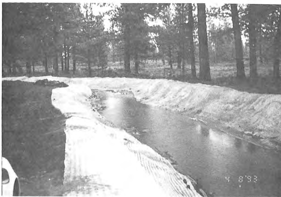
Photograph 62. — Completed canal section. Standing water covers exposed geomembrane.
