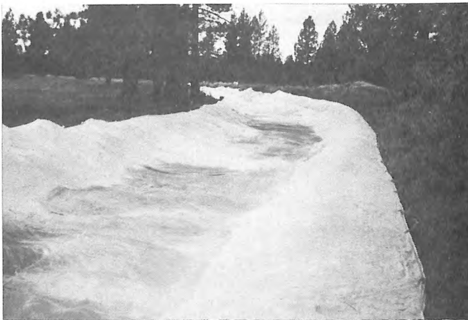
Photograph 44. — Grout mattress in place and ready for grouting. Note ties on right side used to hold grout mattress in place.
