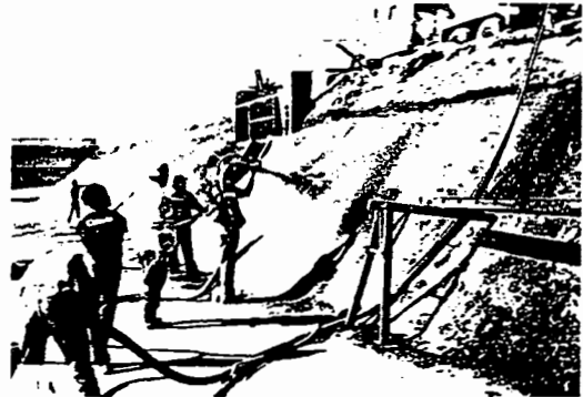
Arizona DOT Shotcrete Project Reinforced with Harbourite
