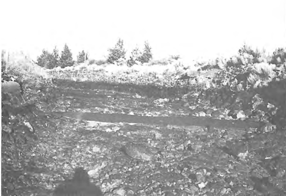
Photograph 7. — Section of canal with rock that can only be removed by blasting.
