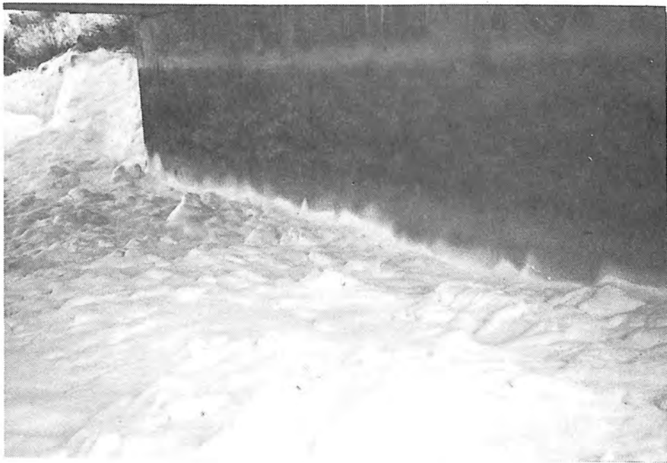
Photograph 66. — Foam bonds well to all surfaces, including this bridge abutment.
