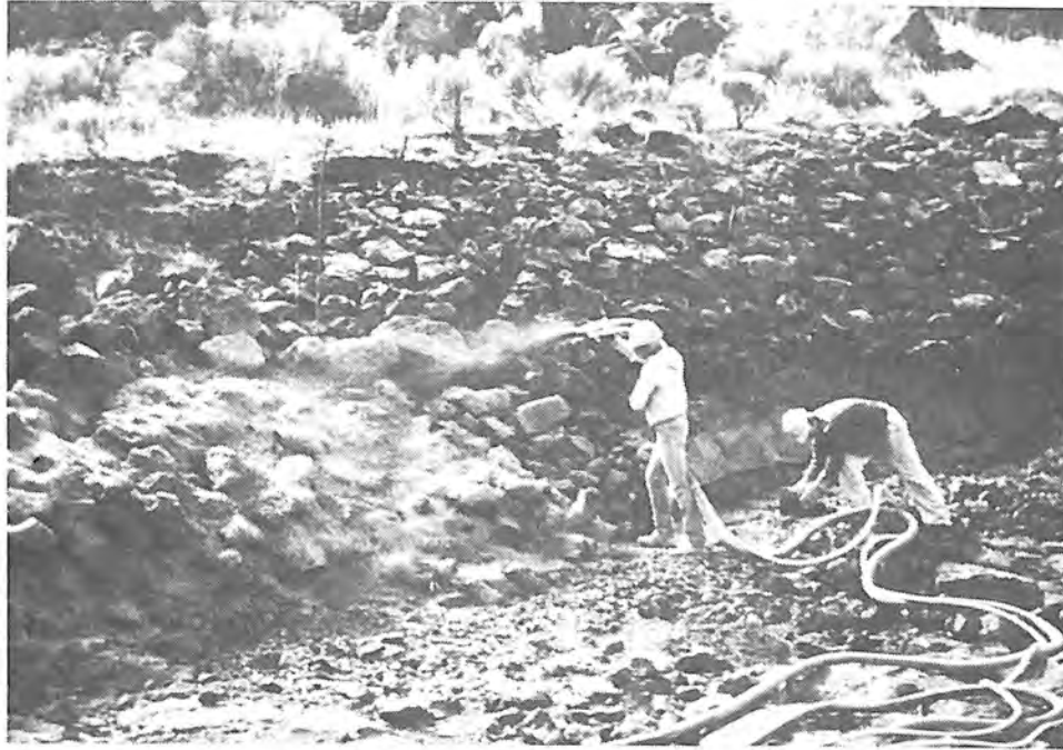
Photograph 91. — Nozzle man starts at top of canal and works his way to the bottom.
