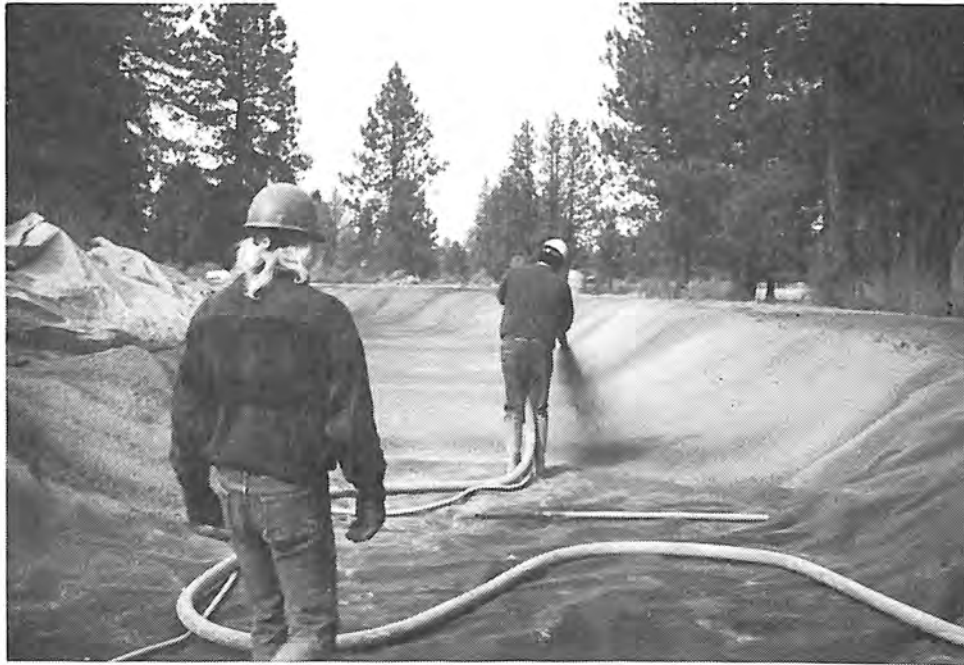
Photograph 17. — Shotcrete is applied over geomembrane.
