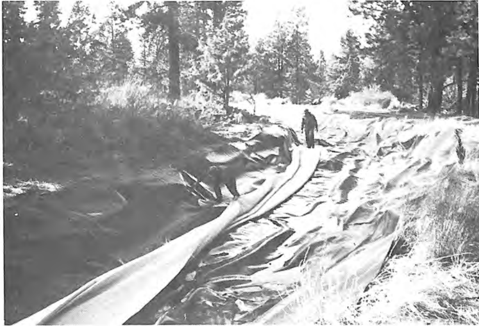
Photograph 59. — Grout mattress is placed in canal.
