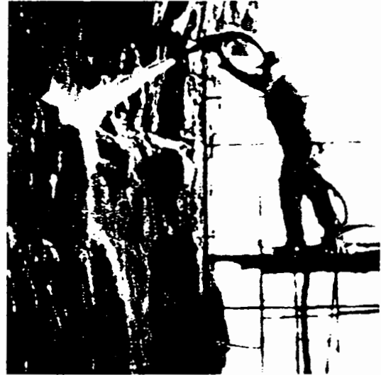
Shotcreting S/G Concrete on Quarry Wall
