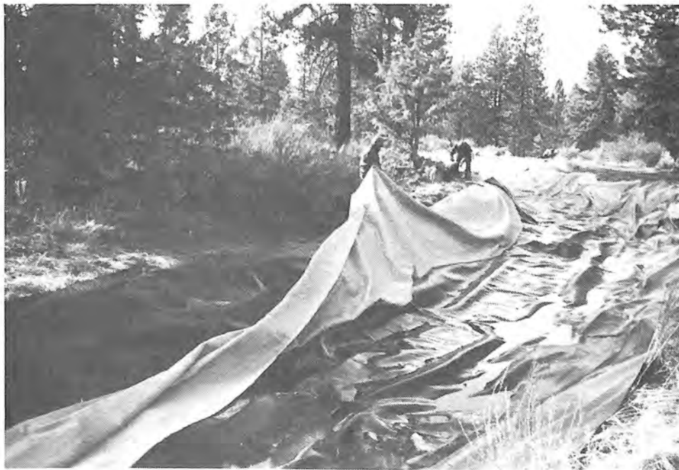
Photograph 60. — Mattress is pulled into place on side slopes. Geomembrane in canal bottom is left exposed.
