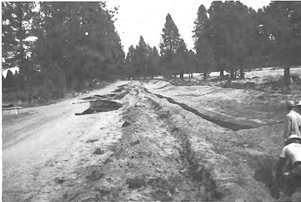
Photograph 35. — Prefabricated Terra-Tuff panel covers two-thirds of canal prism.
