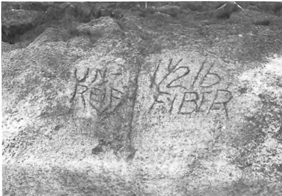
Photograph 106. — Contractor marked the locations of different weights of fiber reinforcement in the shotcrete.
