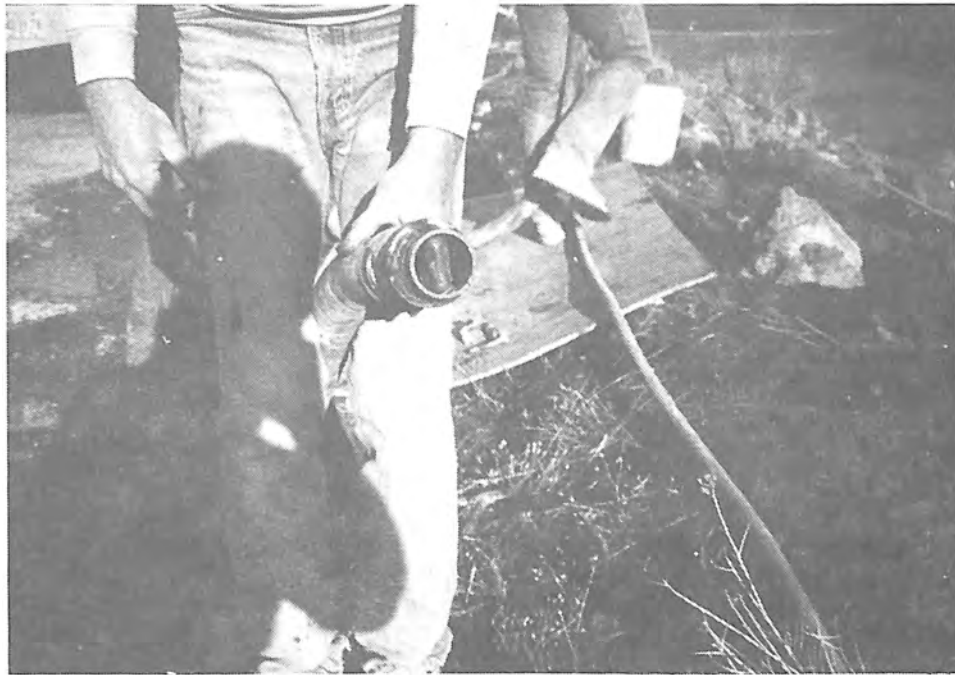
Photograph 89. — Shotcrete mix was specified as \frac{1}{2} inch minus aggregate. However, note 2\frac{1}{2} -inch rock wedged in the 2-inch hose.
