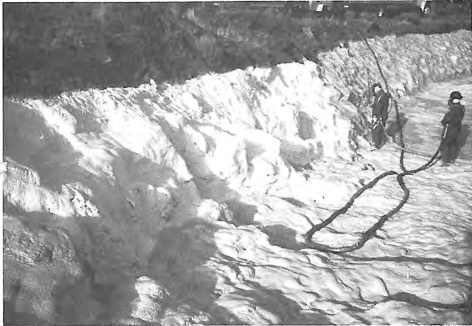
Photograph 67. — The lighter colored five-pound foam is applied over the darker 2-pound foam.
