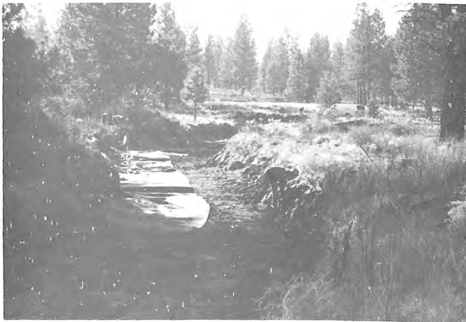
Photograph 54. — Geotextile is placed in canal to centerline. A second geotextile cushion will cover other half of the canal.
