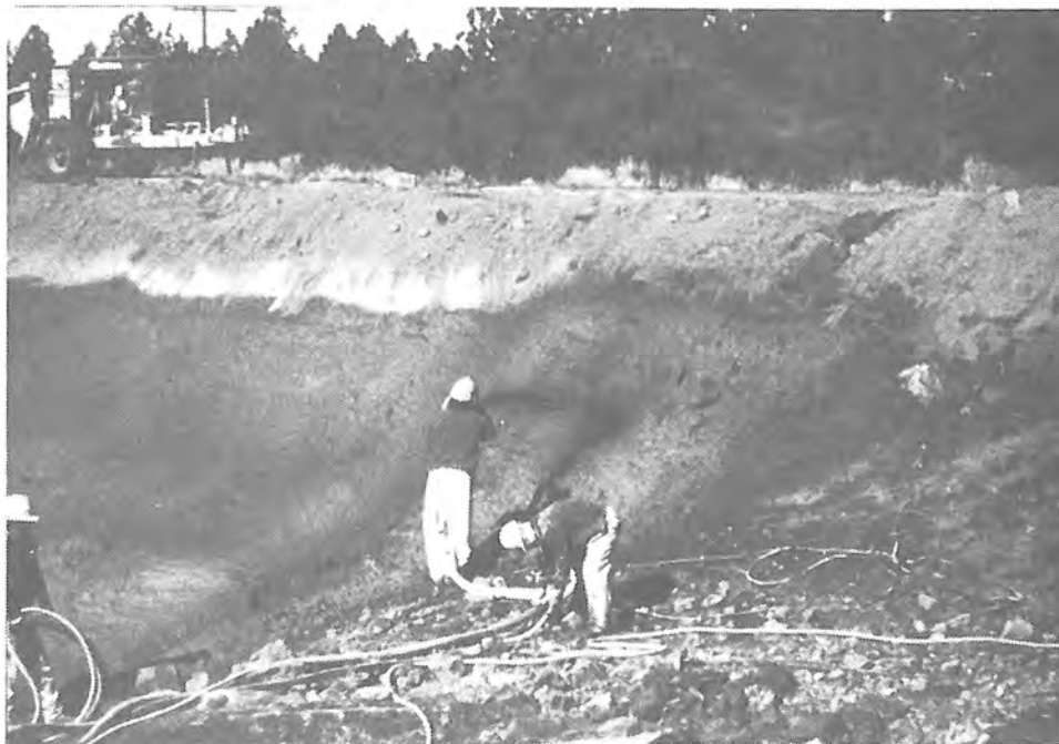
Photograph 90. — Shotcrete application.
