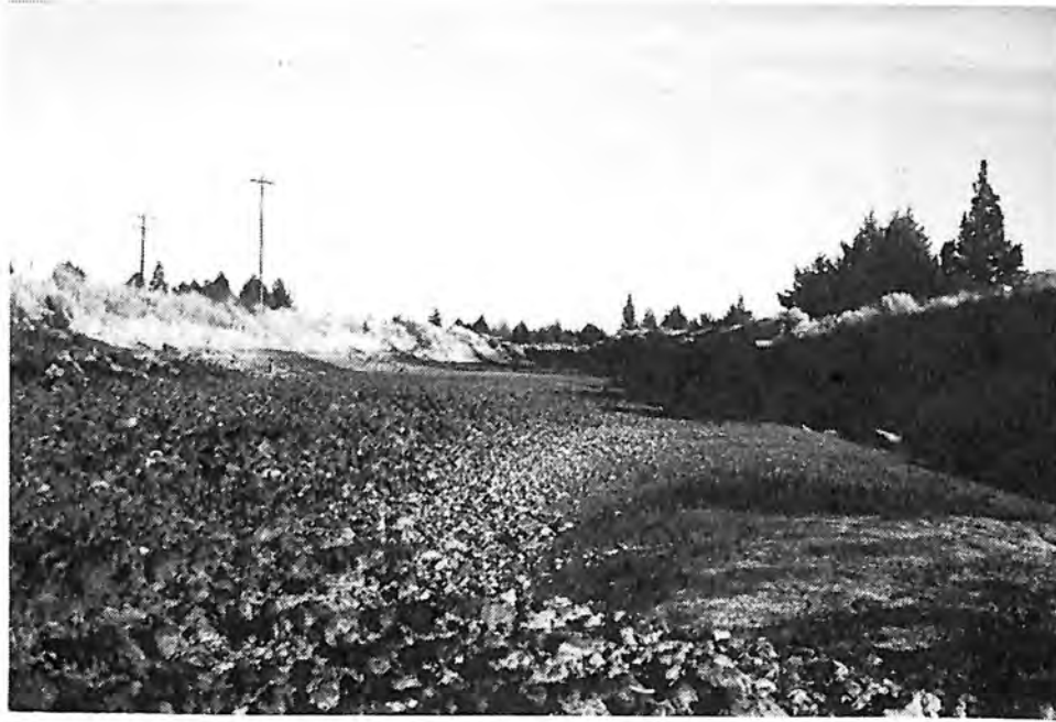
Photograph 5. — Section of canal with natural sediment deposits.
