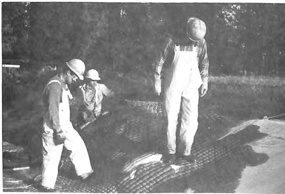
Photograph 46. — A five-man crew works the grout mix through the mattress.
