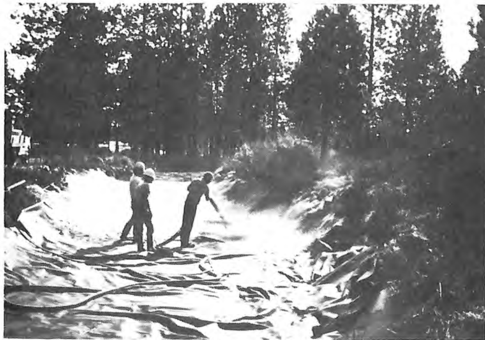
Photograph 10. — Shotcrete is applied over geomembrane.
