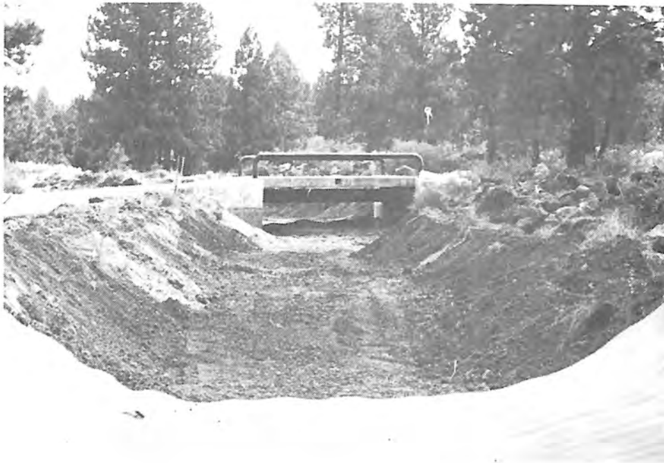
Photograph 19. — Completed canal preparation.
