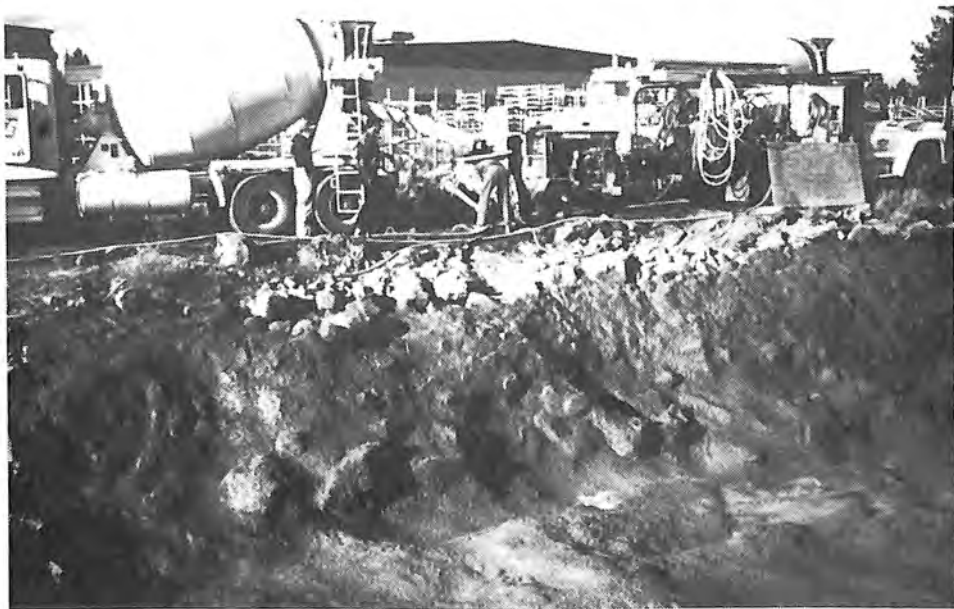
Photograph 86. — Concrete truck, grout pump, and air compressor are used for the shotcrete application.
