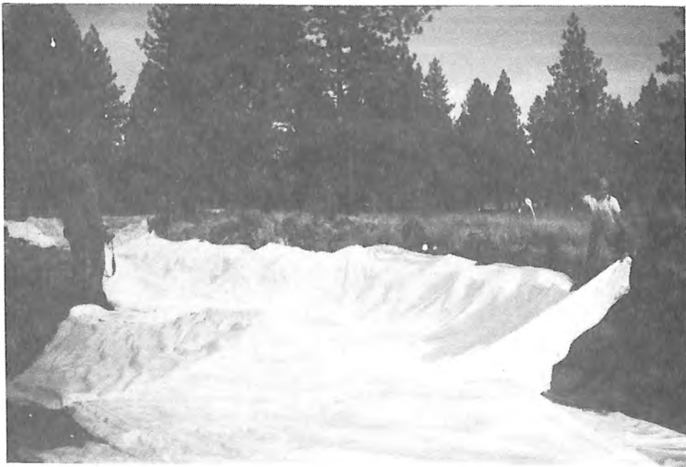
Photograph 42. — Mattress in place, ready for seaming (zipper).
