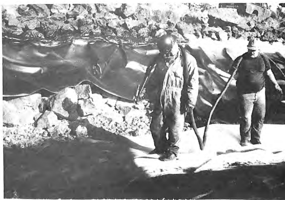
Photograph 78. — Coating is applied to geotextile.
