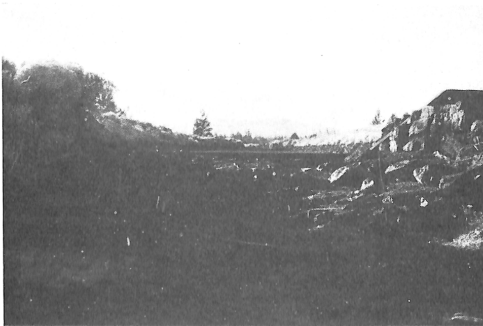
Photograph 8. — Section of canal with natural drop that creates high velocities.
