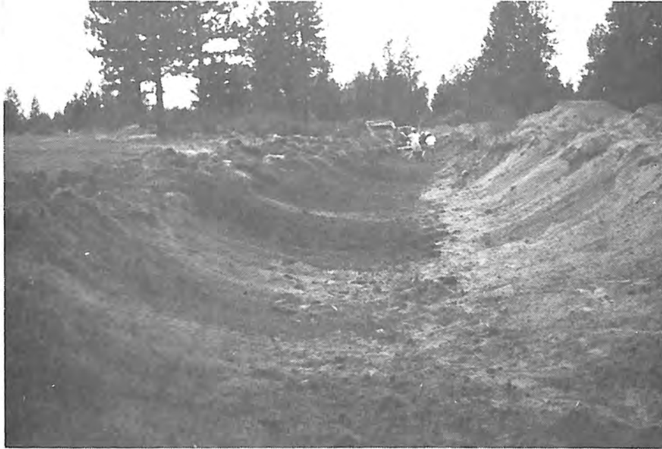
Photograph 27. — Canal prism is complete and ready for installation of geotextile and Geolam.
