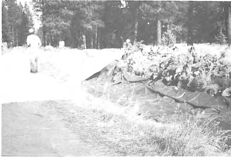
Photograph 41. — Worker places grout mattress cover in canal bottom over PVC geomembrane.
