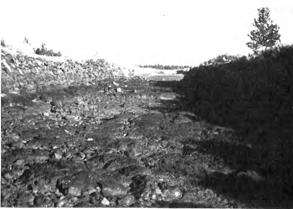
Photograph 6. — Section of canal with fractured rock.
