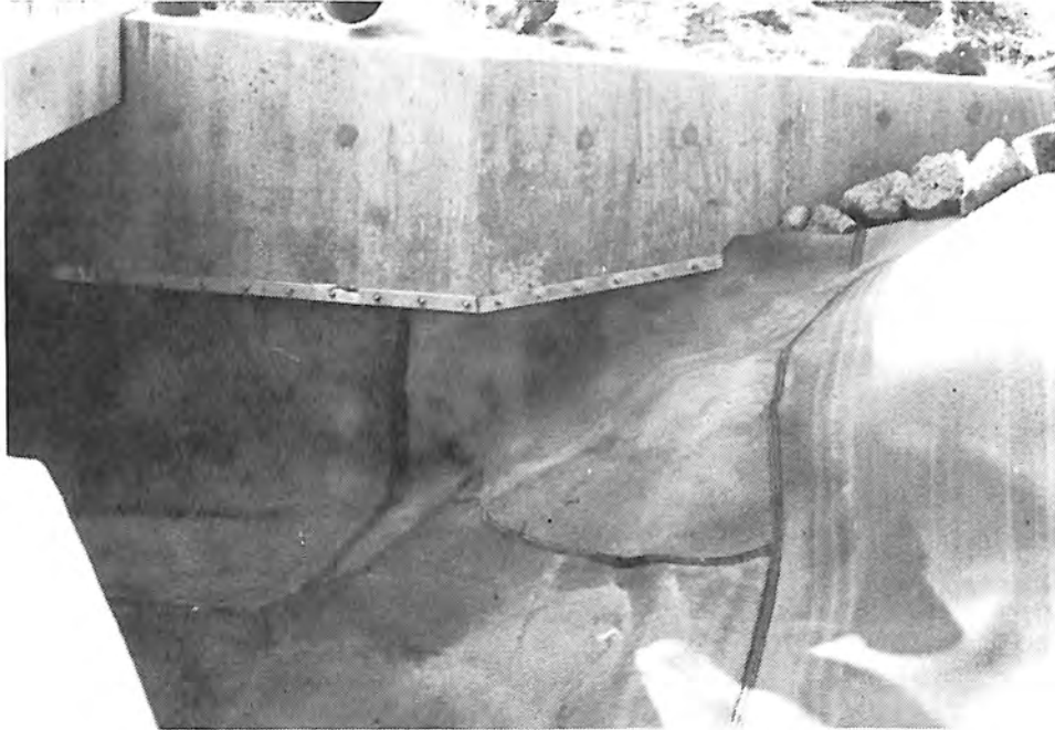
Photograph 23. — Completed seaming and attachment to bridge.
