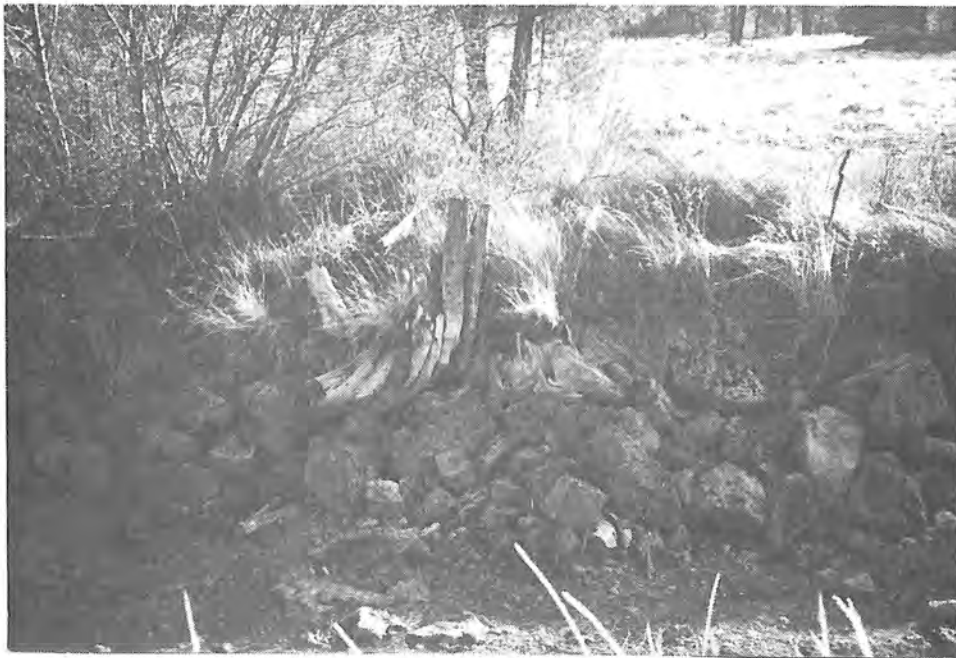
Photograph 2. — Sections of canal with rock and stumps requiring removal.
