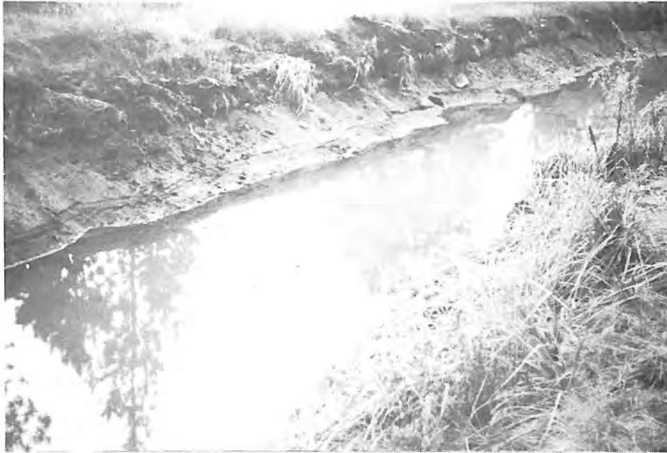
Photograph 39. — Completed canal subgrade after removal of overhang on canal side slope. Note standing water in canal.
