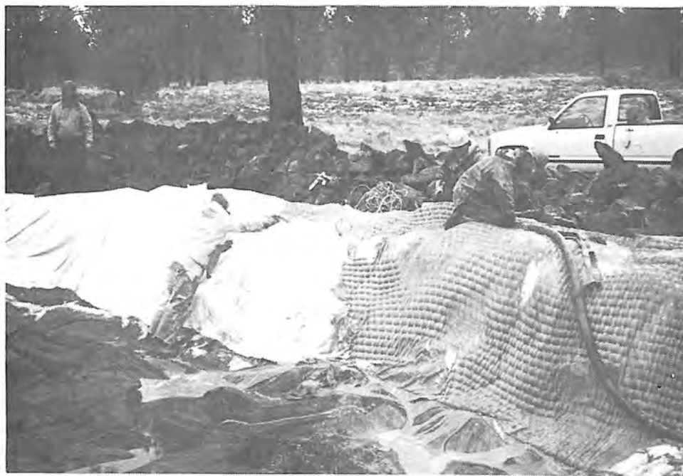
Photograph 61. — Grout is pumped into mattress.
