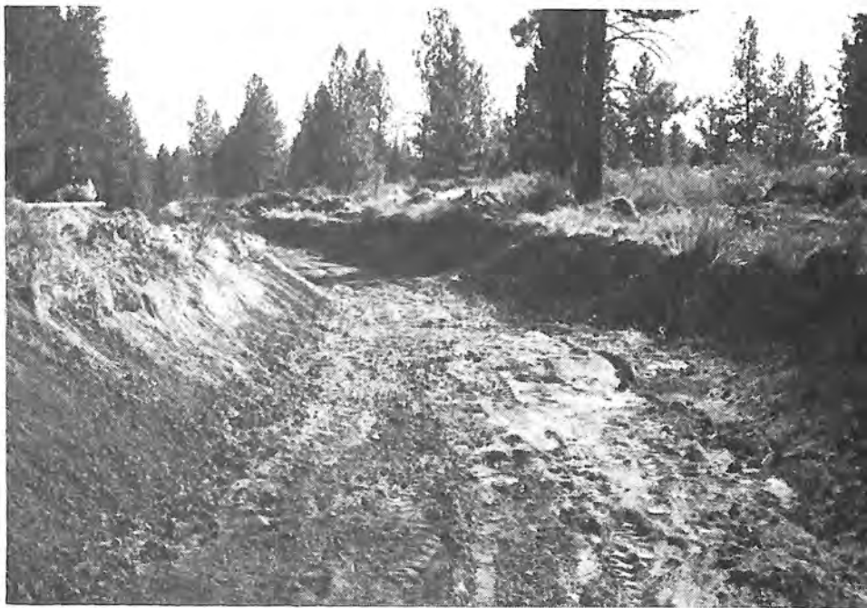
Photograph 14. — Completed subgrade preparation.
