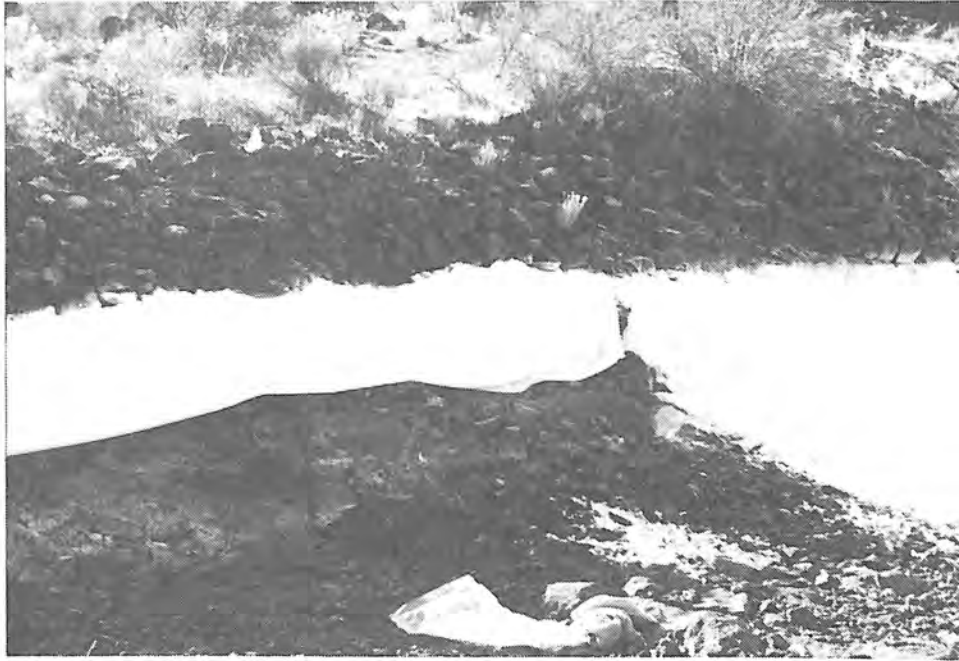
Photograph 73. — The 4-foot-wide geotextile is anchored above the water line.
