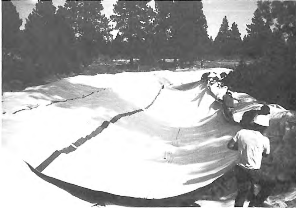
Photograph 29. — Inverted Geolam is placed over geotextile cushion.
