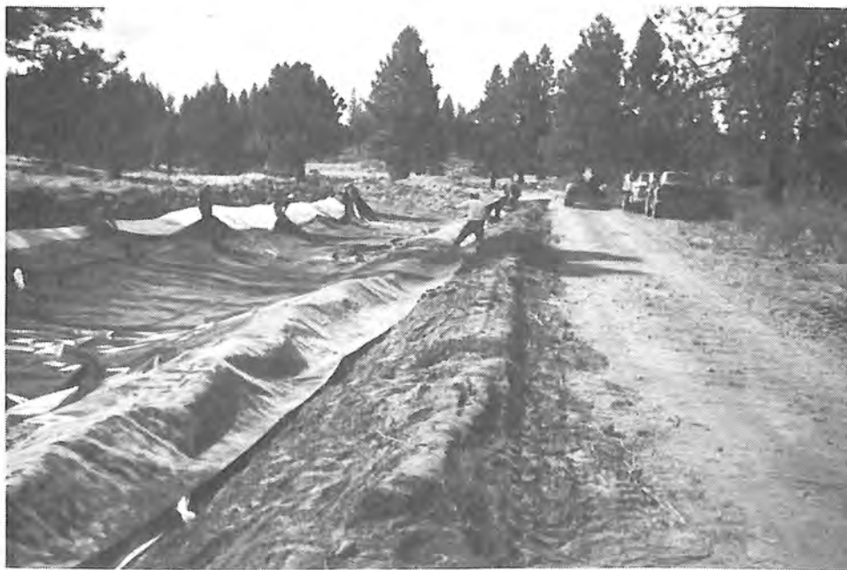
Photograph 32. — Ten-man crew installs geomembrane.
