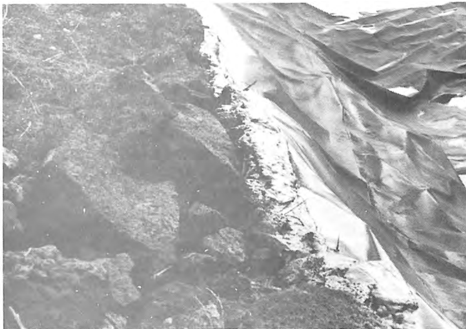
Photograph 79. — View of the side slope and the geotextile anchored with spray-in-place foam.
