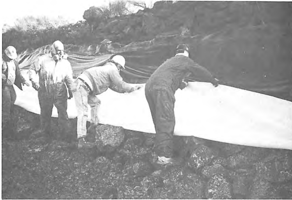
Photograph 75. — Second roll of textile is placed into fresh coating.
