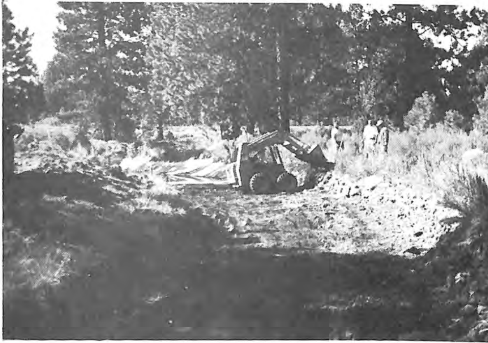
Photograph 13. — Bobcat is used to prepare subgrade side slopes.
