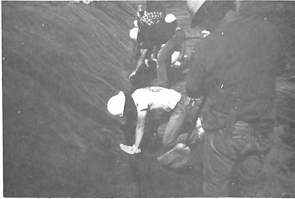
Photograph 37. — Crew joins Terra-Tuff panels using solvent seaming process.
