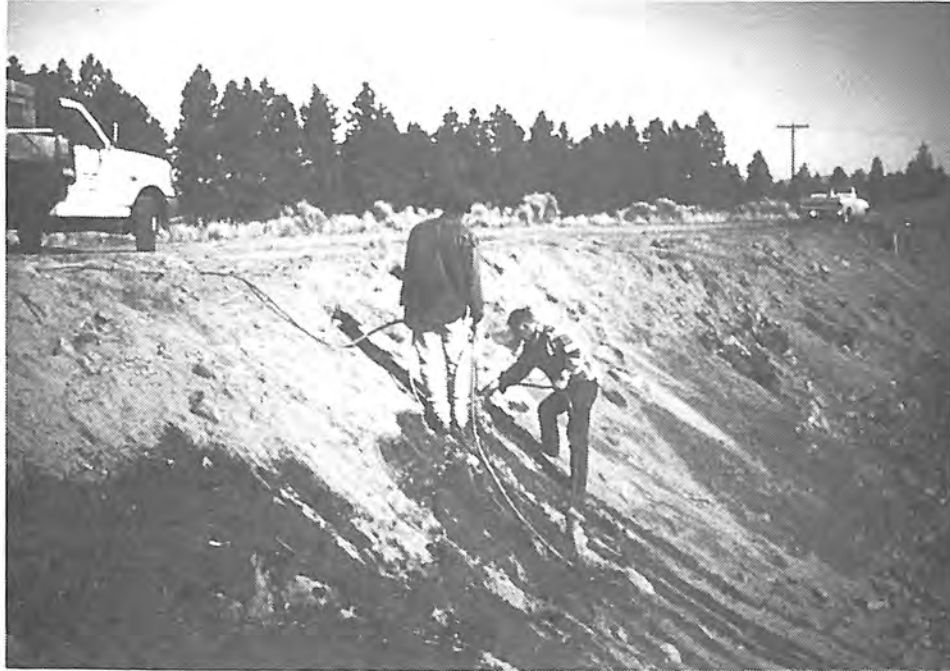
Photograph 83. — Fill material was used to fill in large voids on side slopes. This procedure was soon discontinued because available fill material proved unsuitable.
