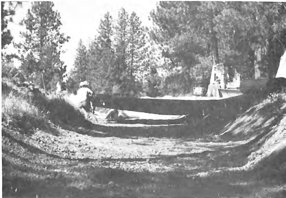
Photograph 20. — Five-man crew installs geomembrane.
