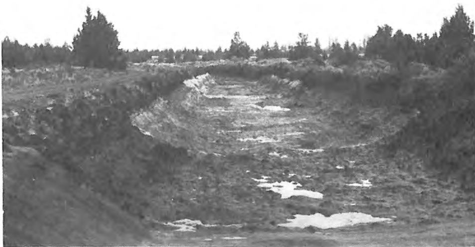
Photograph 82. — Completed canal sections (900 feet) with the Geothane 5020 coating.
