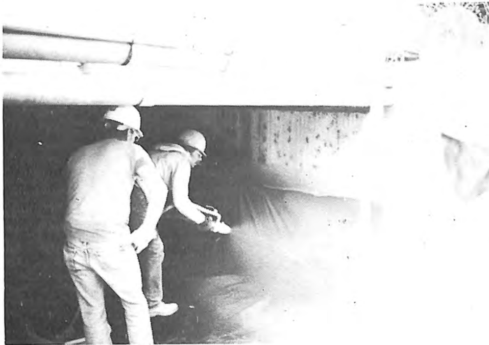
Photograph 11. — Shotcrete is applied to bridge abutment over MB II material.
