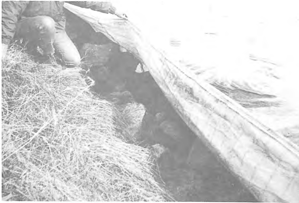
Photograph 49. — After only minimal subgrade preparation, the mattress is laid directly over the rocky side slopes.
