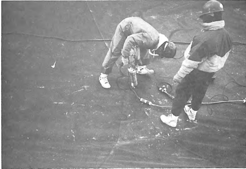
Photograph 21. — Geomembrane is repaired with a rounded patch and extrusion weld.
