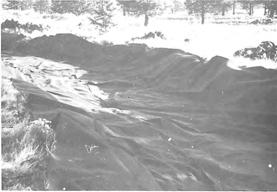
Photograph 55. — Completed geotextile cushion installation.
