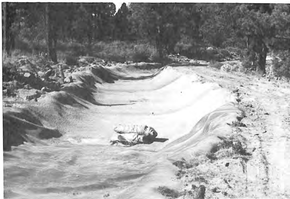
Photograph 18. — Completed canal section in background. Geomembrane awaiting shotcrete cover in foreground.
