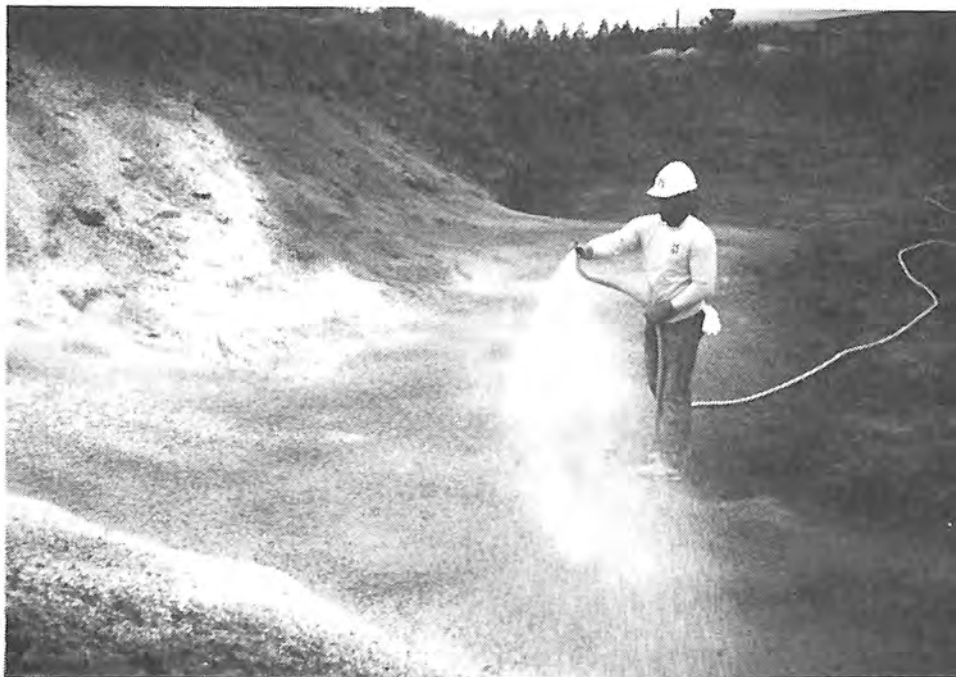
Photograph 94. — Curing compound applied to fresh shotcrete.
