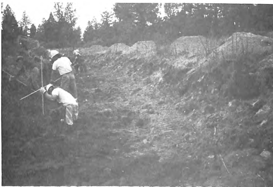
Photograph 25. — Ten-man crew smooths canal bottom. Imported subgrade material is shown on right.
