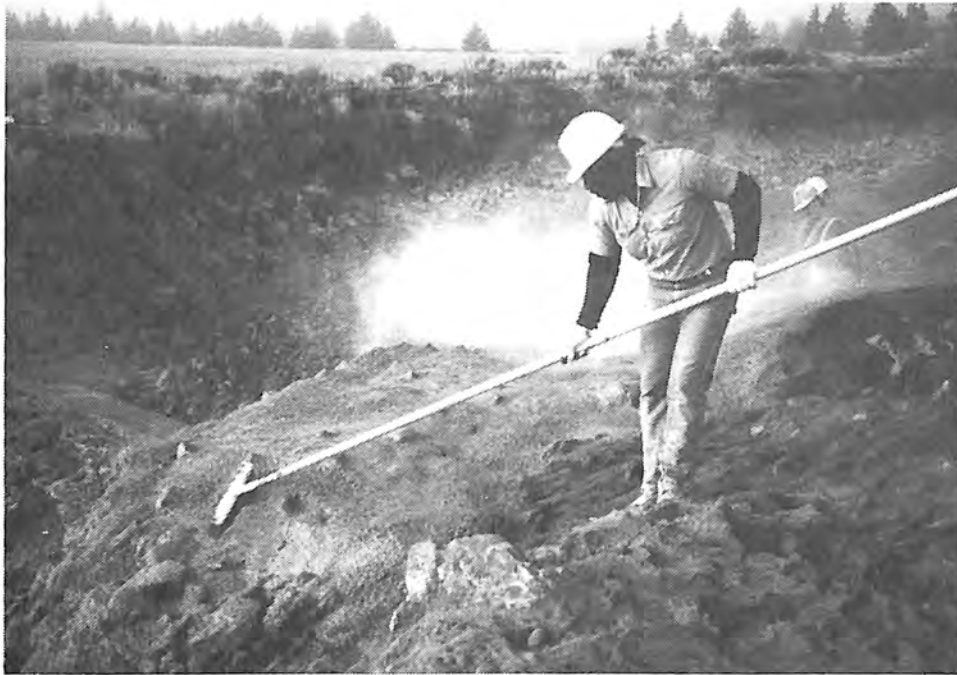
Photograph 93. — Contractor attempted to smooth out rough finish. This procedure was abandoned and shotcrete was left with "as shot" finish.
