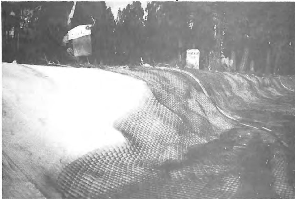
Photograph 52. — Mattress conforms to irregular subgrade.
