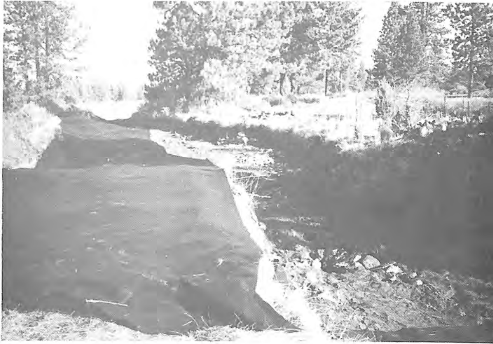
Photograph 53. — Geotextile cushion is laid out along road, ready to be placed in canal.
