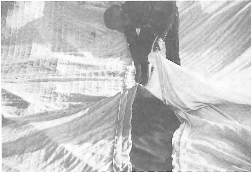
Photograph 43. — The mattress panels, sized to the canal in the factory, are zipped together (seamed).
