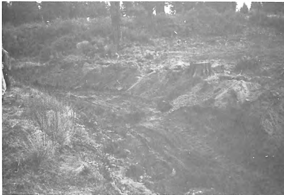
Photograph 25. — Canal is ready for final smoothing by hand raking. Tree stump on right bank was outside the canal prism and was left in place.
