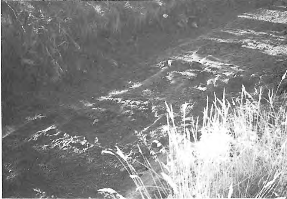
Photograph 3. — Section of canal with loose overhangs that need removal.
