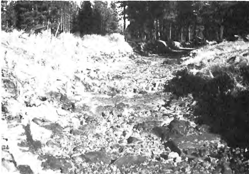
Photograph 4. — Section of canal with fractured rock.
