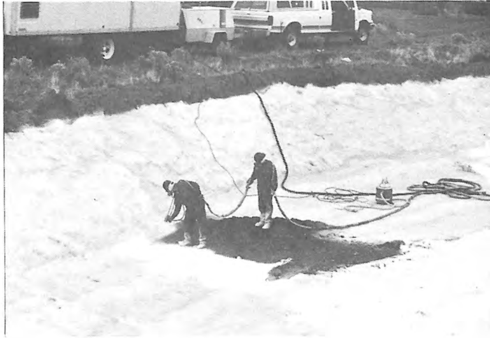
Photograph 63. — Two-pound density foam is applied directly to subgrade.
