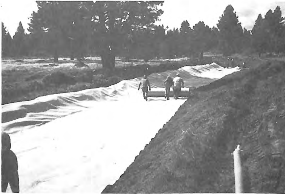
Photograph 31. — Crew installs geotextile on canal bottom and side slopes.
