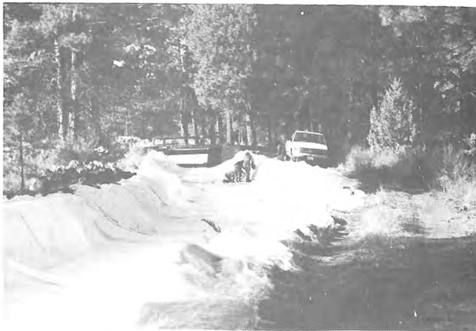
Photograph 50. — Final preparation work before grout is pumped into mattress.
