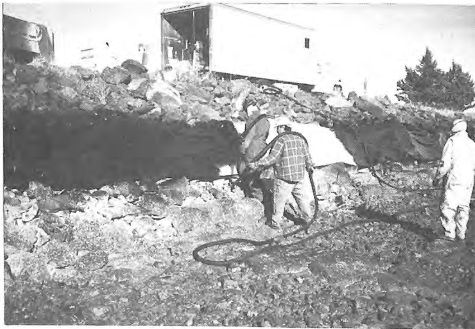
Photograph 74. — Coating is spray-applied over geotextile.
