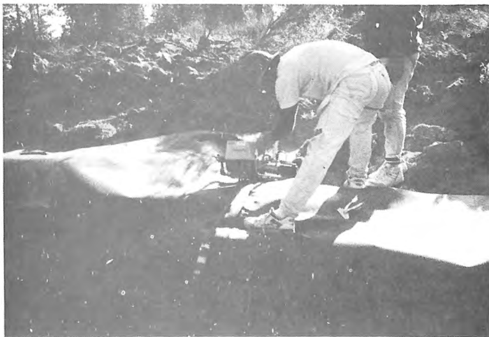
Photograph 16. — Geomembrane is seamed with hot-wedge welder.
