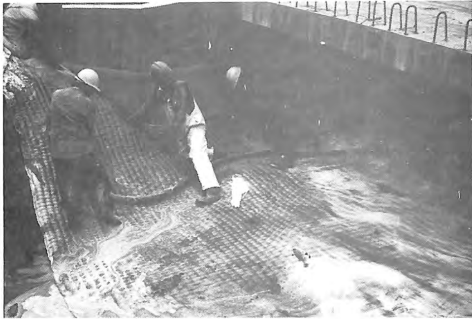
Photograph 51. — Grout is worked around a bridge abutment.
