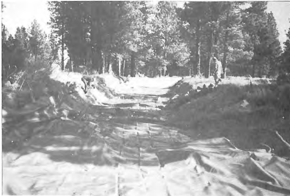
Photograph 40. — 40-mil PVC membrane in place, ready for grout mattress.
