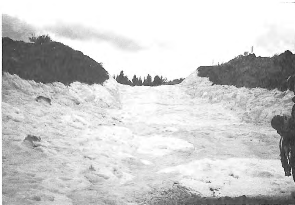
Photograph 64. — Completed application of 2-pound density foam.
