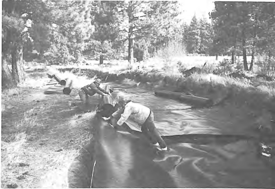
Photograph 57. — Membrane material is rolled across canal and up side slopes.
