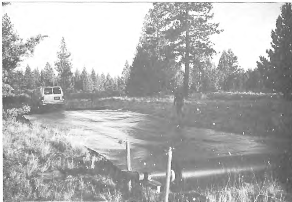
Photograph 56. — Geomembrane is rolled out and cut to fit canal prism.
