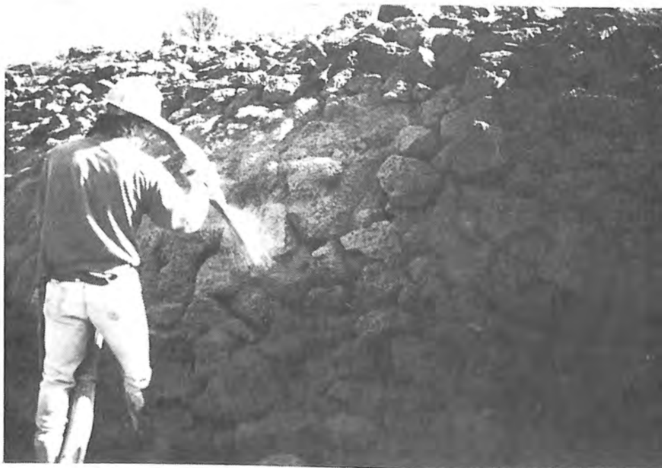
Photograph 92. — Close-up of grout being forced into voids.
