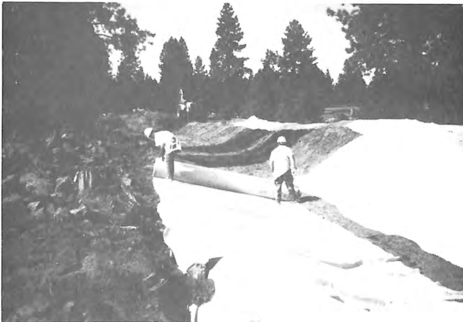
Photograph 28. — Geotextile is laid on canal bottom and side slopes.
