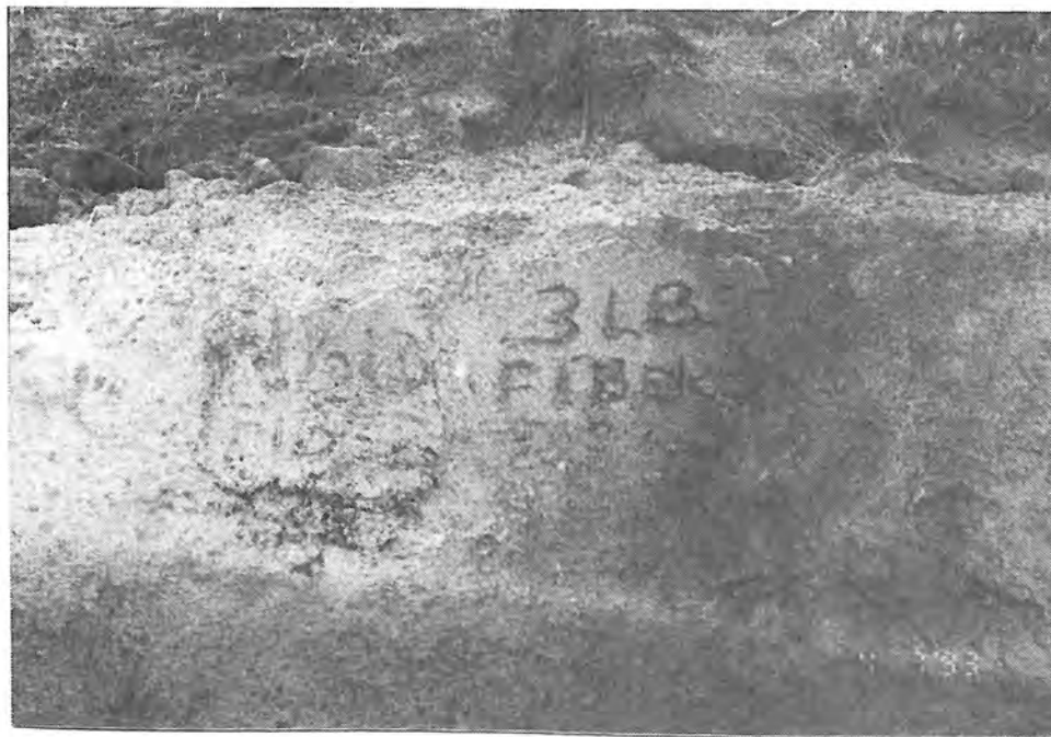
Photograph 104. — Contractor marked the locations of different fiber dosage in the shotcrete.
