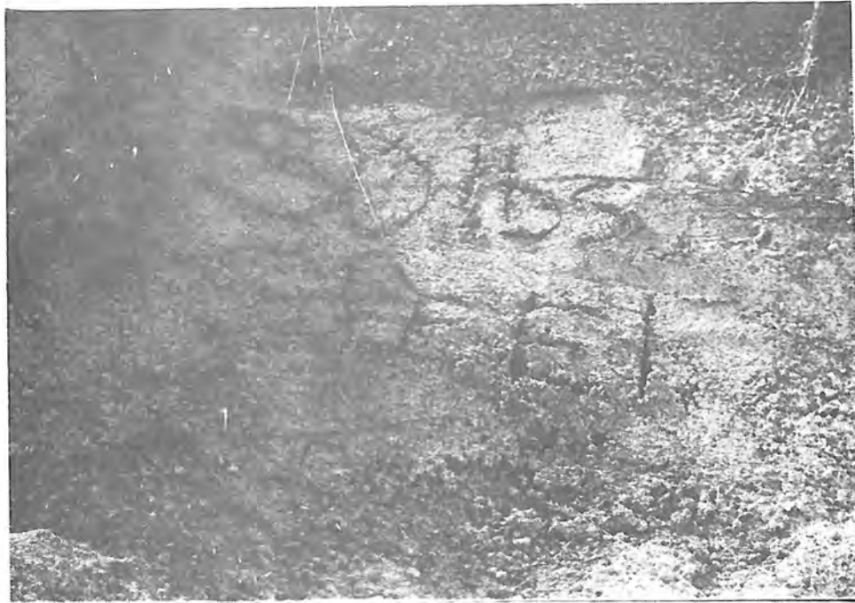
Photograph 97. — Contractor marked location of different fiber material sections in shotcrete.
