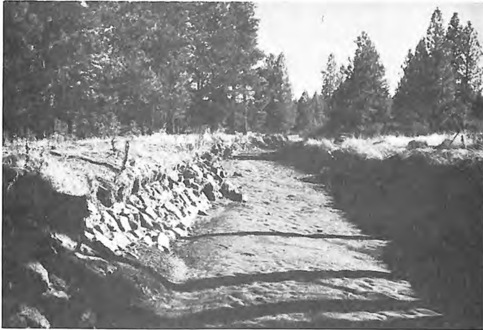
Photograph 1. — Section of canal with natural sediment deposits and rock side slopes.
