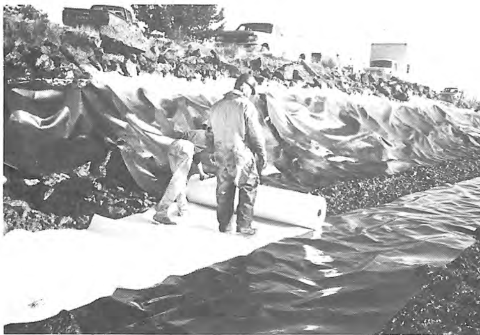
Photograph 77. — Geotextile is rolled into place.
