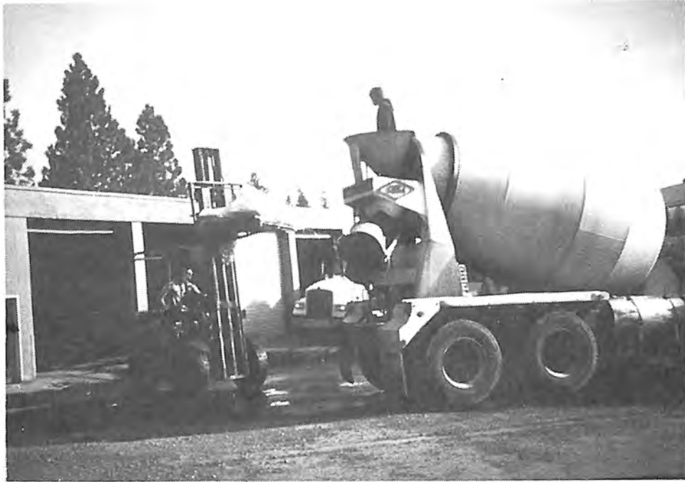
Photograph 85. — Fibers were added to the grout mix at the plant.
