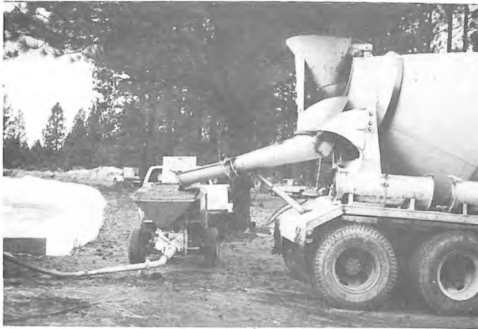
Photograph 45. — Grout mix is transferred to grout pump.
