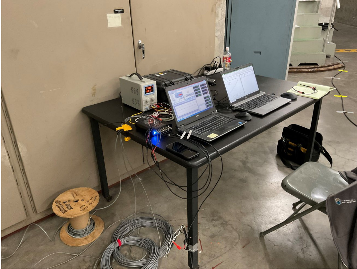
Figure 9. Data Acquisition setup used for WK testing for units G24 and G20.
