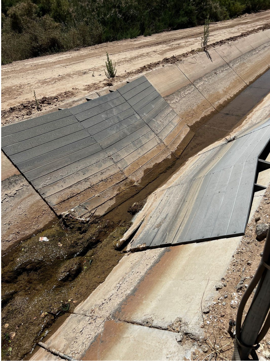
Figure 8. Pima canal flume pictured during a site visit in 2022.
