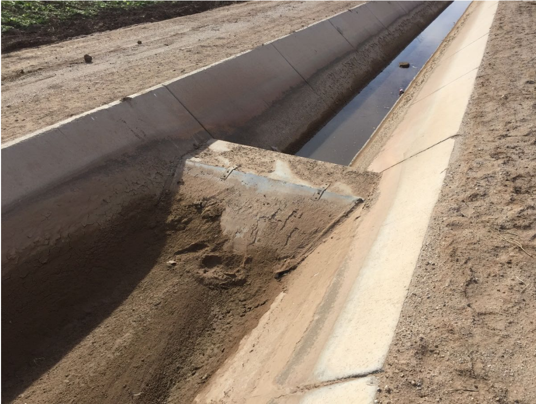
Figure 4. Supai canal ramp flume shown during dewatering.
