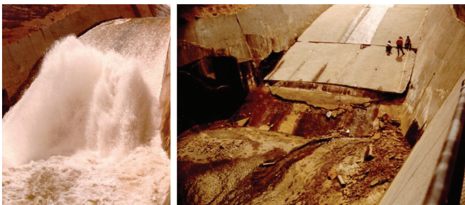
Figure 1. Hydraulic jacking failure at the Bureau of Reclamation's Big Sandy Dam (Wyoming, USA) in 1983.
