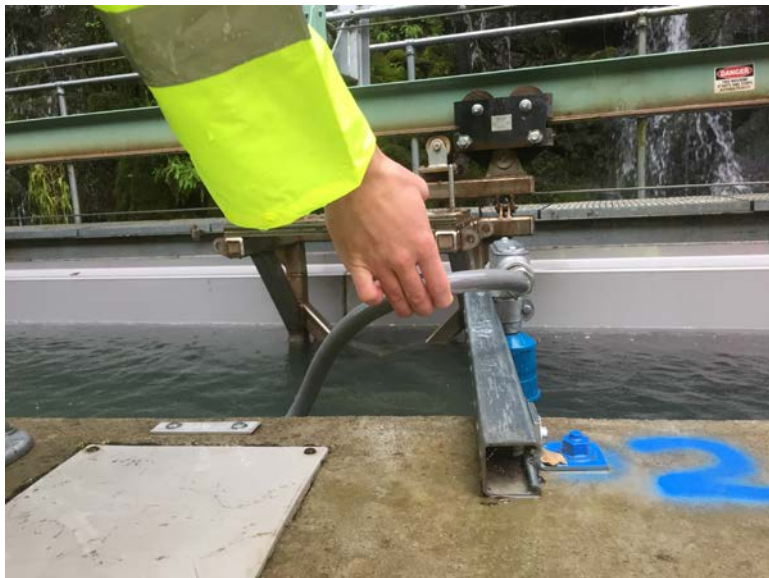
Figure 9. Fish screen forebay WSE (SS2) sensor and mounting bracket showing fish screen blanking panel in the distance. The enclosure for the wiring connections is mounted within the concrete wall to the left of the sensor mount
