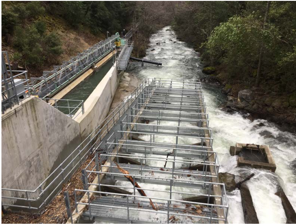
Figure 15. Photograph of North Battle Creek Feeder Diversion Dam fish screen and ladder from the access bridge above the dam. The concrete structure on the right side of the photo is an abandoned fish ladder.
