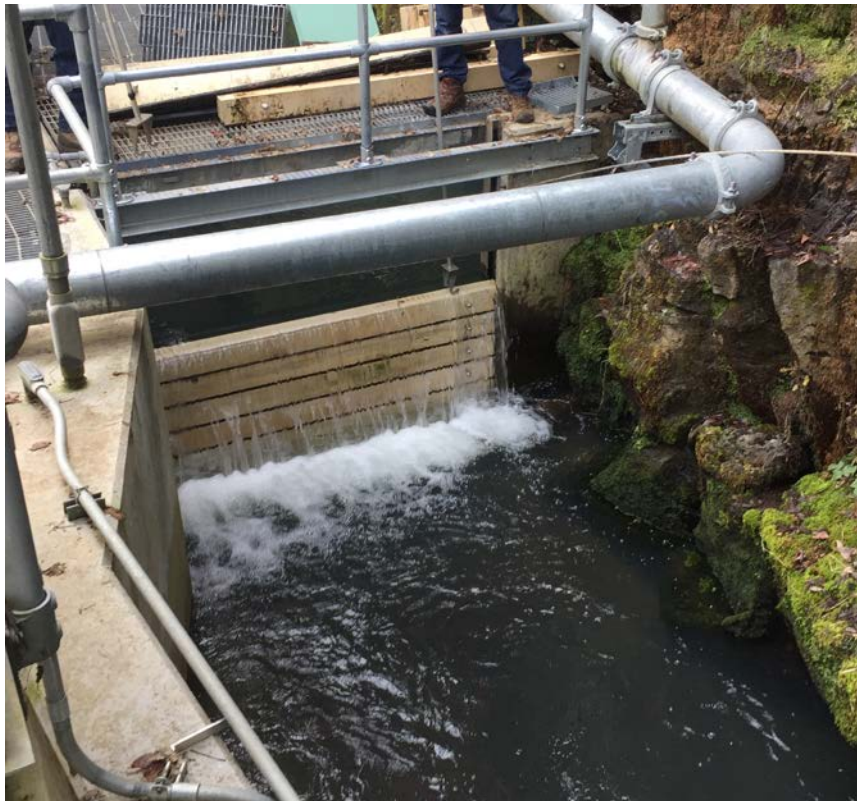
Figure 13. Photograph of the Eagle Canyon canal stoplog guides. Flows were measured at this location with a FlowTracker 2D ADV. Flow measurements were taken without stoplogs in the slot to compare to the CB43 discharge rating..
