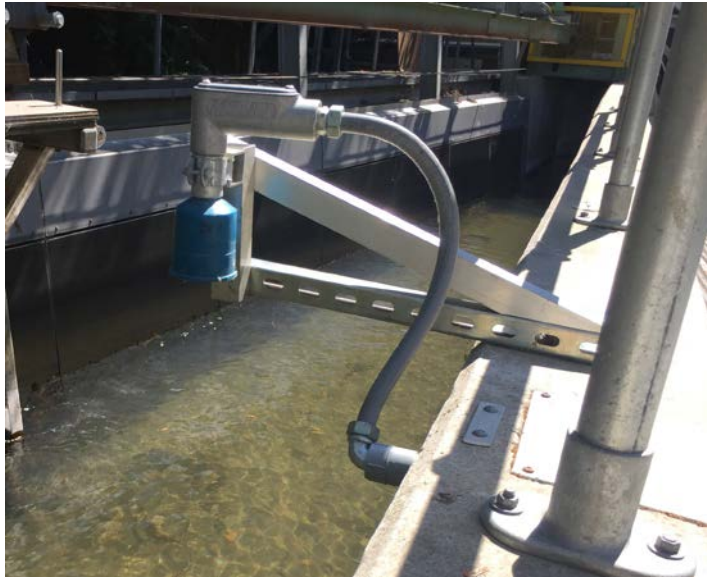
Figure 10. Fish screen forebay WSE (SS2) sensor and mounting bracket as modified in July 2019. The revised mount raised the sensor by 6.5 inches
