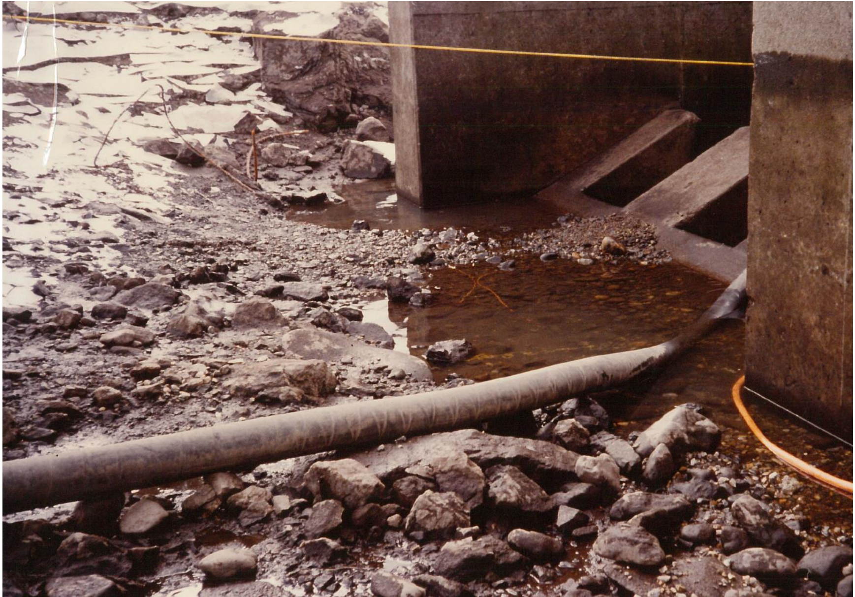
Figure 3. — Gravel deposit on the end sill of the outlet works stilling basin.
