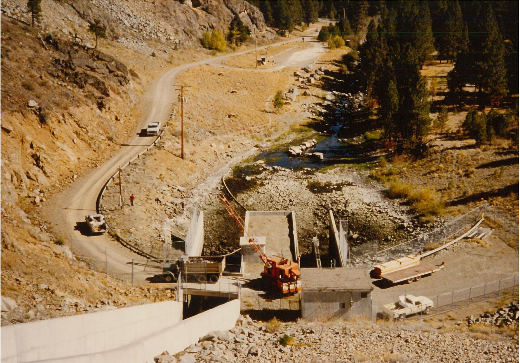
Figure 1. — Stilling basins at Mason Dam, Oregon. The spillway stilling basin is on the left, and the outlet works stilling basin is on the right.
