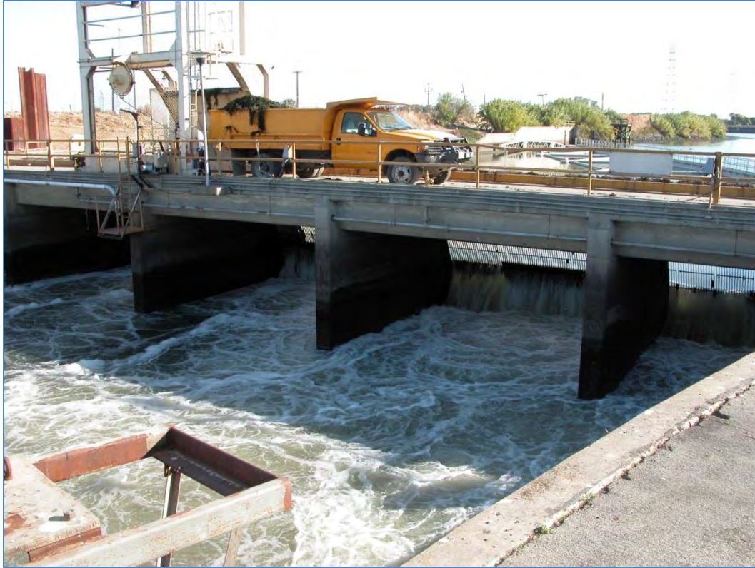
Figure A6-1.—Downstream looking perspective of the trashrack at the Bureau of Reclamation's Tracy Fish Collection Facility (Byron, CA). The image shows a significant trashrack differential, or difference in water depth upstream and downstream of the trashrack, and how such conditions create turbulent flows in the primary channel.
