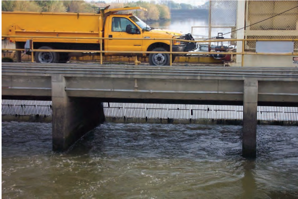
FIGURE 12.—Trashrack fouling was documented during data collection.
