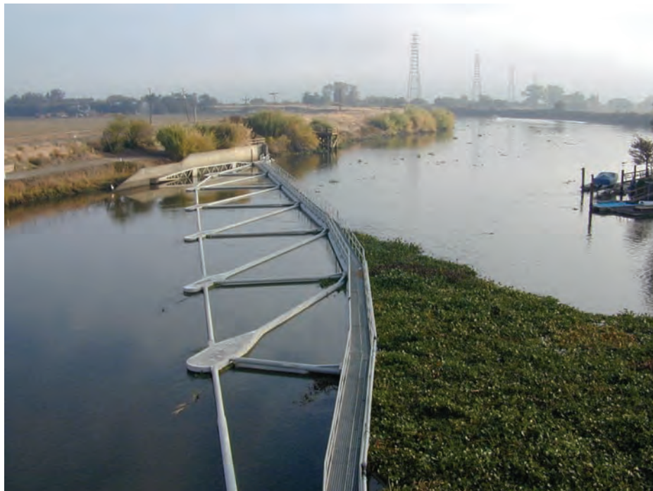
FIGURE 11.—Debris collected upstream from the debris boom. Heavy debris loads clog the facility and affect the performance of the louver system.
